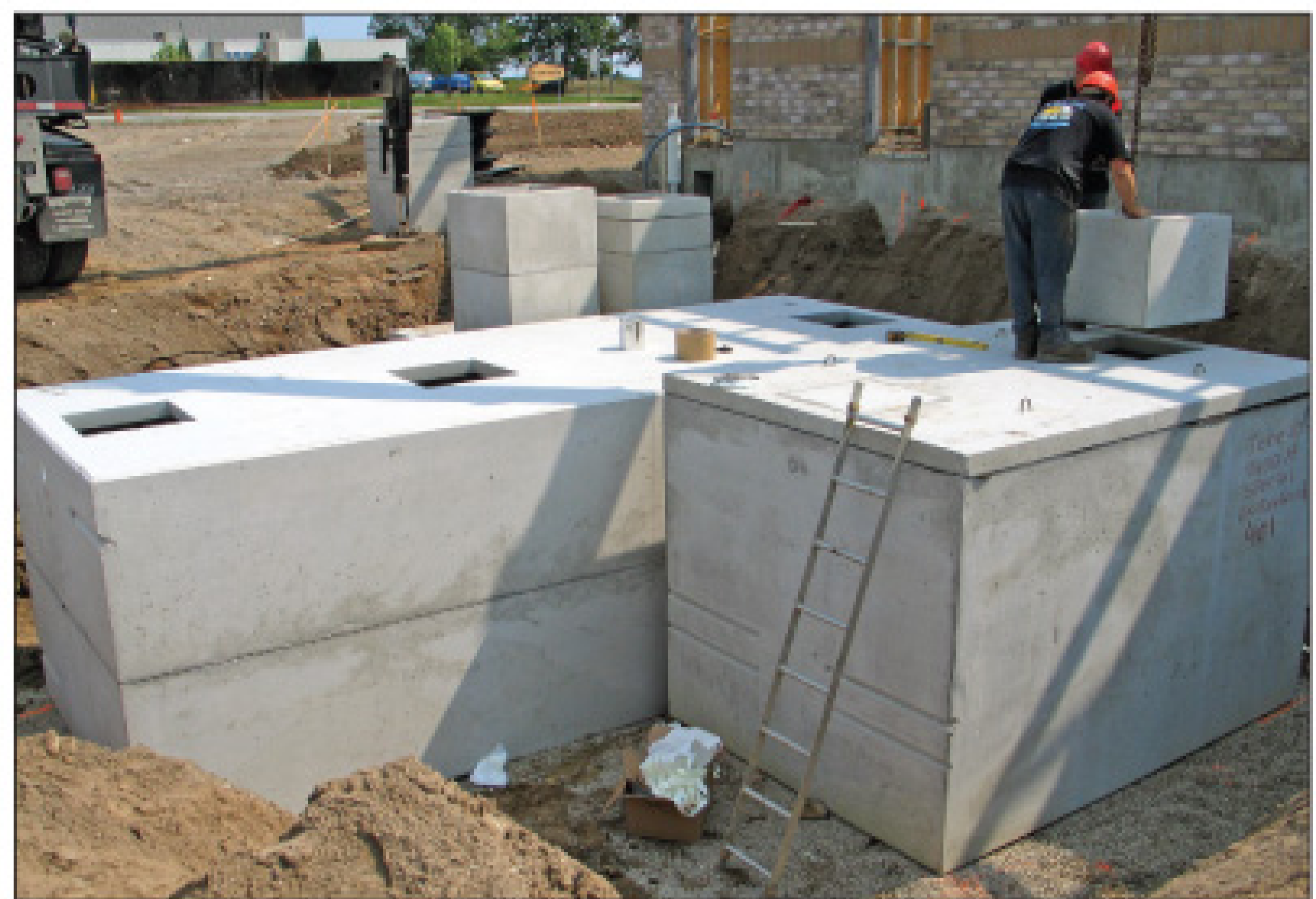
The crew from Unit Precast places (background to foreground) the kitchen holding tank, grease interceptor, and one pump tank.
