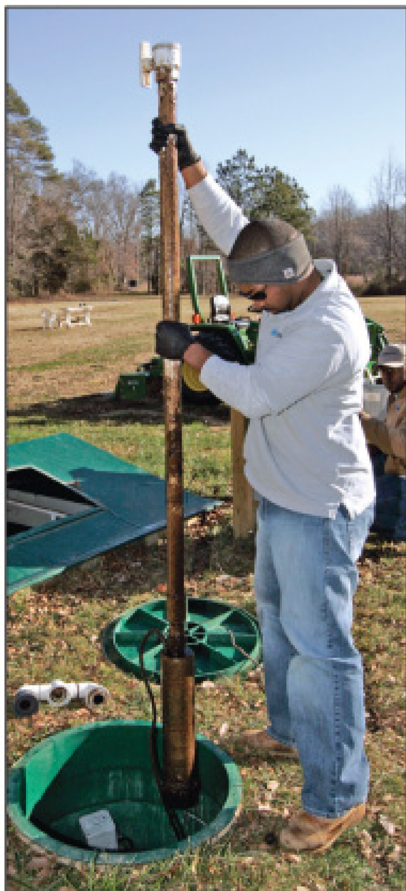
Jamal Jones pulls a pump from the second stage of a packed bed filter system.
