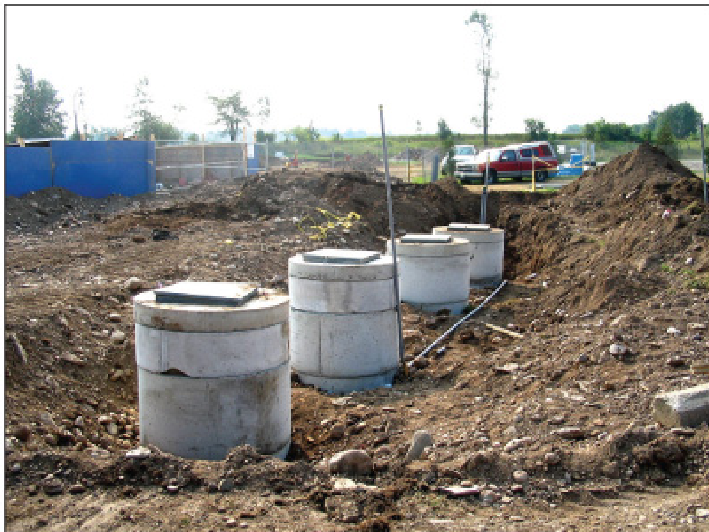
Access risers for deep-buried tanks are shown just after installation.
