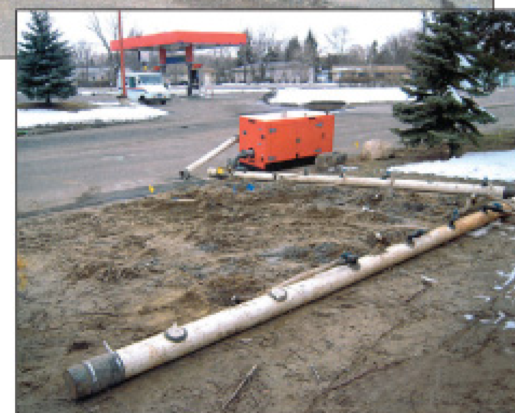
An example of a dewatering manifold fed by small-diameter well points.
