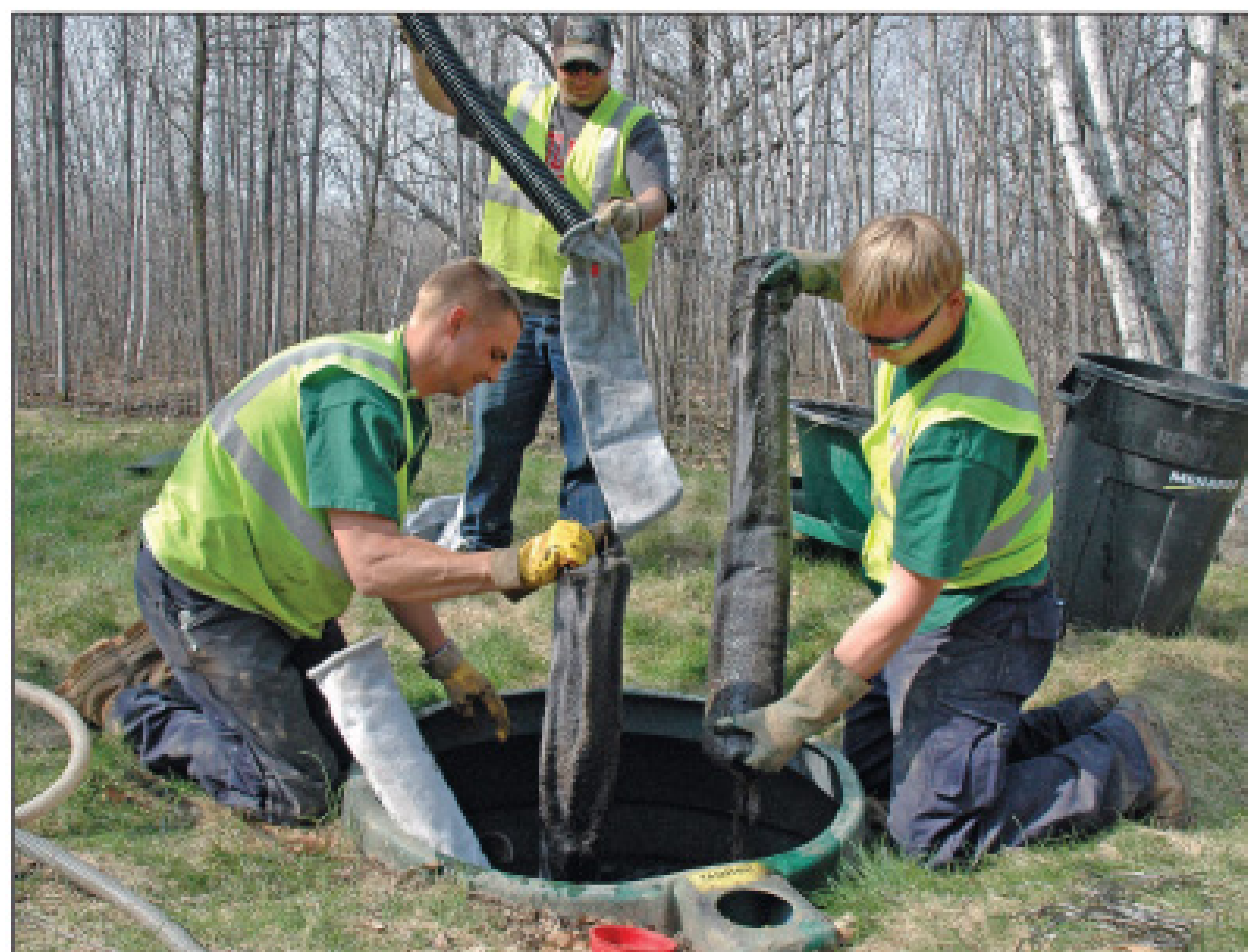
From left, Brian Koski, Kevin Newgard and Jared DeBoer replace the filter socks in a Multiflo aerobic treatment unit from Consolidated Treatment Systems Inc. Septic Check has a laundry that it uses to wash and reuse the socks, which are replaced about every five years.
