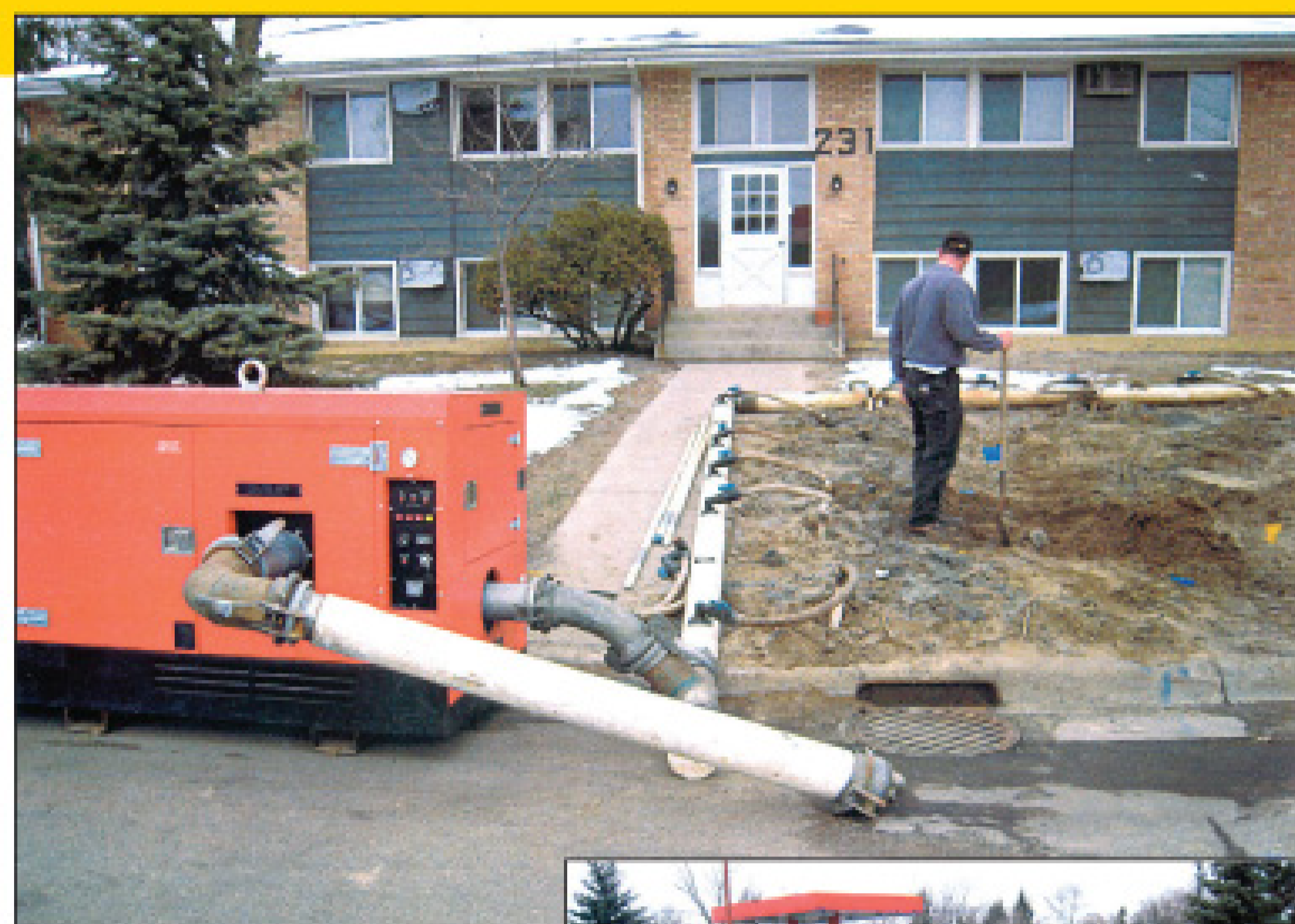
An example of a dewatering manifold fed by small-diameter well points.
