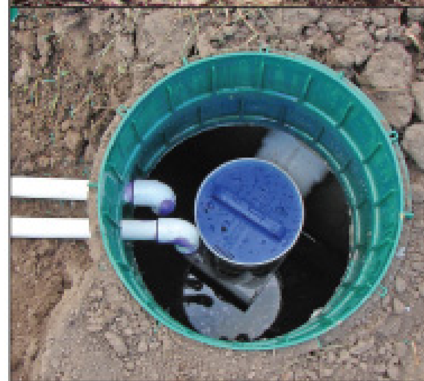
Tuf-Tite Inc. supplied the EF-6 Combo effluent filter.
