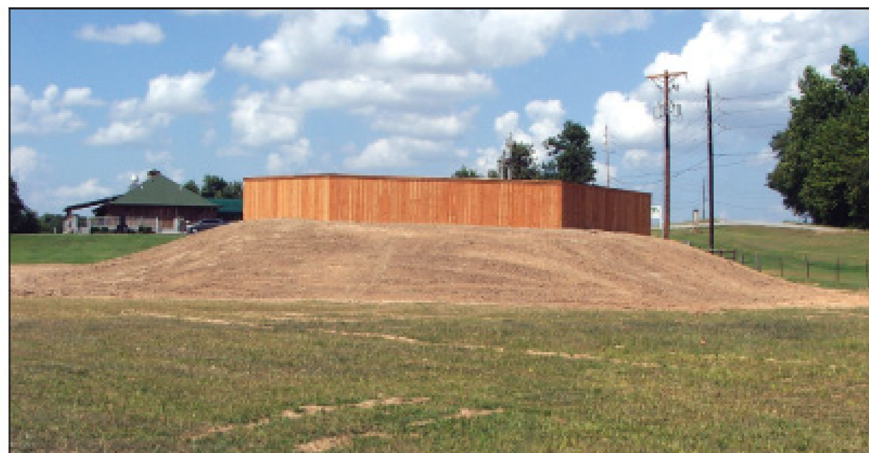
The completed treatment plant site, with Dripfield 1, zones 1-4, in the background.
