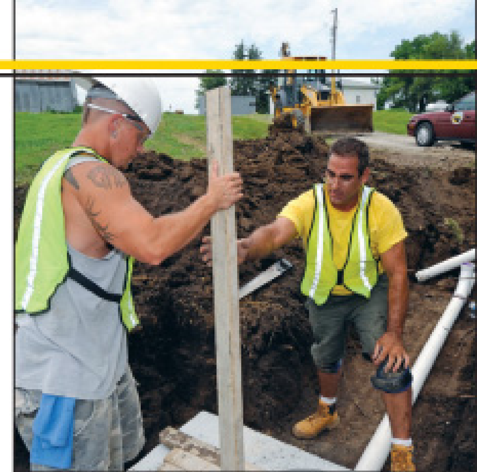
The Jakoubeks prepare a septic tank for installation.
