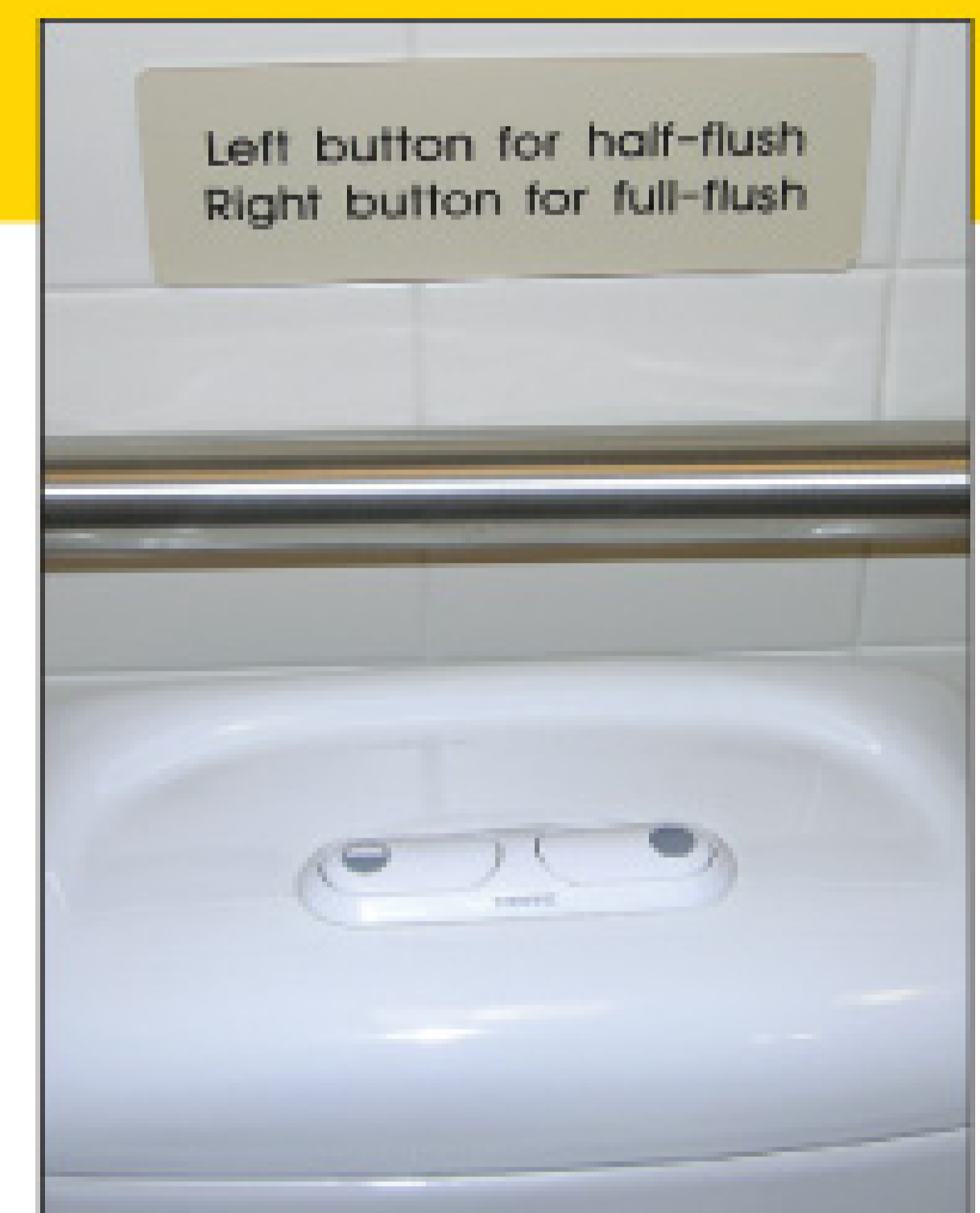
New techniques for saving water in homes with onsite systems include toilets that allow the owner to choose a half flush or a full flush.
