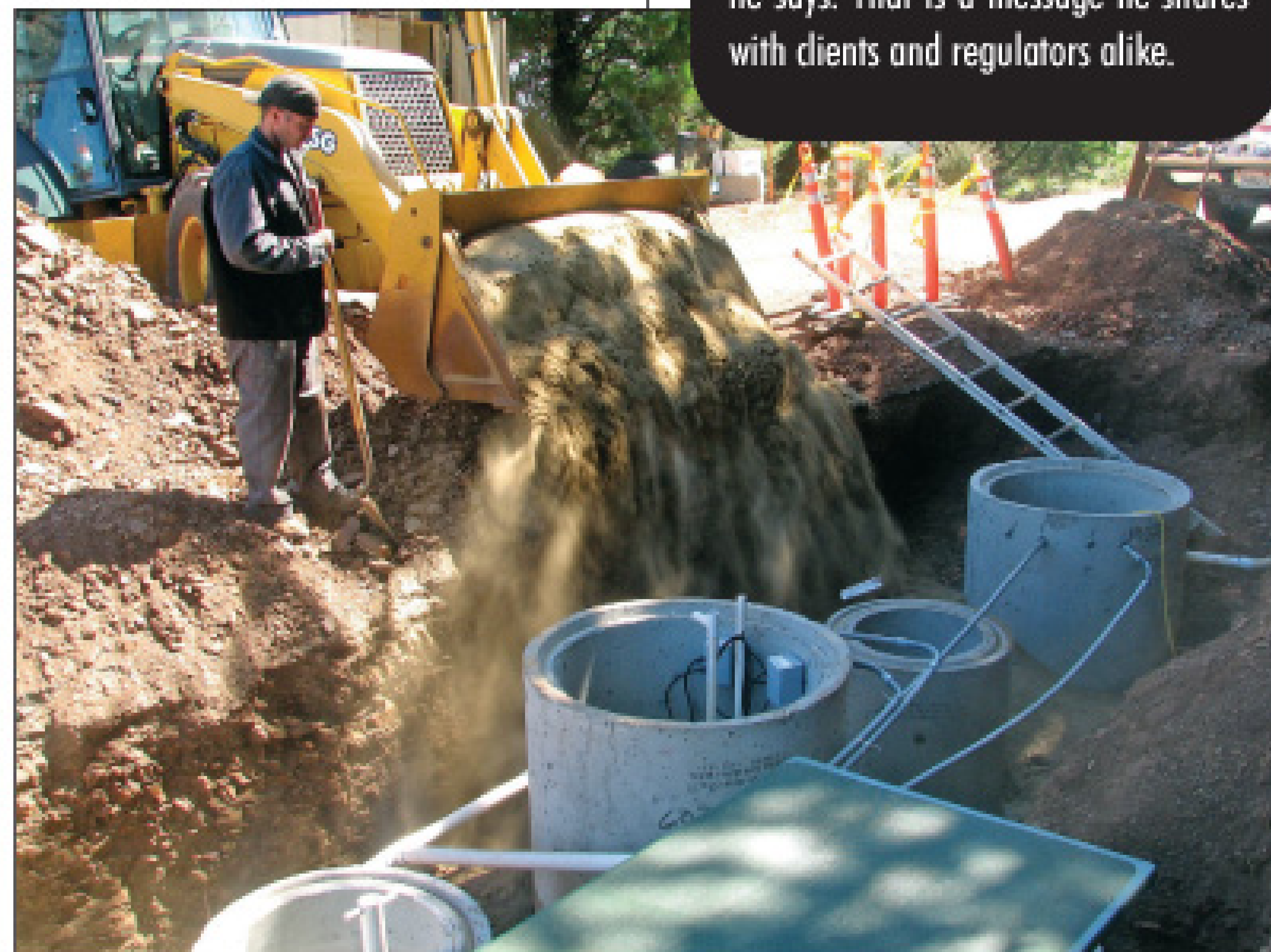
Damon Clark supervises backfilling of an AdvanTex aerobic treatment system. (Photo by Josh Clark)
