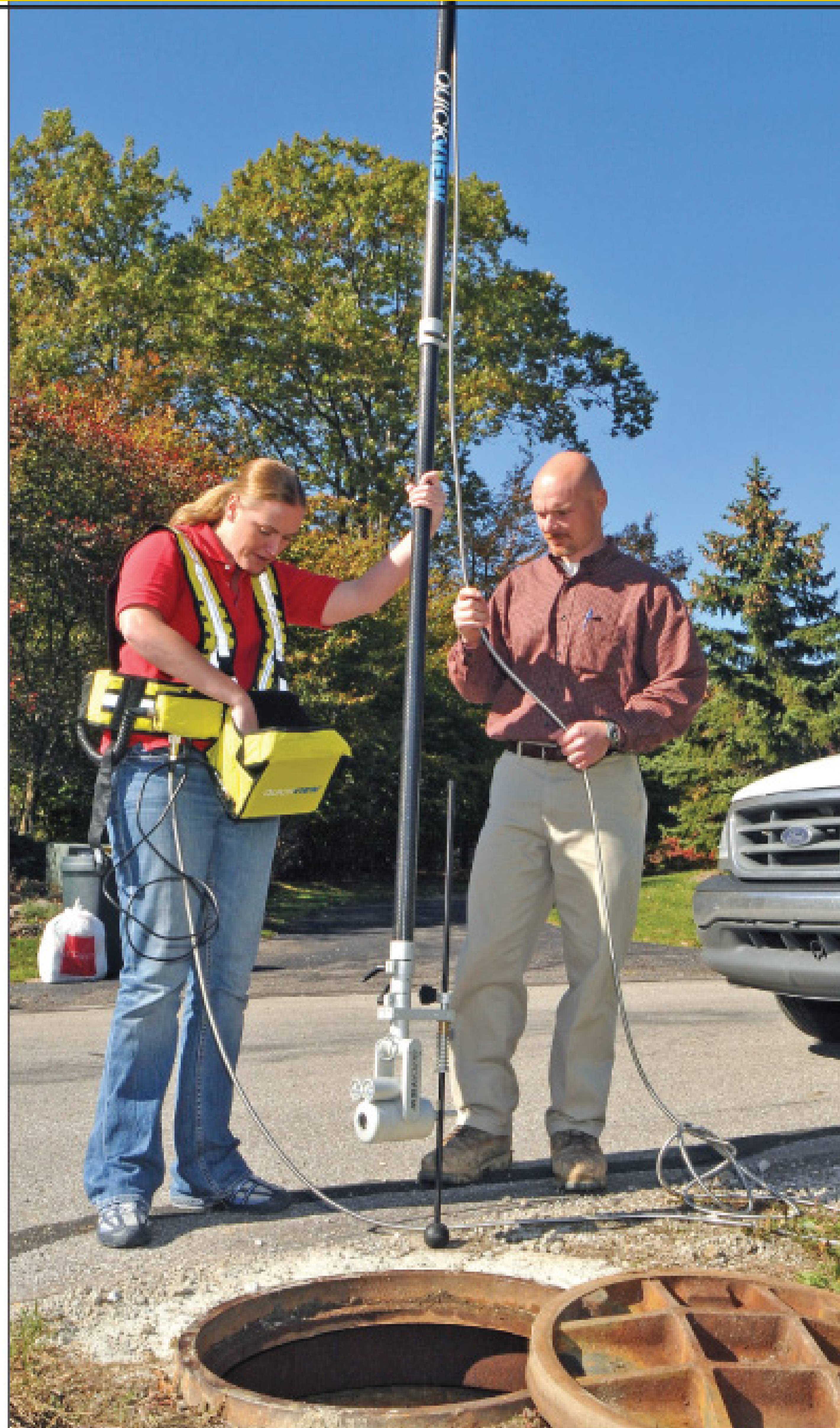
Laura Travers operates a QuickView zoom camera from Envirosight LLC with assistance from Nate McConoughey. The camera allows inspection of storm and sanitary sewers without confined-space entry.
