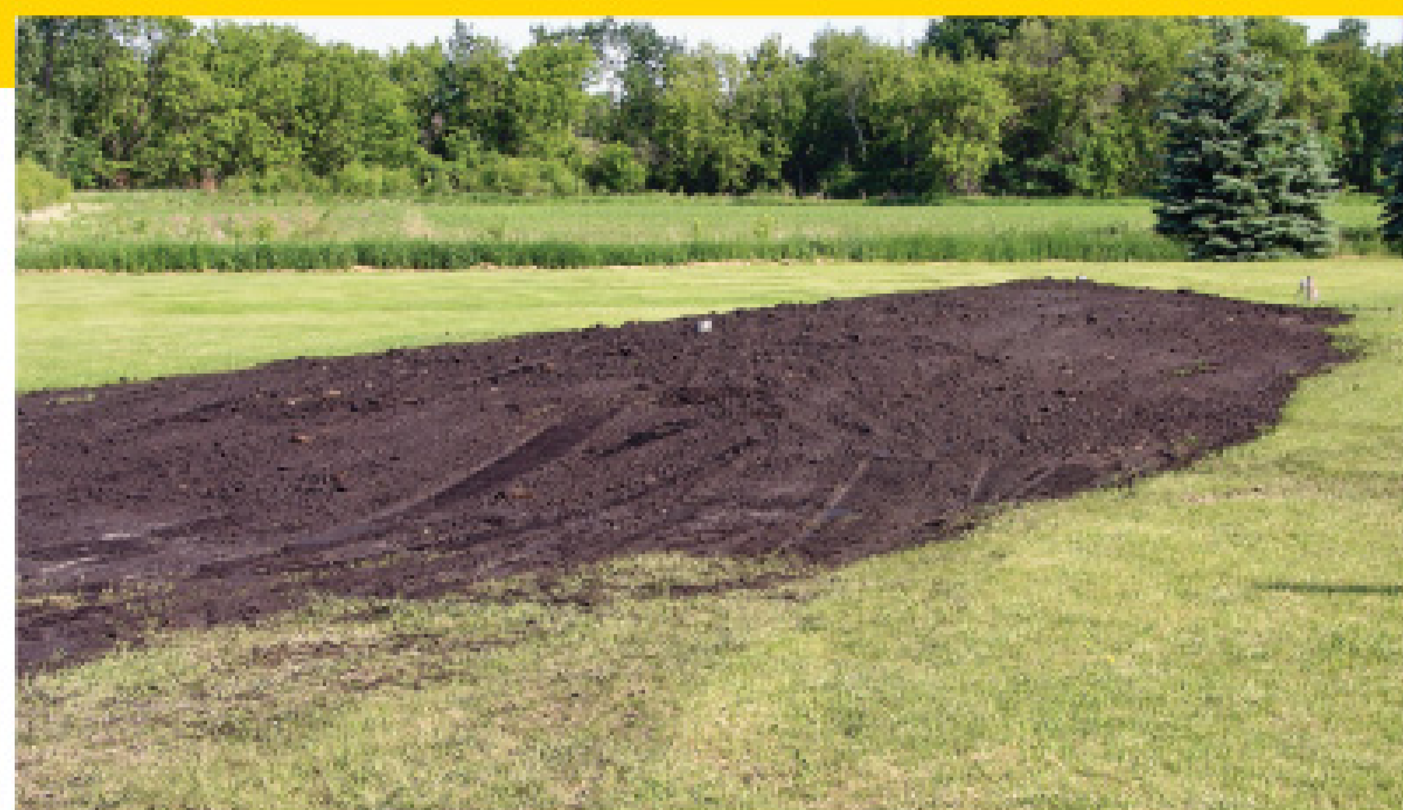
Here, a mound system has been covered with topsoil.
