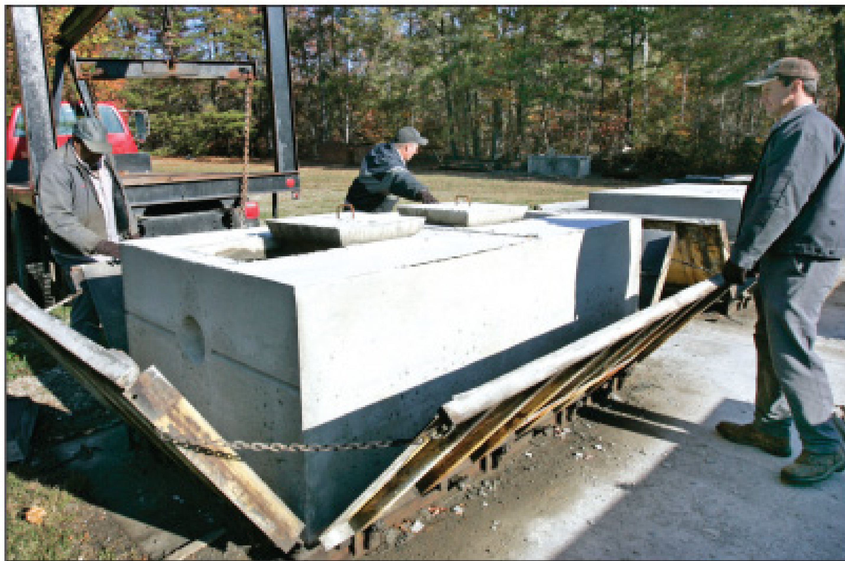
From left, Linwood Harris and co-owners Everett Parsley and Mike Parsley open a form to reveal one of the concrete septic tanks the company produces.
