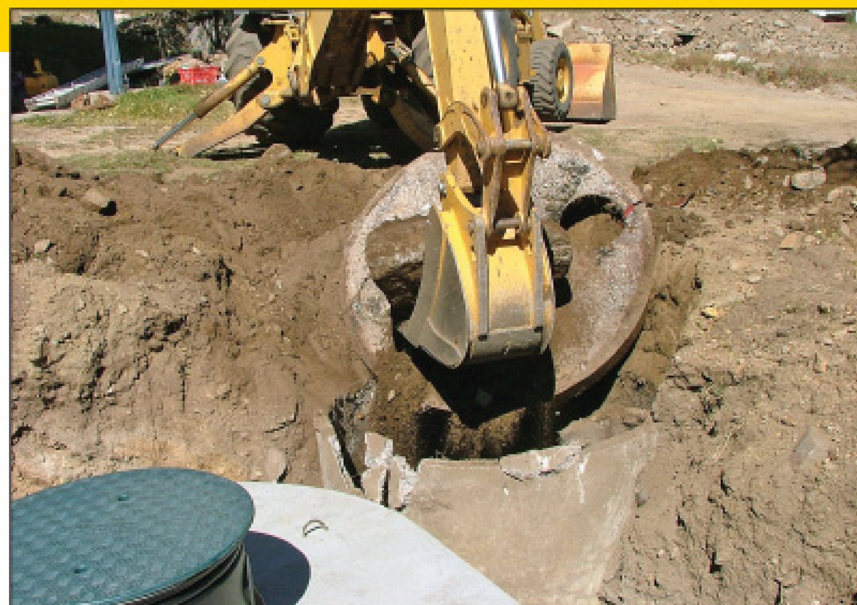
To abandon an old onsite system properly, the tank must be removed or filled with aggregate. (Photography by David Gustafson, P.E.)
