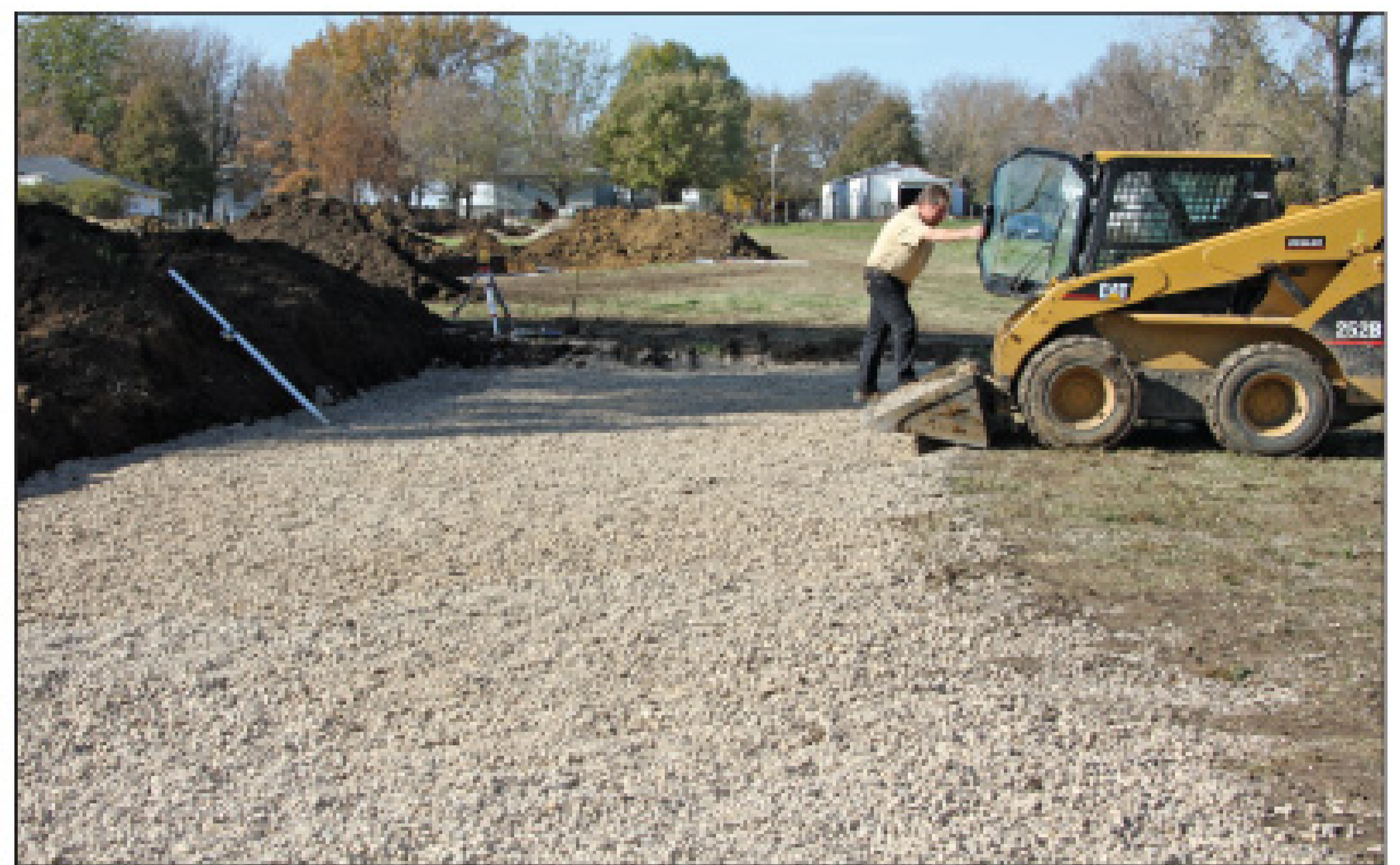
George Dickerson Sr. covers the dosing field with washed rock.
