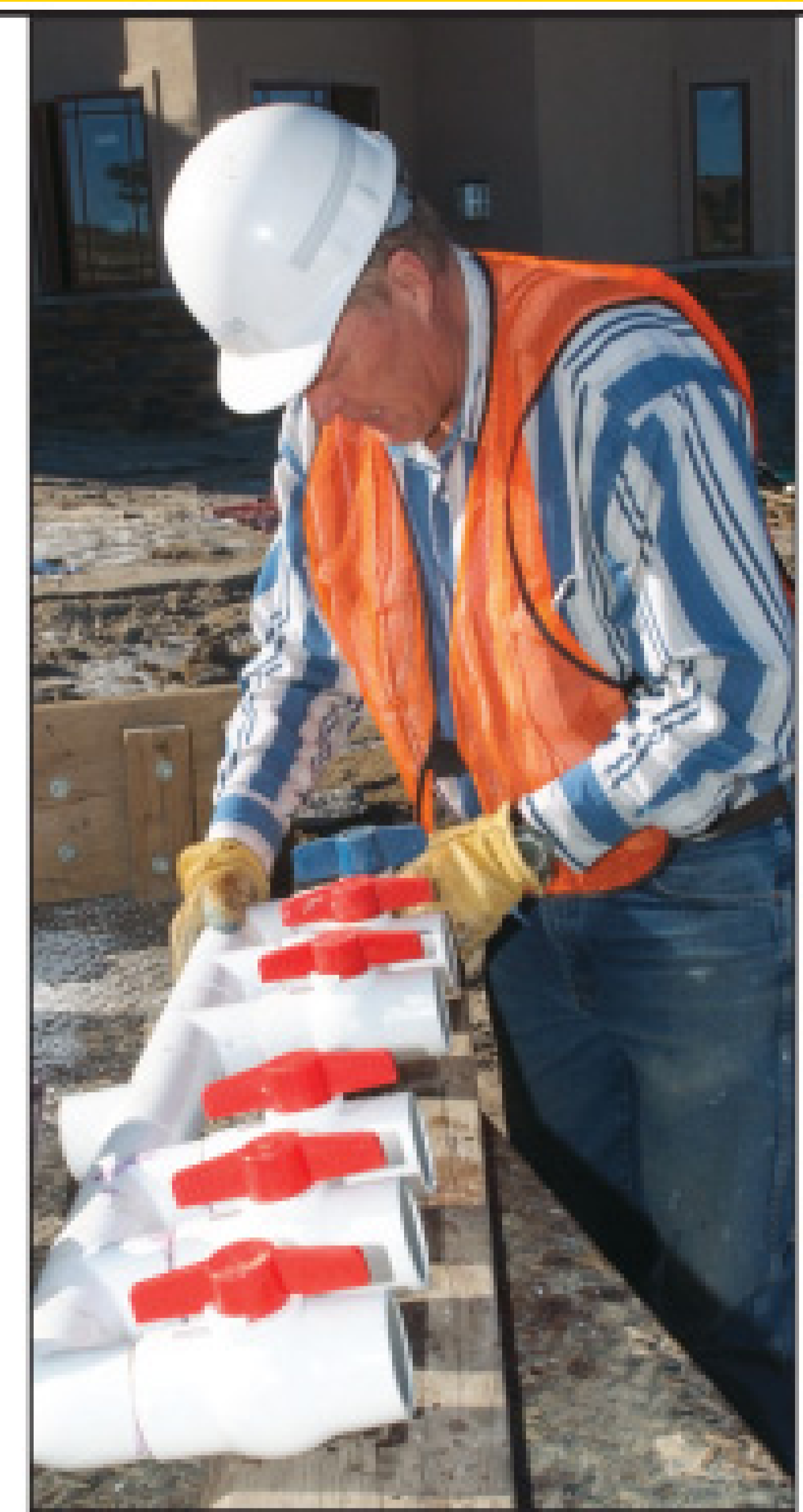
Mike Oliver prepares a drain manifold.
