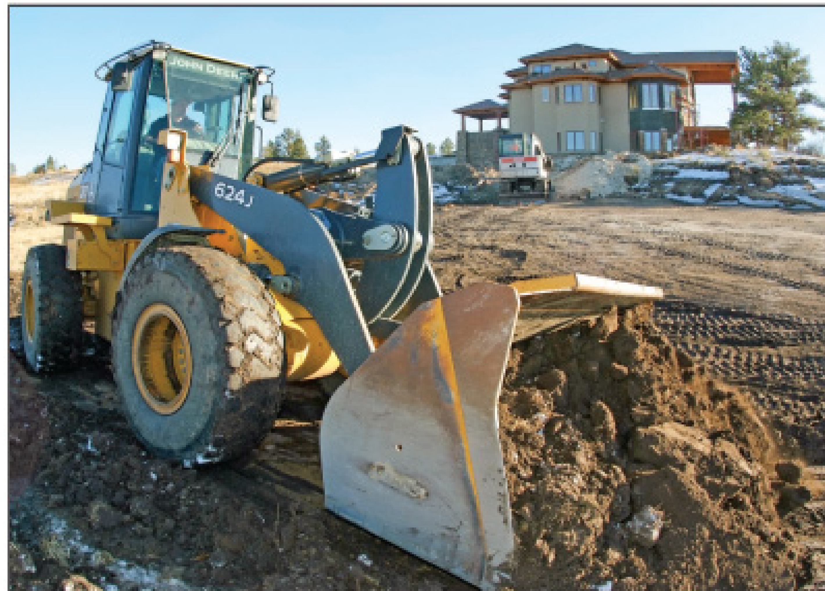
Scott Kellogg excavates a drainfield with a John Deere 624 front loader.
