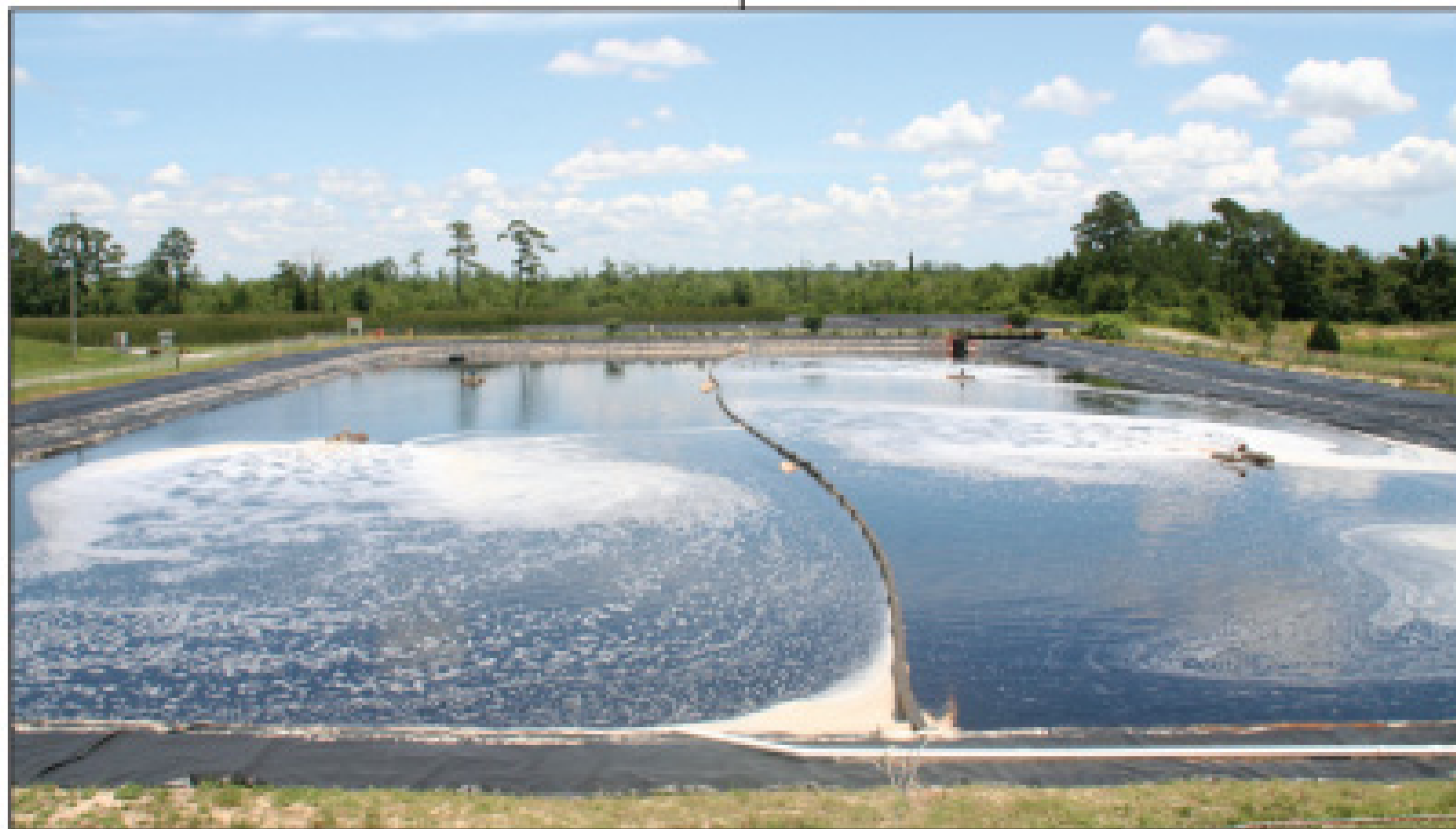
The lagoon, seen from the top of the wastewater treatment plant. What looks like a black box in the back left corner of the lagoon is the influent pump for the wetlands. (Photo by Shannon Culpepper)
