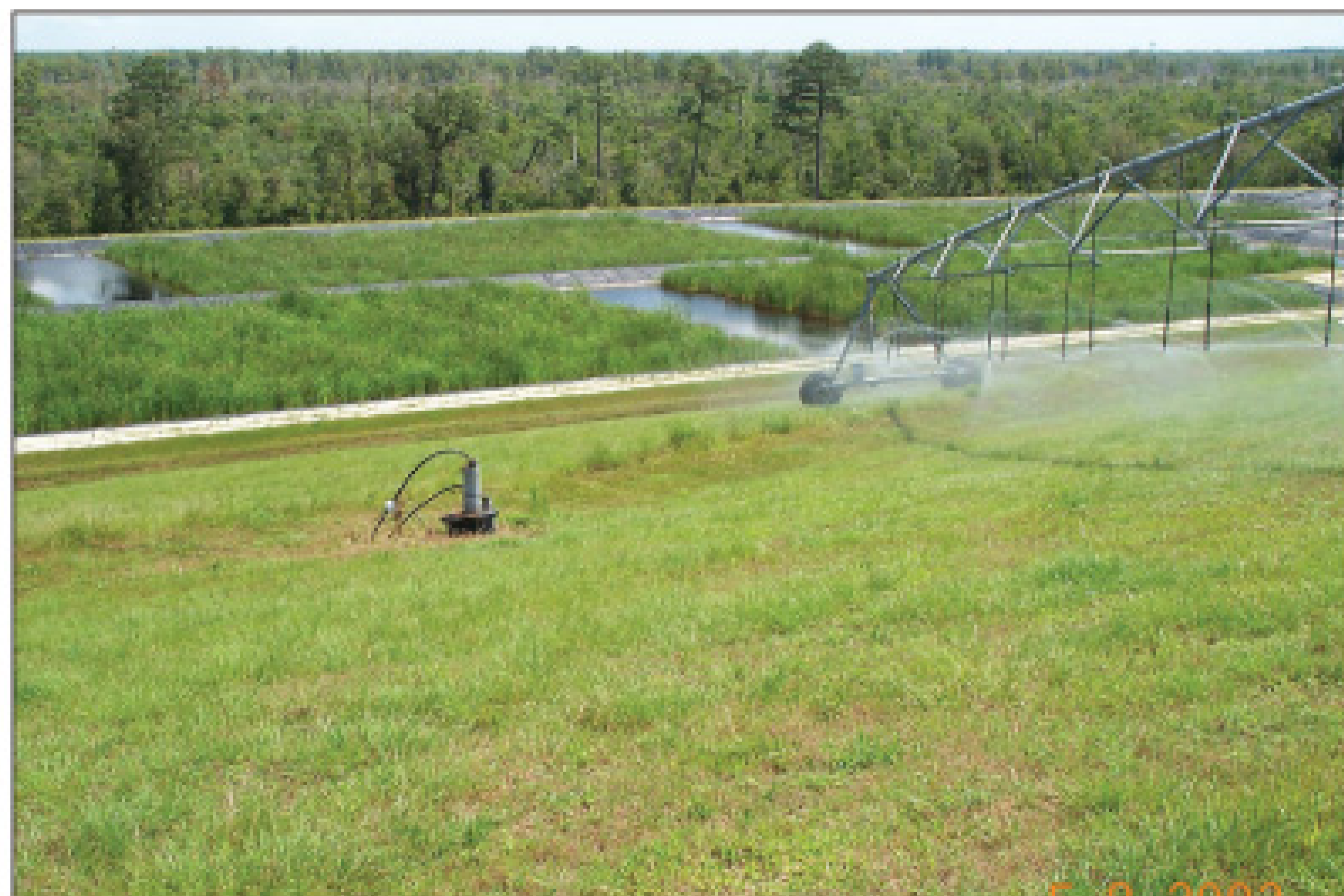
A Greenfield mini center-pivot irrigation system sprays 10,000 gallons an hour of treated landfill leachate on a 10-acre closed cell. Wetland Ponds A and B are in the background. (Photo courtesy of the New Hanover County Department of Environmental Management)
