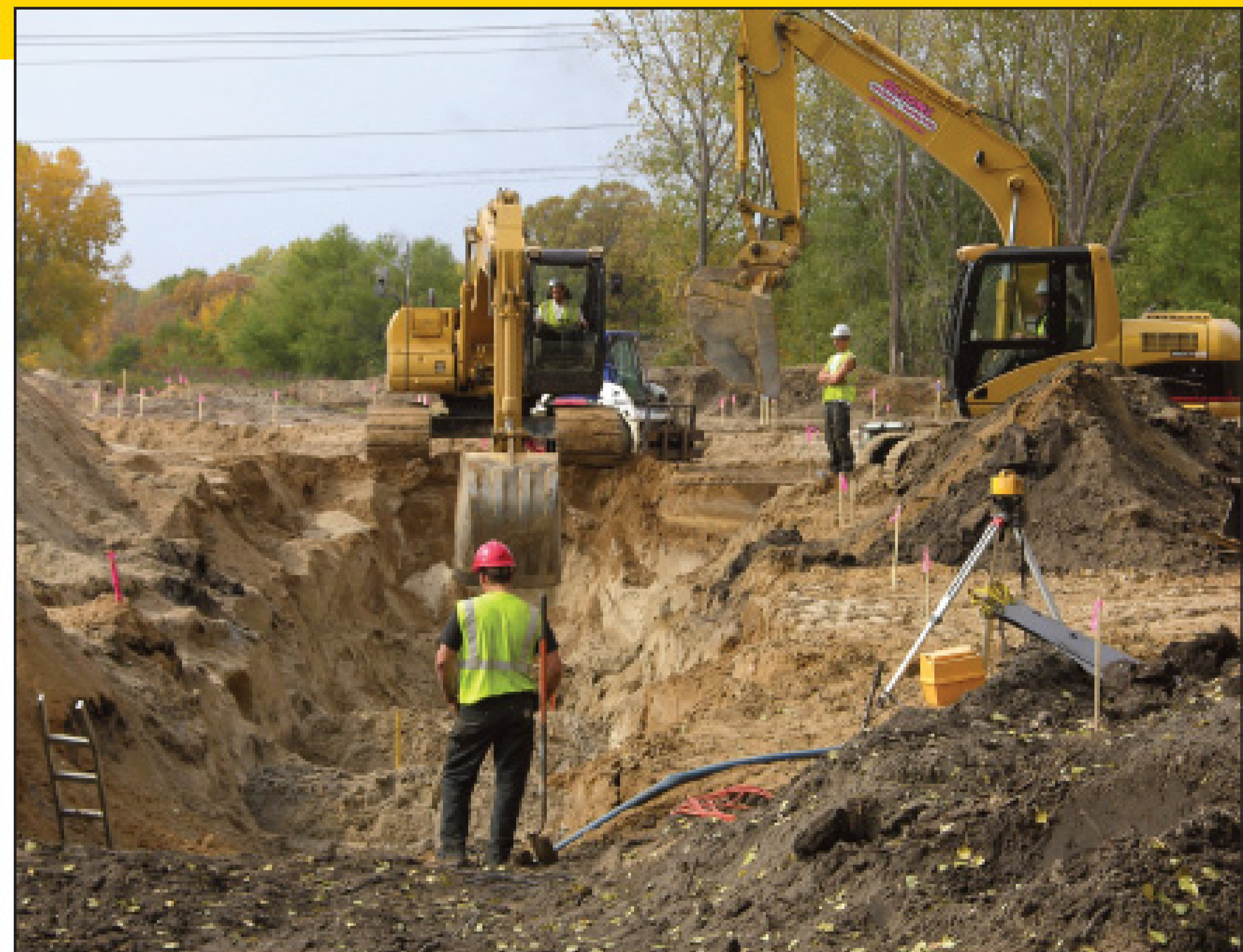
A laser level and a shovel represent the high and low ends of valuable tools for installers. (Photos courtesy of Jim Anderson and Dave Gustafson)
