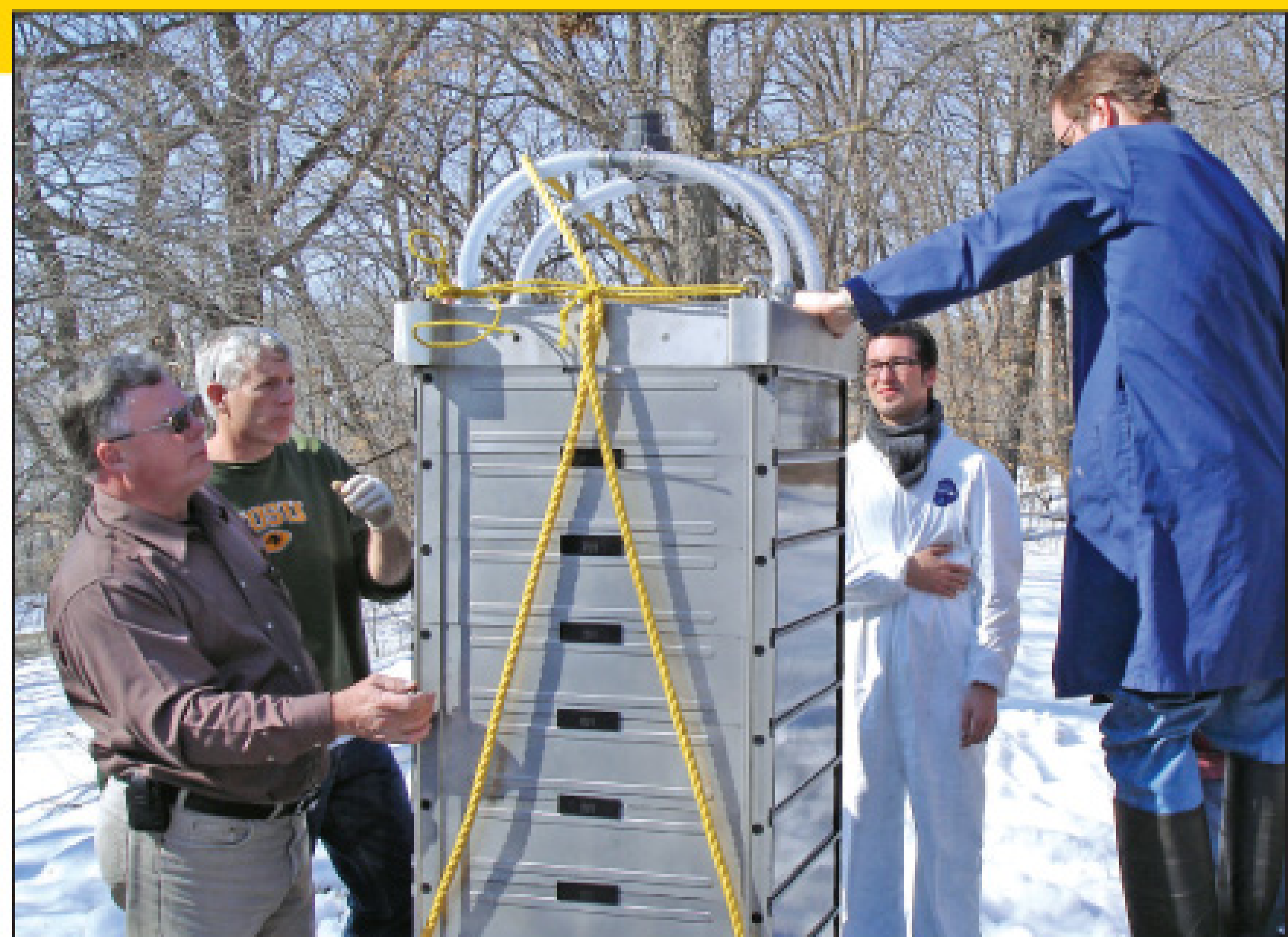
Ed Gades of Ivanhoe Environmental, Jim Lockrem of SJE-Rhombus, Christof Gränitz of ItN Nanovation, and Dave Long of SJE-Rhombus prepare the 600-pound ceramic membrane tower for its descent into the filtration tank. (Photos courtesy of SJE-Rhombus Controls)
