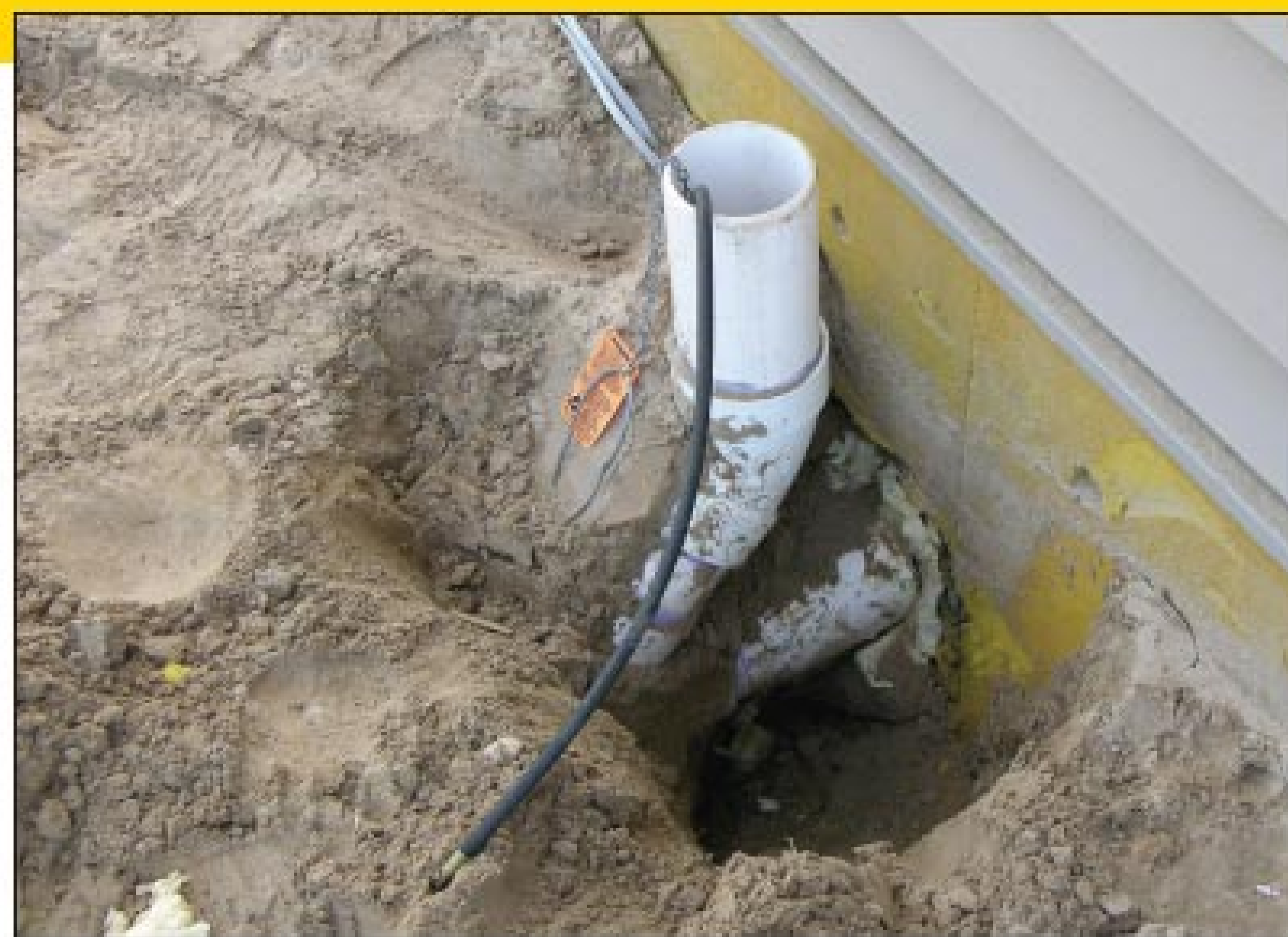
A cleanout installed outside the house on the building sewer makes it easier to jet the line from outside the house. Cleanouts should extend at least 2 inches above grade.
