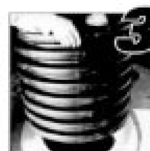
Place plastic maintenance pipe on ring.
