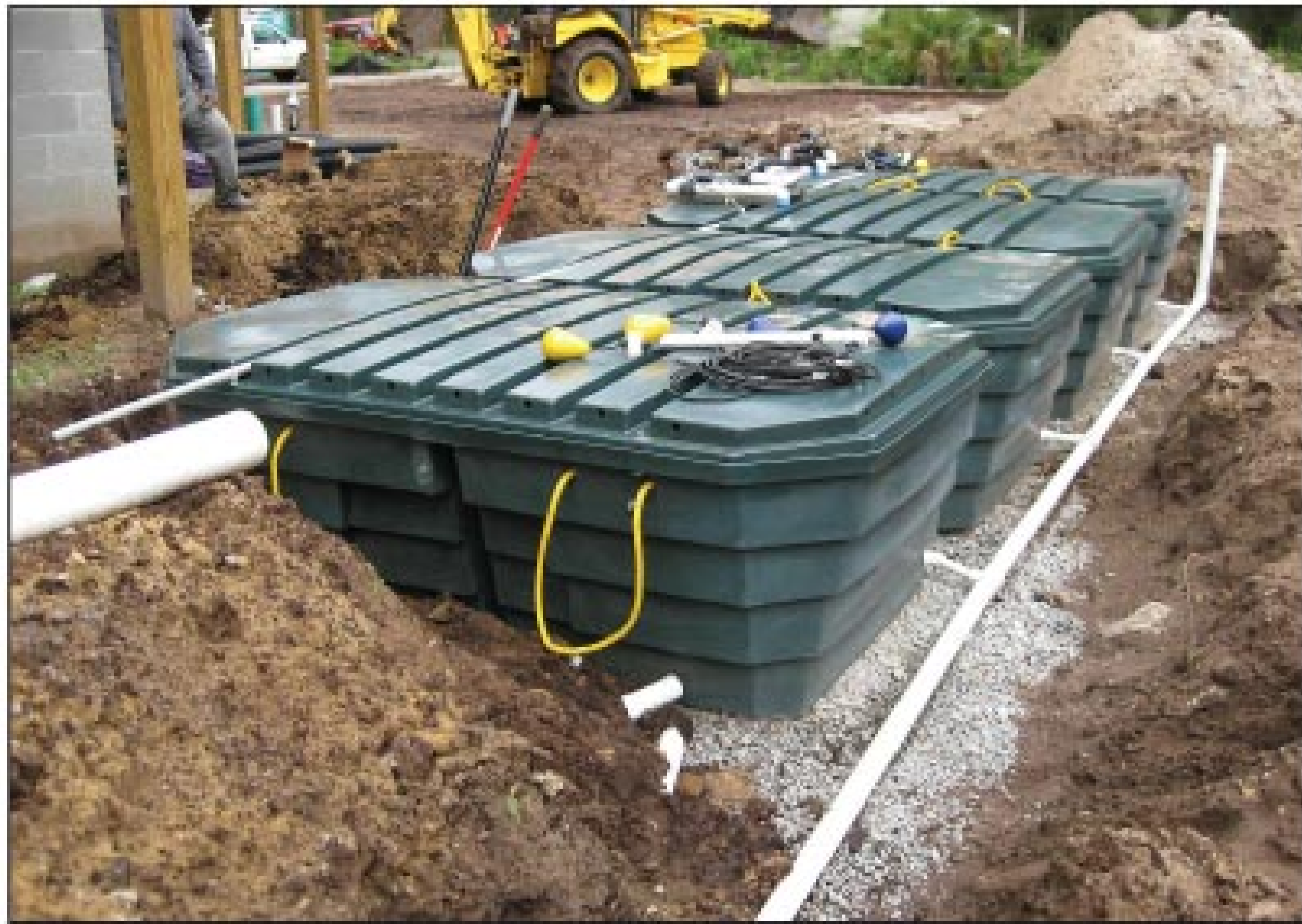
The four biofilter modules rest on a 6-inch-deep gravel support bed.
