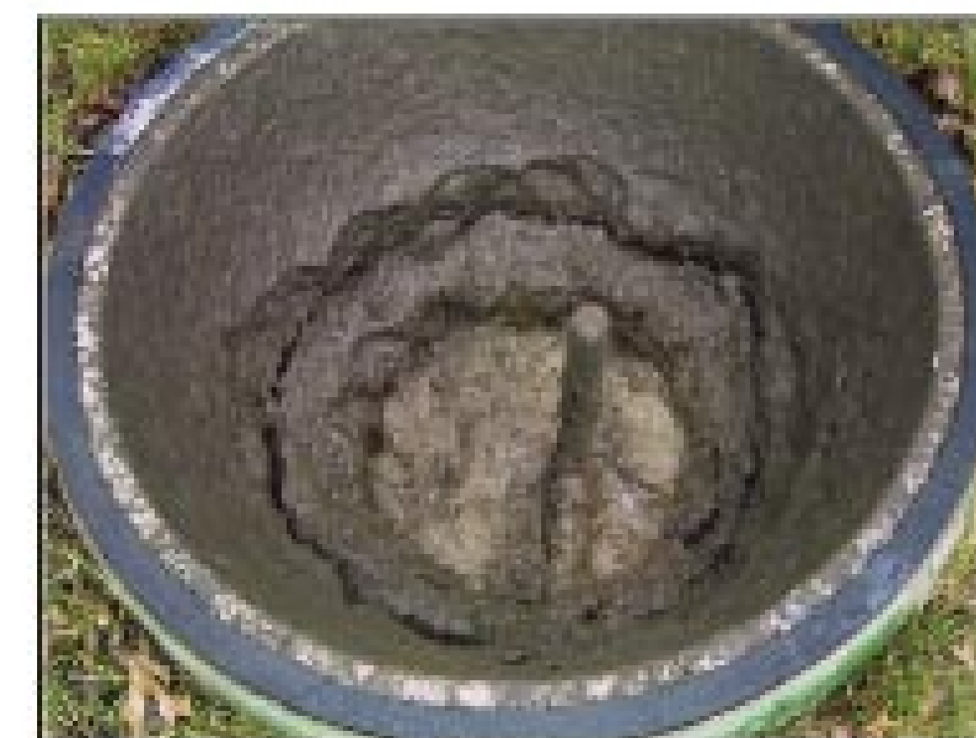
Light, fluffy scum caused by bulking sludge.
