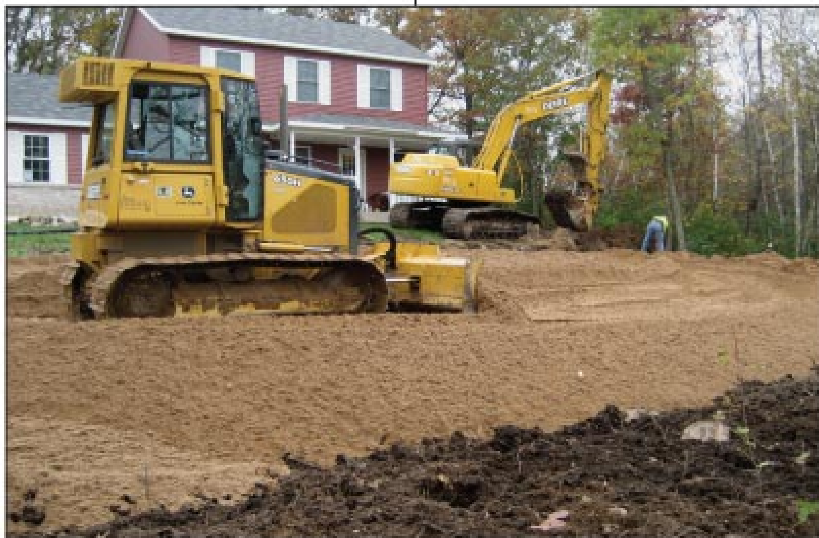
The clean sand for a mound is placed over the properly scarified soil surface.
