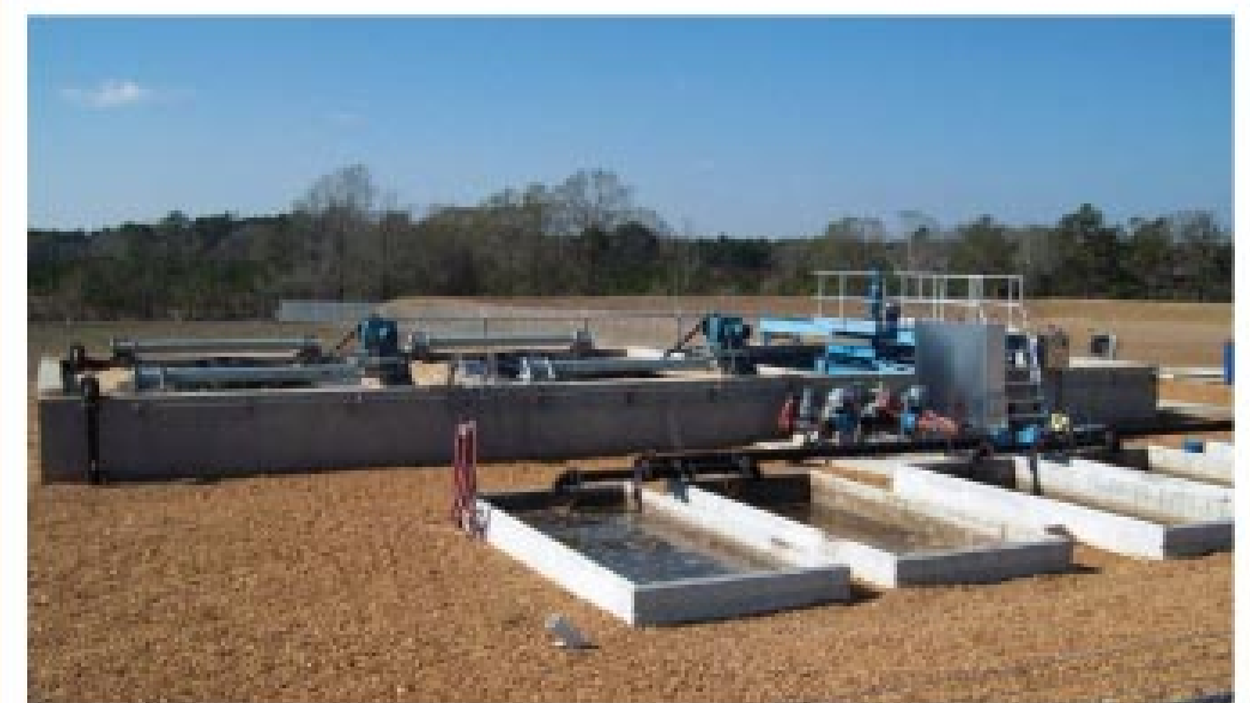
250,000 GPD (500,000 peak) system for a small city.
