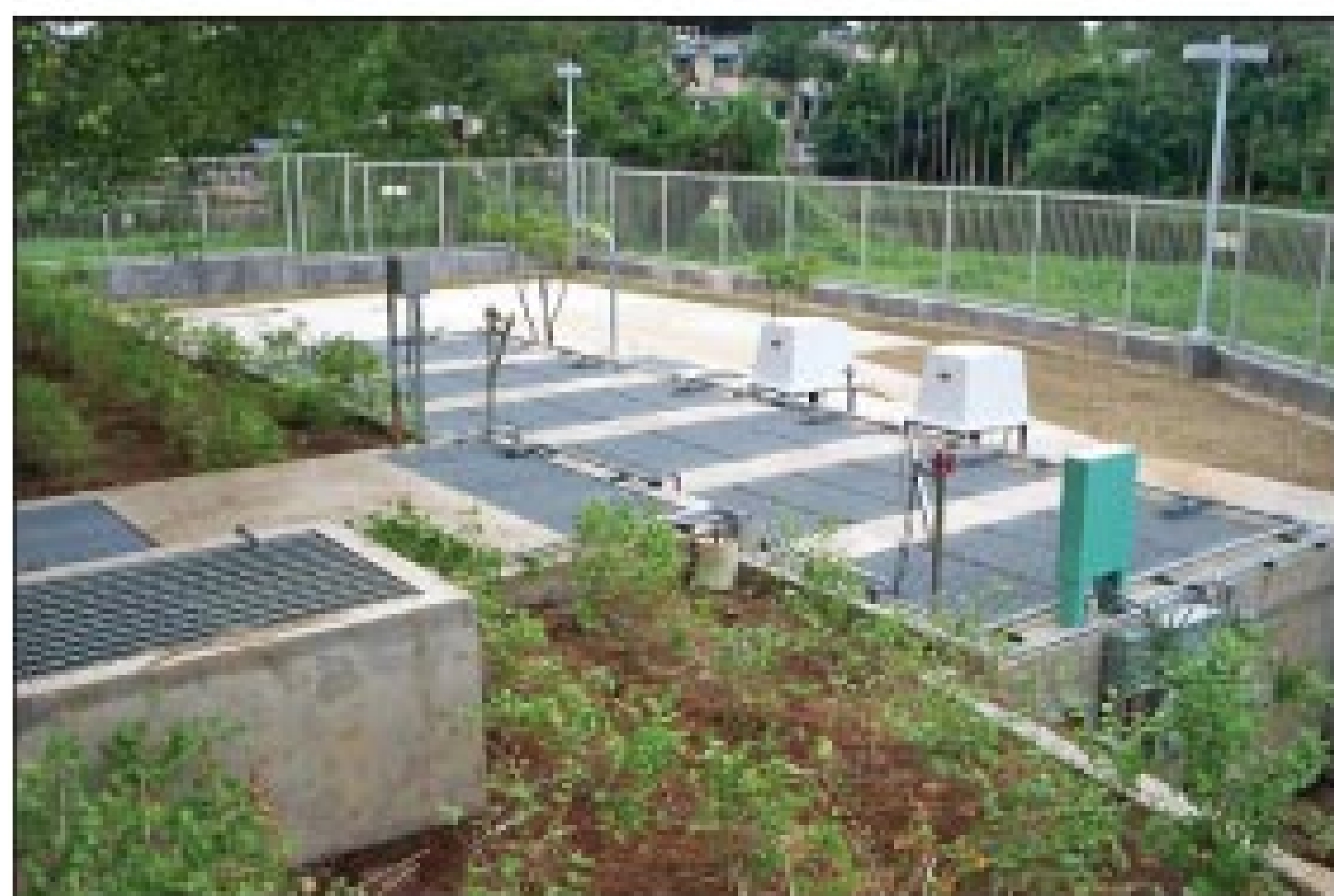
Module construction from Jet Inc.
