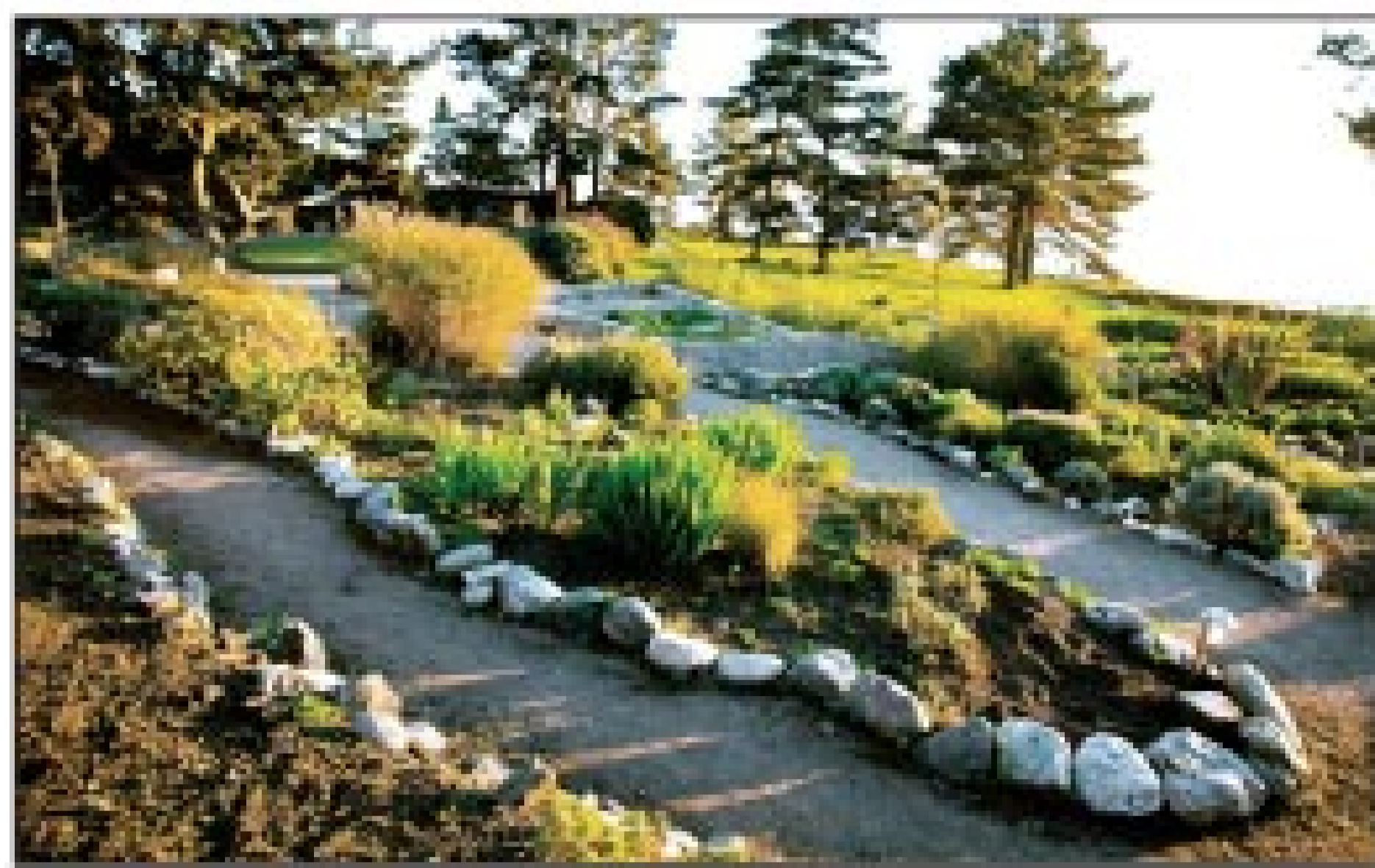
NextGen Living Machine from Worrell Water Technologies LLC
