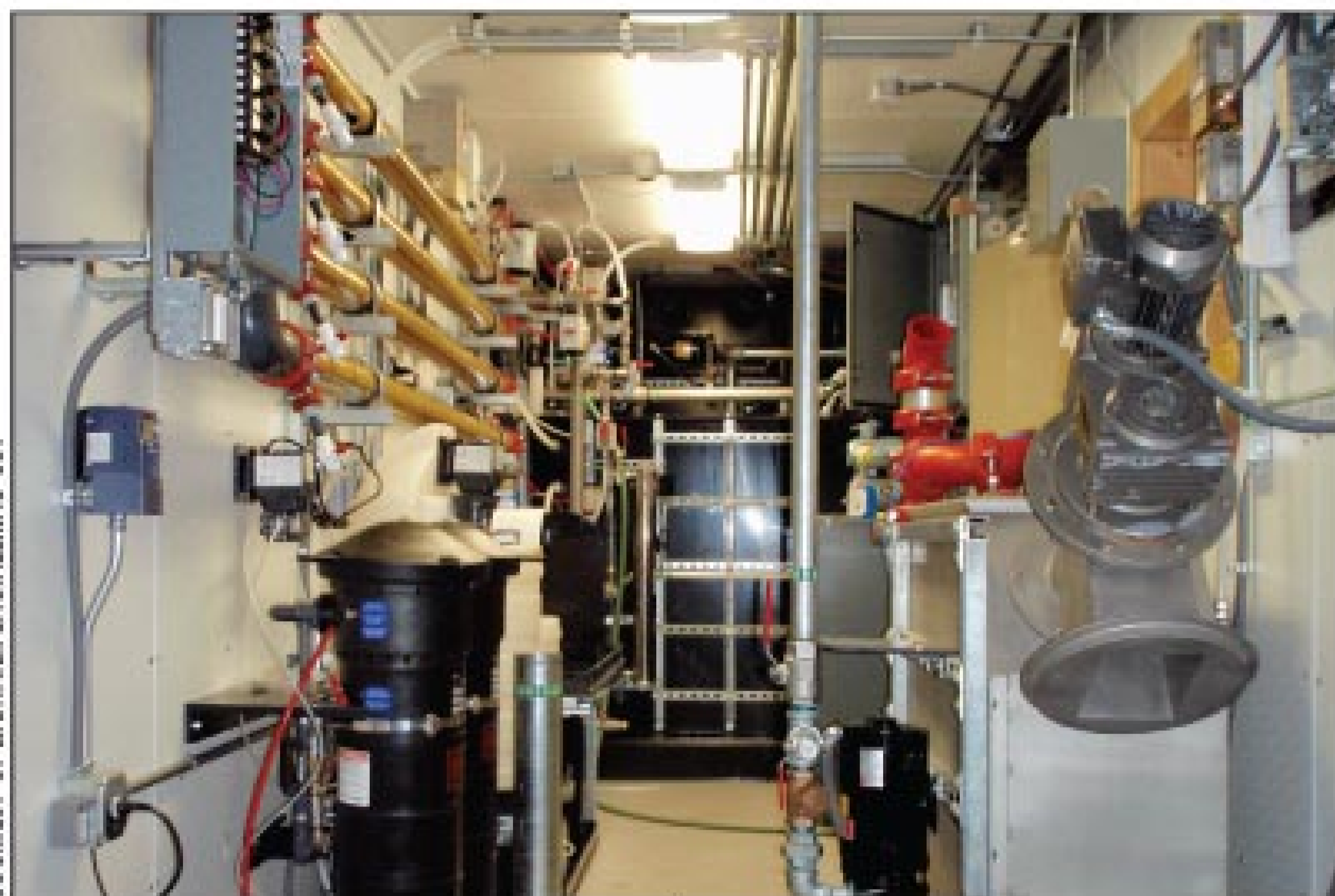
Above: The Sherman Adams Building is 75 feet above the treatment plant and 400 feet away. An arctic entrance has since been added to the plant. Left: The equipment room nears completion. The long, brown pipes are the tubular membranes. The Trojan UV disinfection system is mounted to the end of the lower tank. The control panel and operator's desk are on the right side, and the raw sewage screen is in the foreground.
