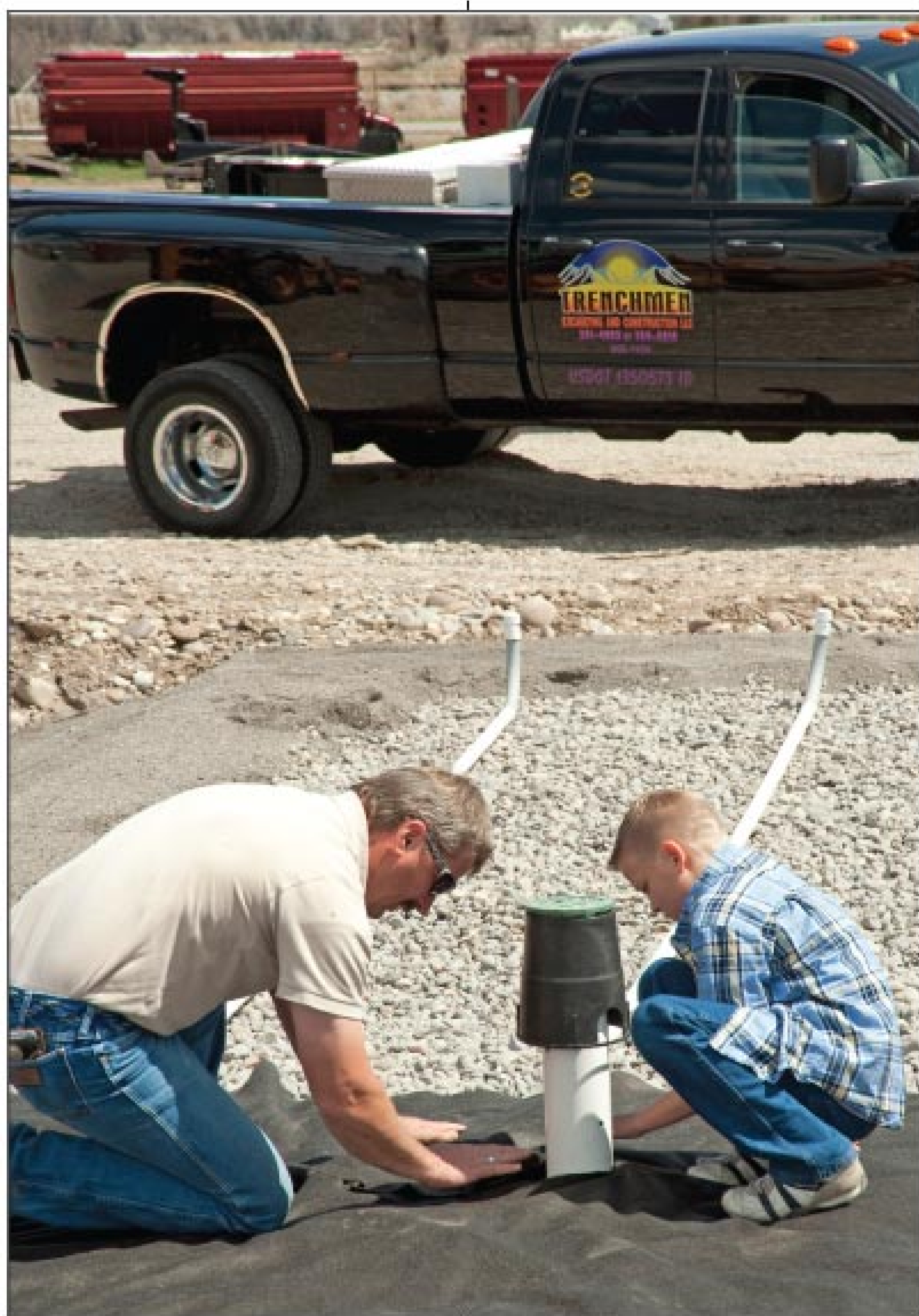
Kim Walker and son Trey place geotextile cloth over the gravel bed on a pressurized sand mound.
