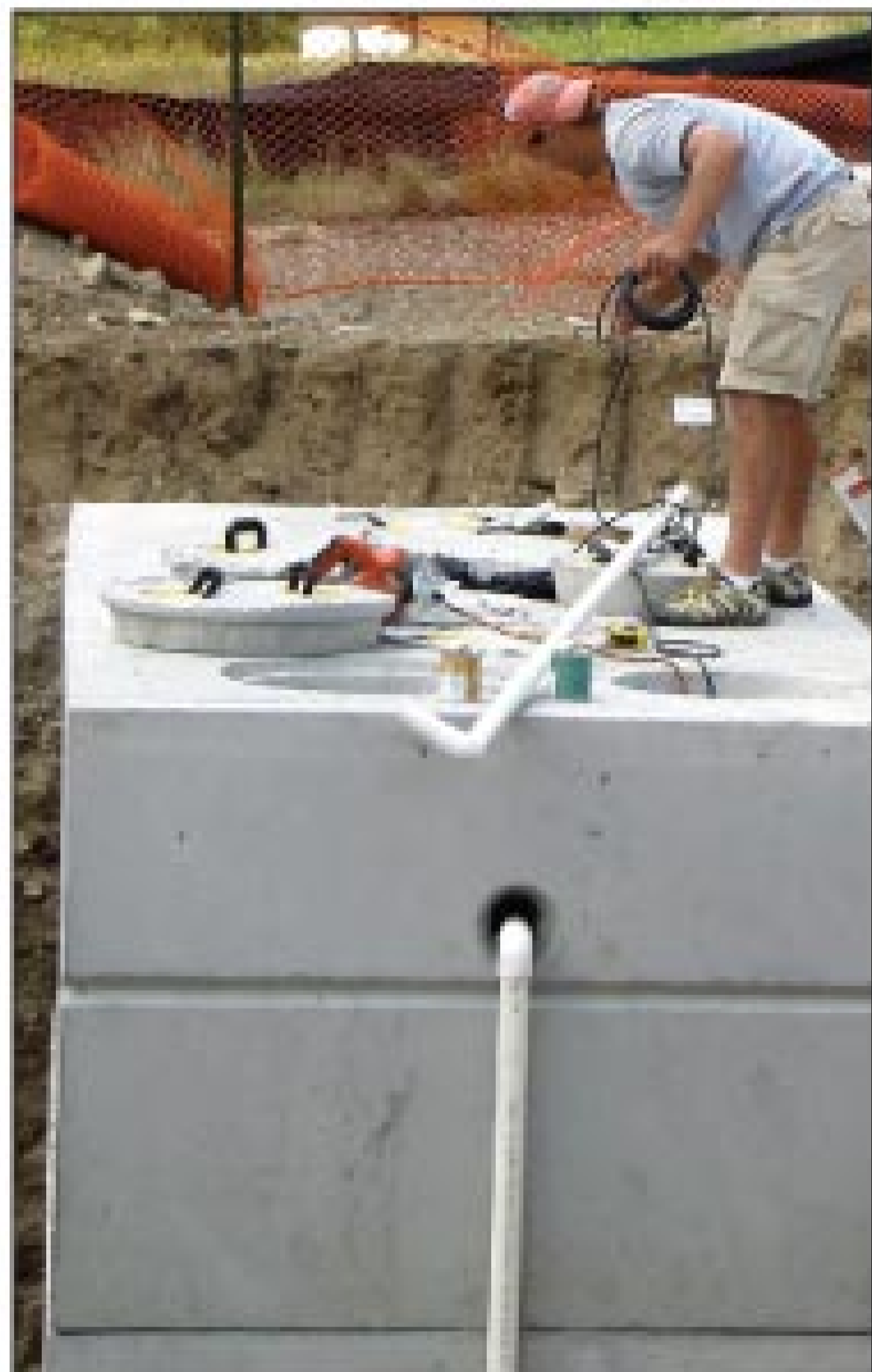
Tony DeGidio works on the bioreactor's electrical wiring.
