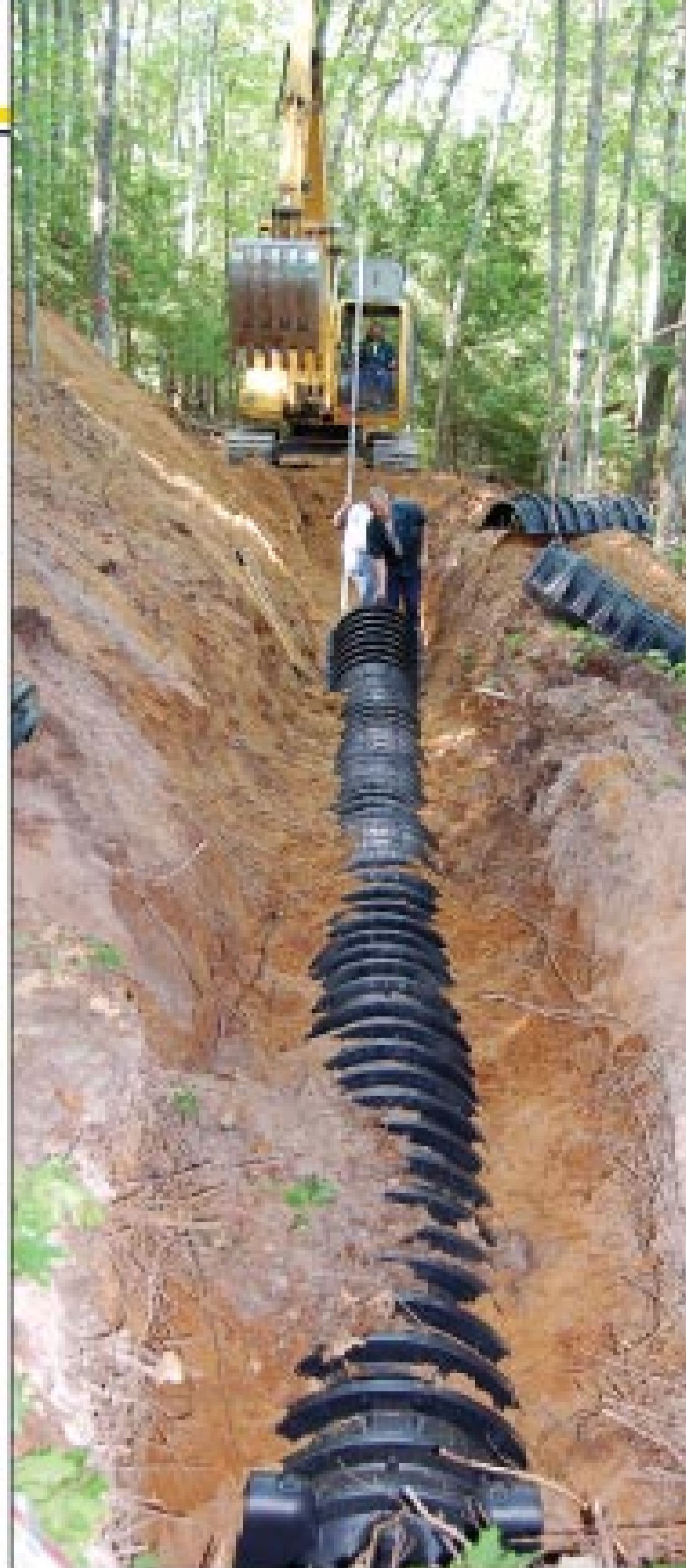
Clockwise, from top left: Chambers are laid in the first of two trenches; John Hoban manipulates the John Deere excavator; Todd Schrom hand-carries chambers for placement in a trench; Schrom (foreground) and Brian Grundy position the septic tank.
