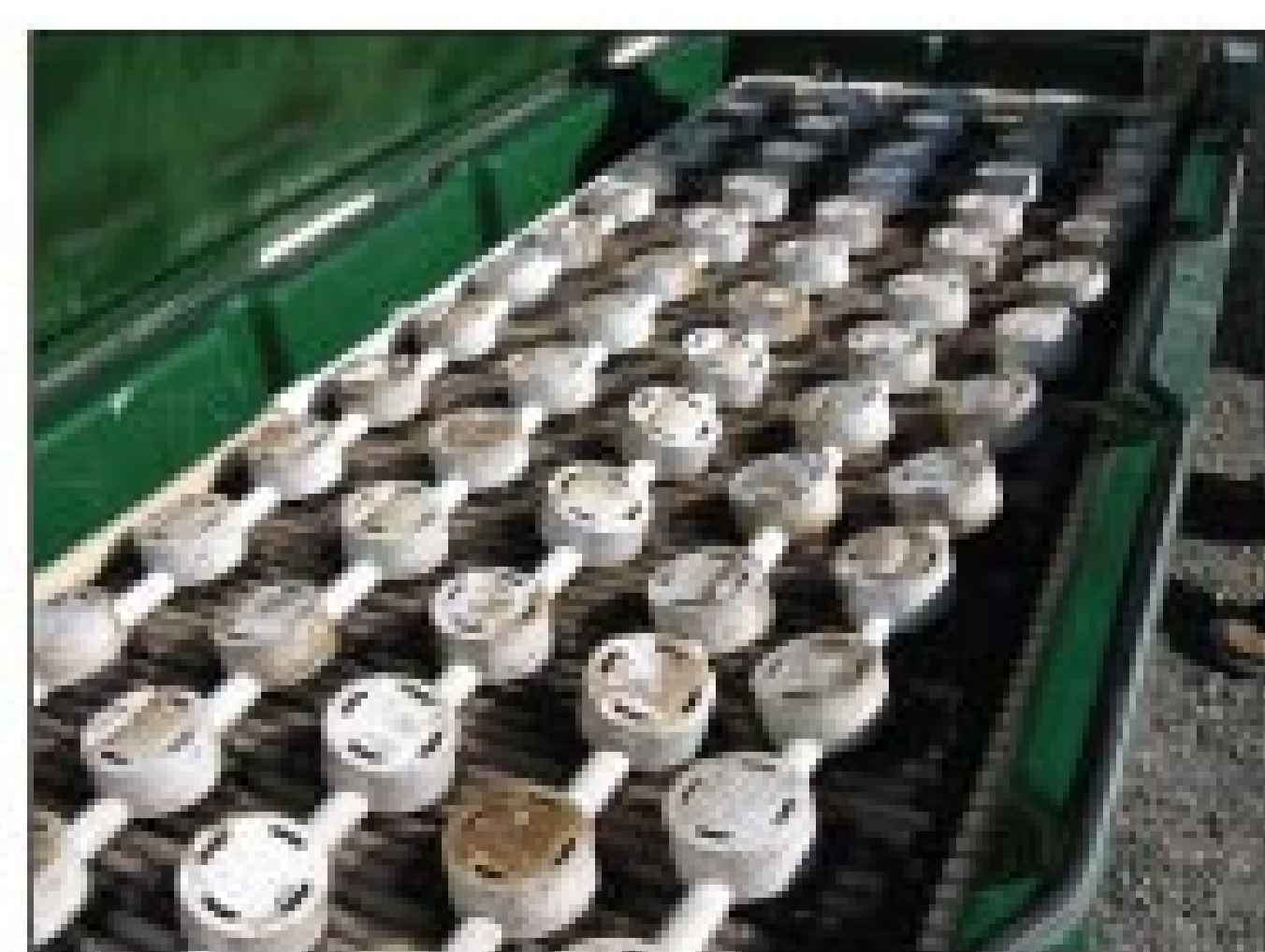
A media filter that can be used to clean up effluent.
