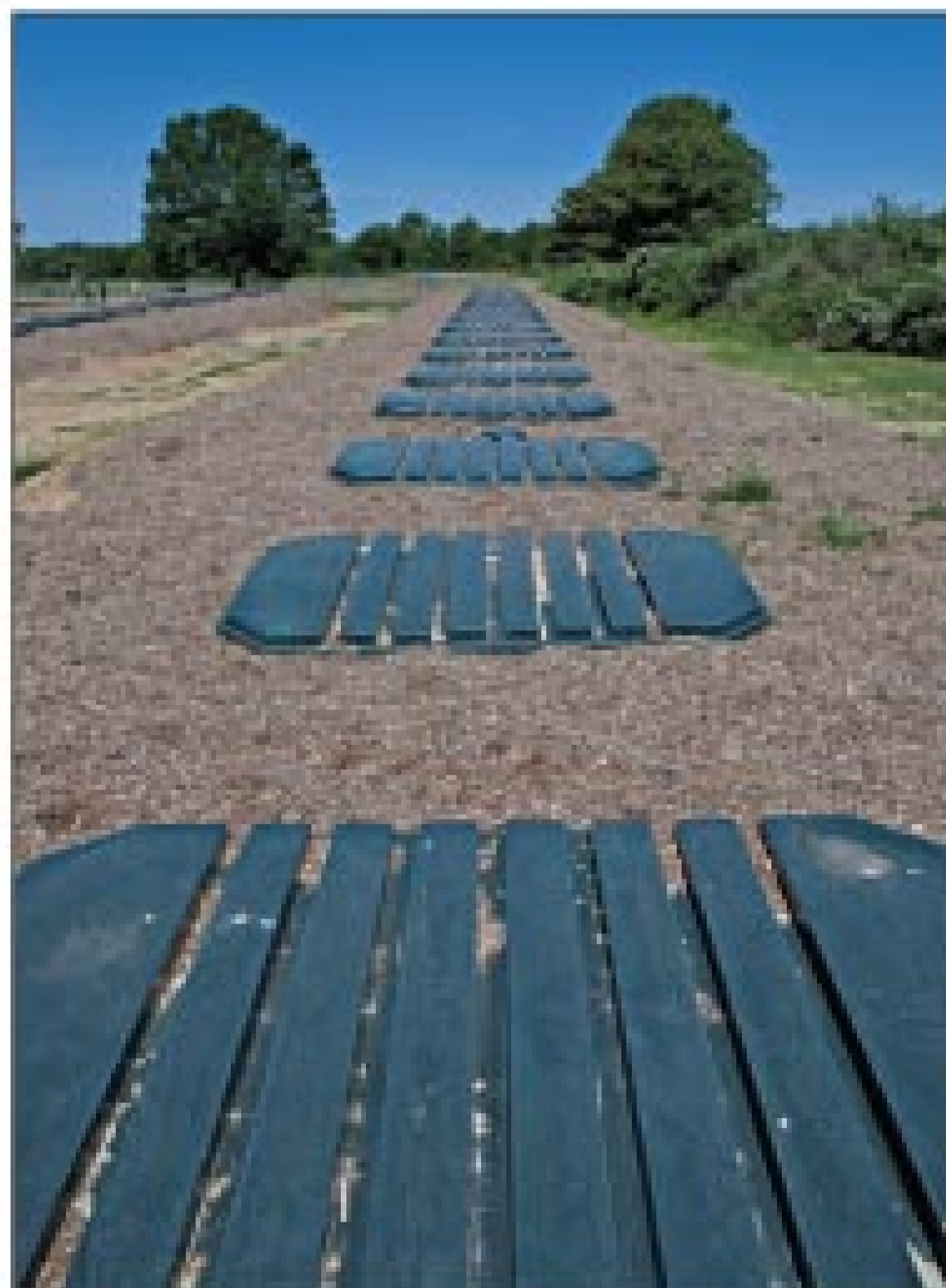
Bord na Mona peat biofilter systems are among the alternative systems the company installs to accommodate the diverse soils in the company’s service area.
