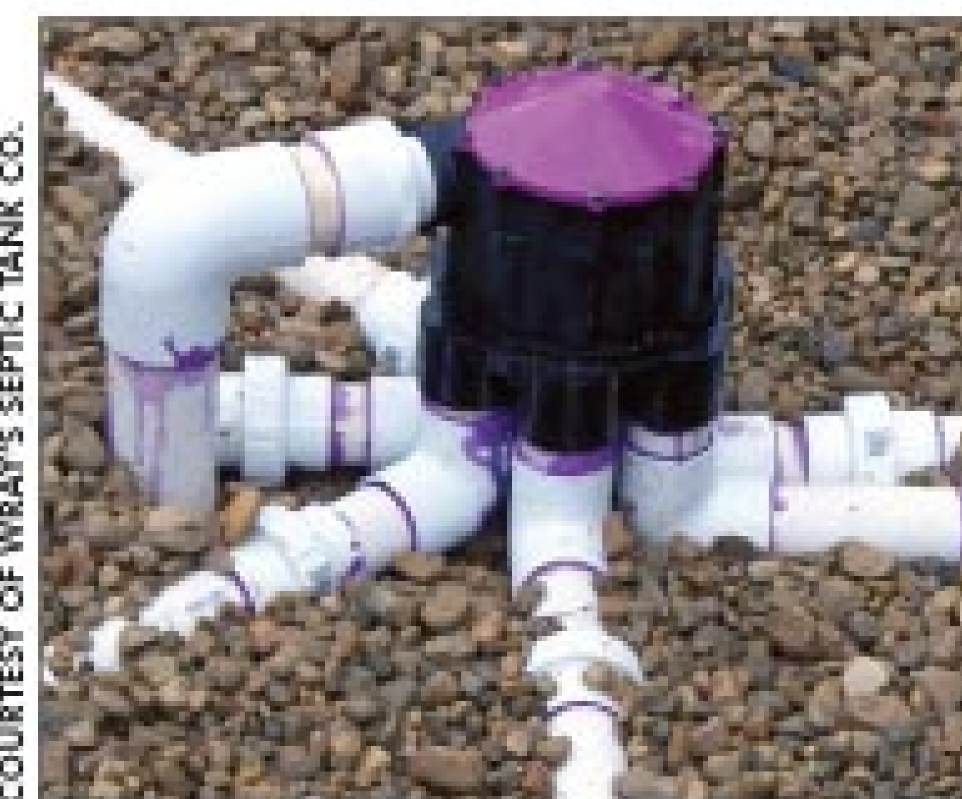
A Hydrotek 6606 valve in the center of the field splits the flow through a 1.5-inch header to six zones.
