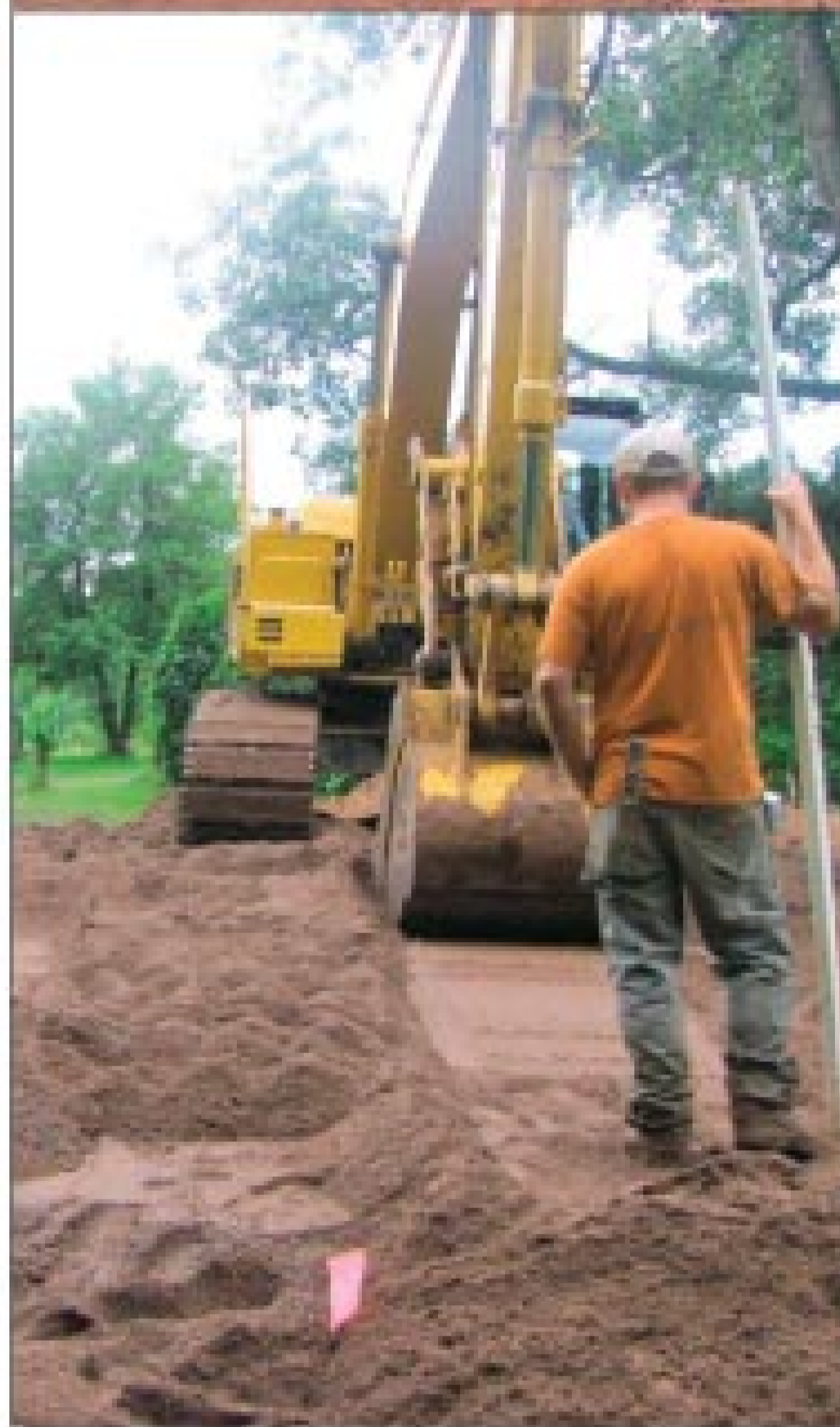
Project manager Greg Brown from Brown Plumbing and Heating uses a laser to set the elevation on a 4-foot-wide trench.
