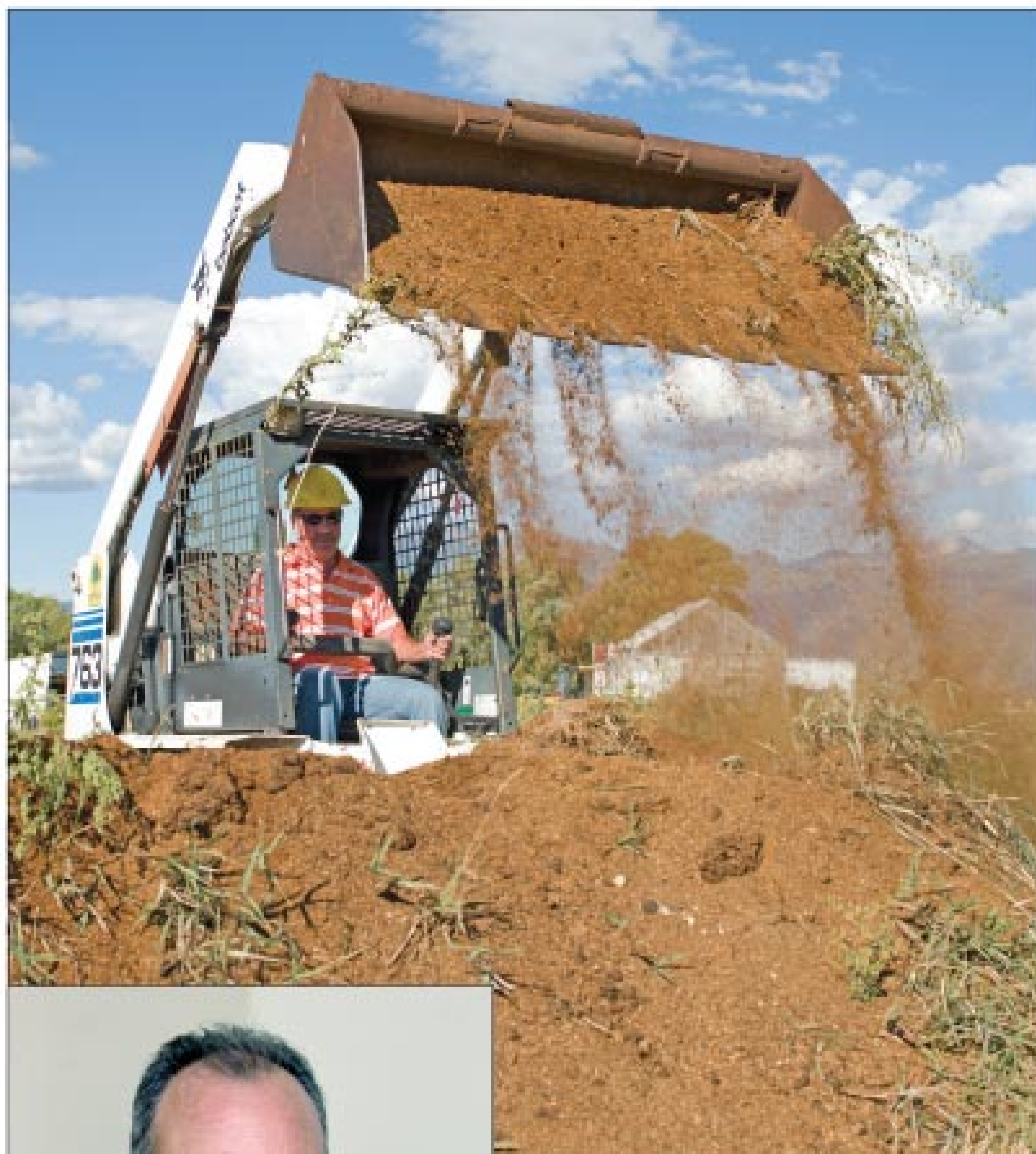
Scott Johansson, owner of Alta Perc Testing, is shown at the left and on his Bobcat 763 skid-steer loader as he spreads topsoil for finish on a drainfield.
