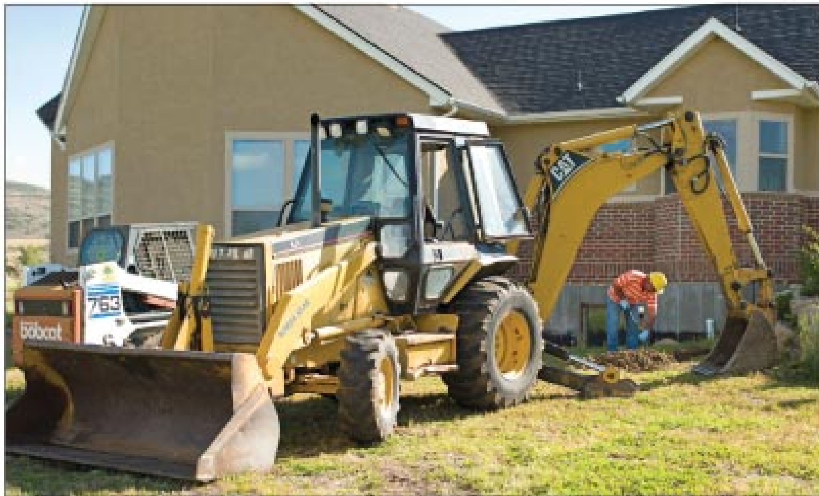
Johansson, with his Cat 416B backhoe and front-end loader, does a routine inspection of an existing septic system.
