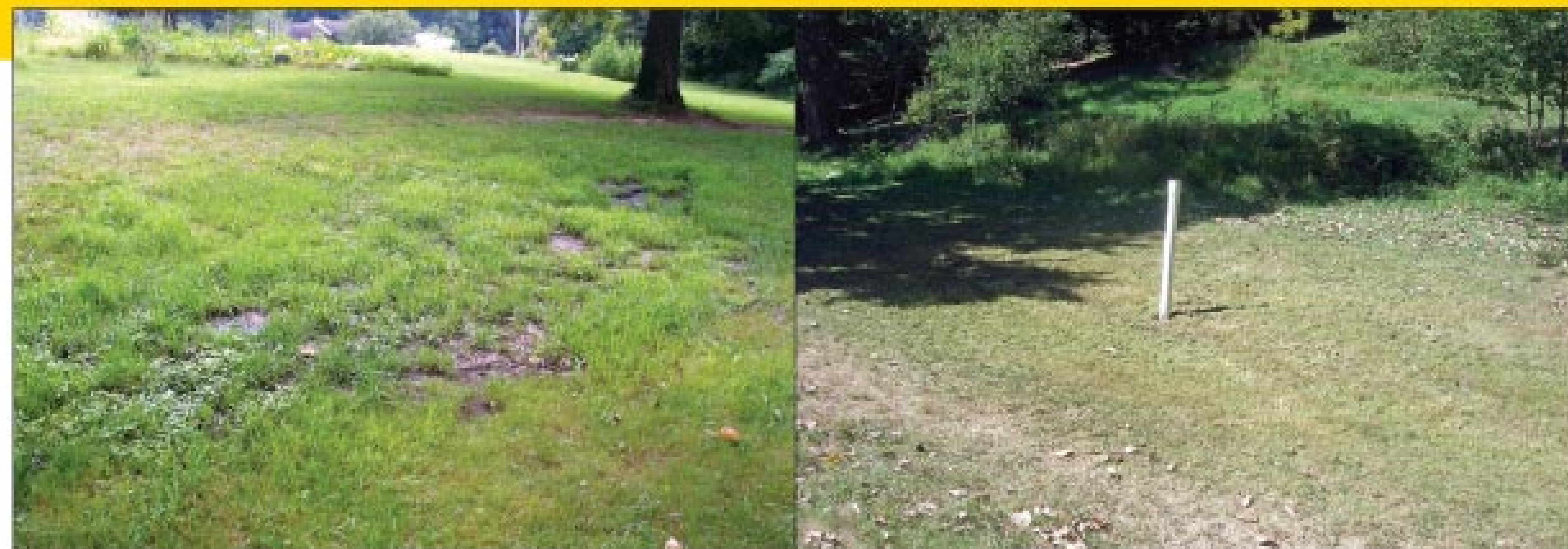
Left, the drainfield before installation of the new system: There is ponding as the field was plugged. Right, after installation, all ponding has disappeared.
