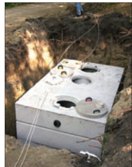
Many local codes require dual-compartment tanks.
