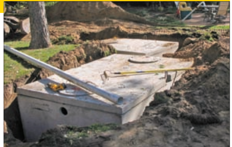
Sometimes it is necessary to use more than one tank in series to provide adequate capacity.
