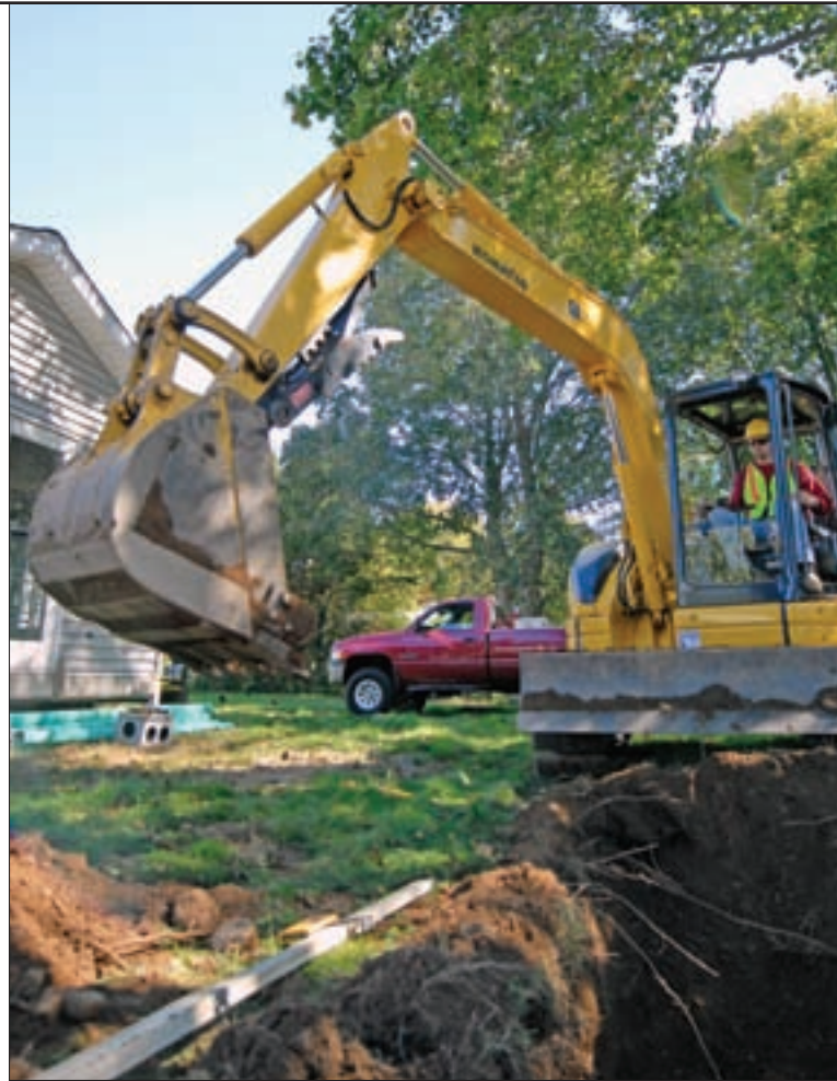
With a zero-tail-swing excavator, Jason Walter can get any job done, large or small.
