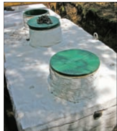
A spray-on insulation can keep the tank from freezing and act as a seal of the seams.
