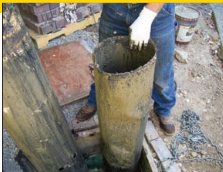
A properly designed system includes an effluent screen in the septic tank. If no screen is installed, or if the design employs a two-compartment tank, a pump screen should be installed to prevent fouling of the pump or transfer of unwanted solids to the soil treatment area.
