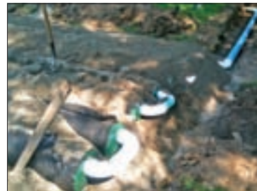
Offset adaptors cap the ends of the pipe. They accept a 4-inch PVC 90-degree elbow that connects to a short length of pipe to join two rows.
