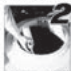
Place ring over opening and apply foam.
