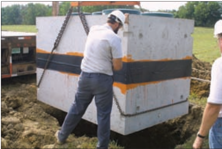
Tanks with mid-wall seams need to have those seams properly sealed before installation.
