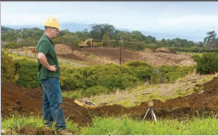
Gabe Hoeffken overlooks a recently dug leachfield for a septic system.
