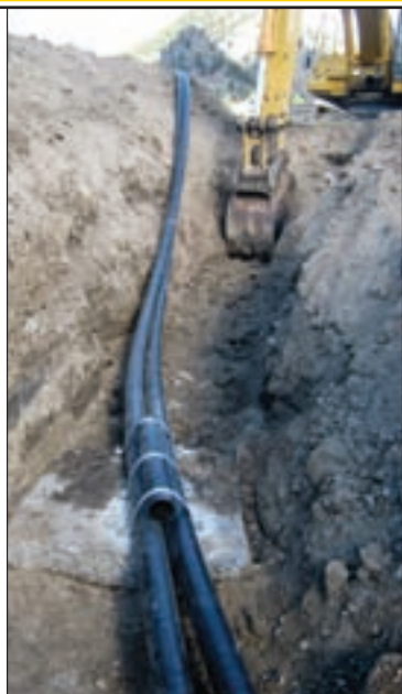
Workers lay 3,000 feet of 4-inch 160 psi DR 11 HDPE force mains down the highway department right-of-way.
