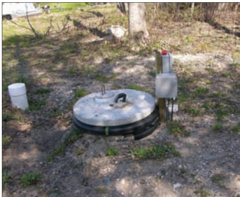
A pump tank with controls and alarm as well as a riser brought to the surface.
