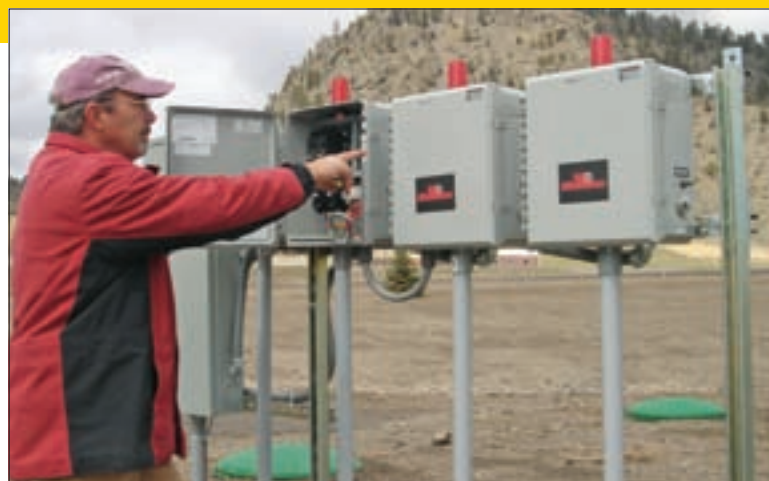
Steve Durkin, caretaker of the Dearborn highway rest area, takes readings from the onsite treatment system control panel.
