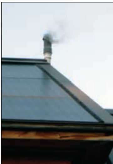
It's not a new Pope, but assurance that the roof vent for the plumbing was clear.
