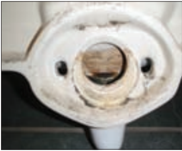
ABOVE: The smoking gun: Smoke from behind a urinal is proof positive that the leak was the plumber's fault and not the septic system installer's. LEFT: The back of the removed urinal shows where the seal slipped down during installation, keeping water from leaking out the bottom but letting sewer gases out the top.
