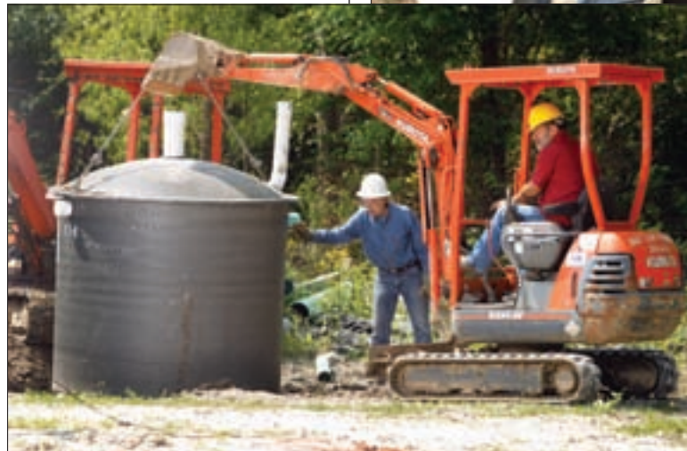
A tracked mini-excavator comes in handy as Phillip Butler, left, and Woody Watson place an ATU.
