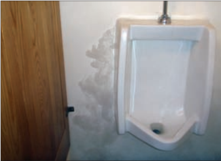
ABOVE: The smoking gun: Smoke from behind a urinal is proof positive that the leak was the plumber's fault and not the septic system installer's. LEFT: The back of the removed urinal shows where the seal slipped down during installation, keeping water from leaking out the bottom but letting sewer gases out the top.
