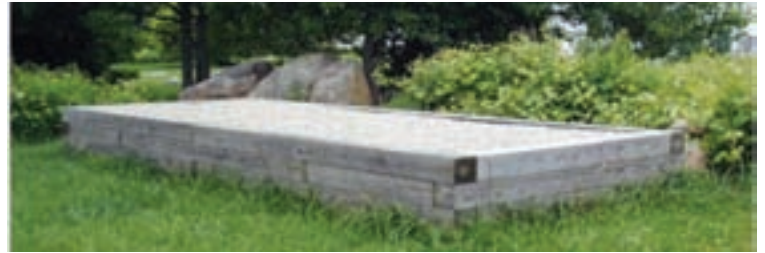
ABOVE: Single-pass sand filter with underdrain.
