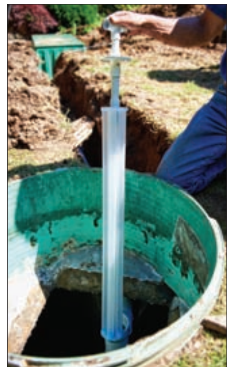
A 4-inch Orenco biofilter is installed in a primary processing tank.
