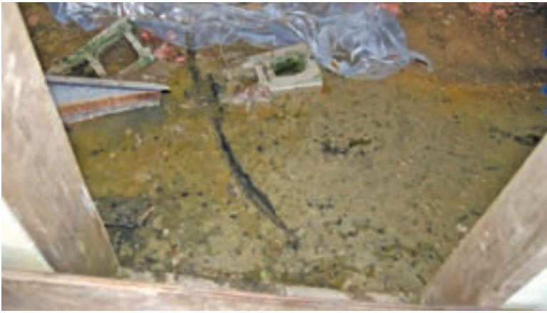
TOP: Raw sewage ponds in the northeast corner under the mobile home. RIGHT: A leak in the hose surprises TR Davis employee Michael Rakes as he fills the septic and dose tanks half-full of water.
