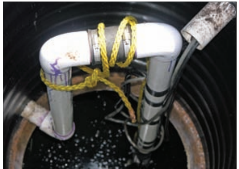
A quick-disconnect coupling with a rope to help extract the pump is part of a quality pump installation.
