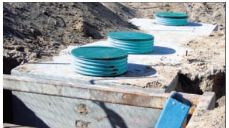
TOP: Straps and turnbuckles secure the 3,000-gallon Xerxes septic tank to the concrete deadmen. RIGHT TOP: The discharge side of the Advan-Tex AX-MAX module shows the textile media, distribution manifold with spray nozzles, vent fan, and recirculation piping. RIGHT BOTTOM: The 2,500-gallon concrete sand trap at Restroom One collects water from four outdoor showers. Fines settle out before the water discharges in the septic tank.
