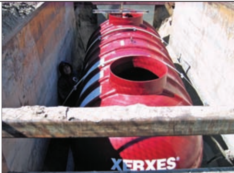
TOP: Straps and turnbuckles secure the 3,000-gallon Xerxes septic tank to the concrete deadmen. RIGHT TOP: The discharge side of the Advan-Tex AX-MAX module shows the textile media, distribution manifold with spray nozzles, vent fan, and recirculation piping. RIGHT BOTTOM: The 2,500-gallon concrete sand trap at Restroom One collects water from four outdoor showers. Fines settle out before the water discharges in the septic tank.
