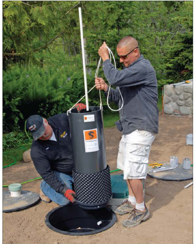
Above: Doug and Mike Fellner lower a SludgeHammer S-86 unit into a treatment tank. Below: Mike Soukup left, and Mike Fellner cut slits in the fabric and install inspection ports on either end of the drainfield media.
