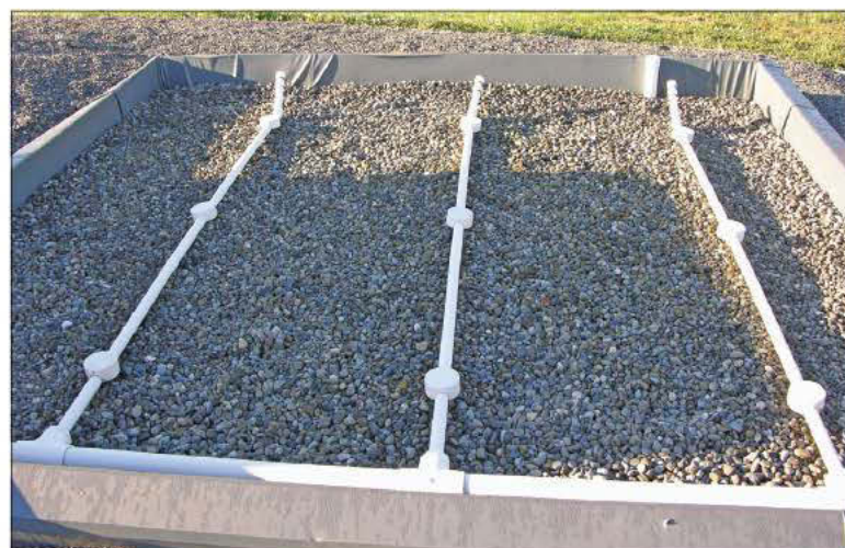
A pressure distribution system over a sand filter before backfilling. Effluent is applied to the rock at the surface.
