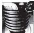
Place plastic maintenance pipe on ring.
