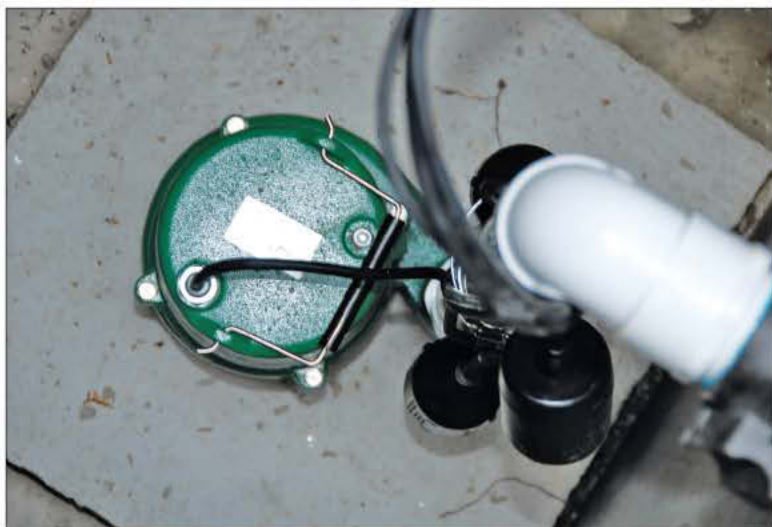
The Hydromatic SHEF 40 pump with Septic Products control floats will convey waste from a below-ground tank to the above-ground drainfield.
