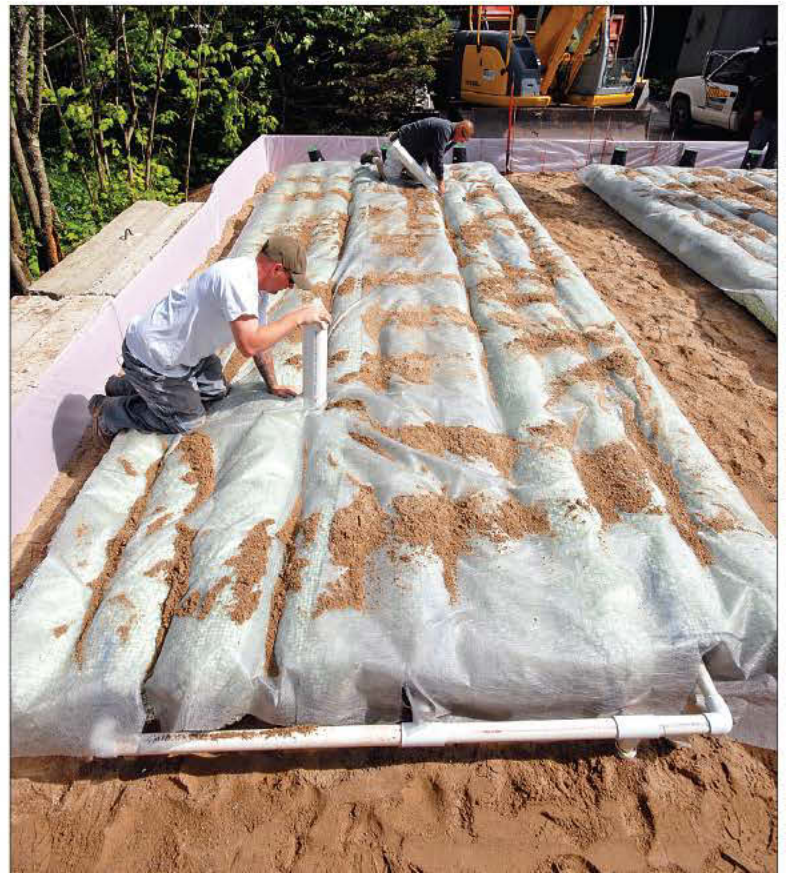
Above: Doug and Mike Fellner lower a SludgeHammer S-86 unit into a treatment tank. Below: Mike Soukup left, and Mike Fellner cut slits in the fabric and install inspection ports on either end of the drainfield media.
