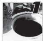
Apply foam sealant to tank.
