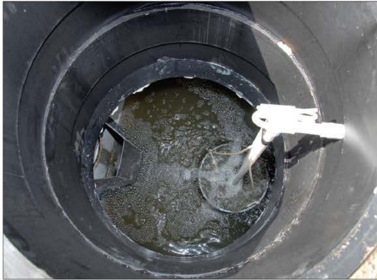
The SludgeHammer unit is powered up after installation.
