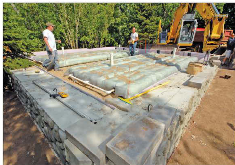
The raised mound system includes two 9- by 20-foot drainfields using Flowtech geosynthetic aggregate from ICC Technologies, enclosed by a concrete retaining wall. (Photography by Jim Kneiszel)
