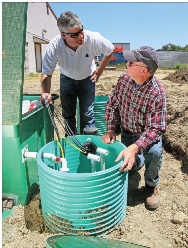
Ryan Pearson, owner of Pearson Exploration, and onsite consultant Mike Treinen inspect a recently installed AdvanTex (Orenco) treatment system pump unit.
