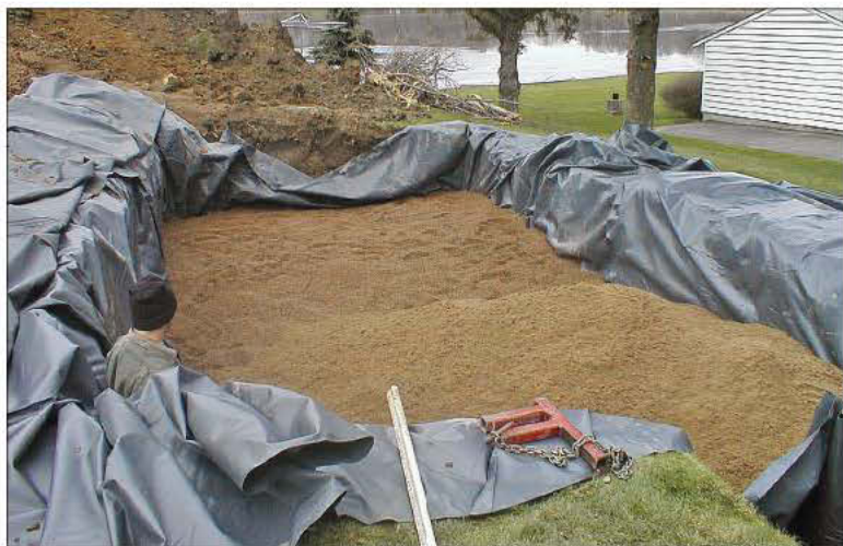
A liner is placed in an excavation for a sand filter; some of the media is already in place.
