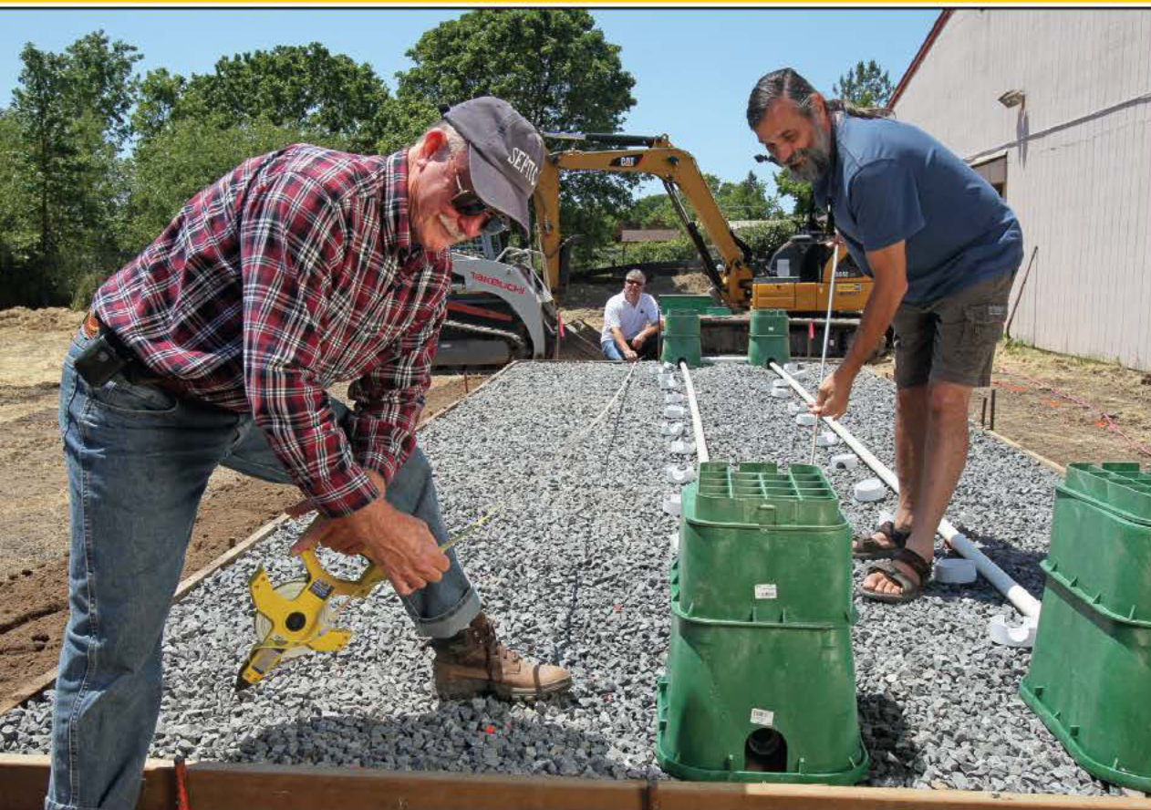
Mike Treinen and Frank Dono, REHS, take drainfield measurements during system construction.
