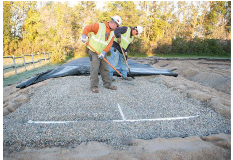
LEFT: Onsite technicians Cameron Deleski and Randy Storey attach the risers from Polylok. RIGHT: Storey and lead onsite technician Deleski rake the rock over the pipes in a mound system.
