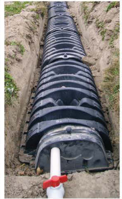
LEFT: An engineered aggregate system greatly simplifies installation. RIGHT: Chamber installations have become extremely common alternatives to conventional aggregate in many regions.
