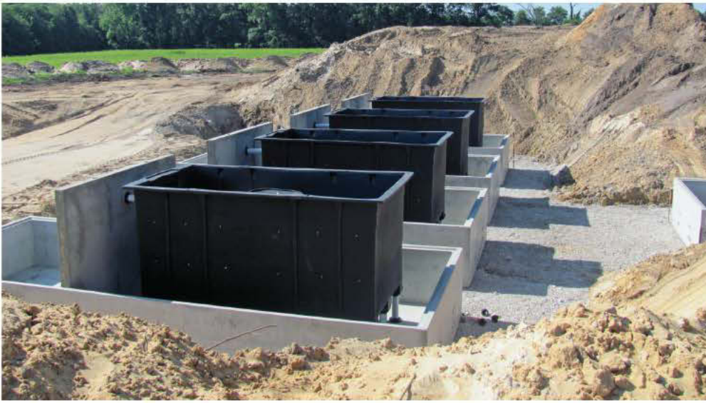
LEFT: Four high-strength FAST treatment units from Bio-Microbics were installed in the 9,000-gallon compartment of the 15,000-gallon tanks. RIGHT: Scott Rexroth of Clear Water Environmental Systems installs one of two Polylok 10,000 gpd PL-525 effluent filters in the outlet riser of the 6,400-gallon septic tank.
