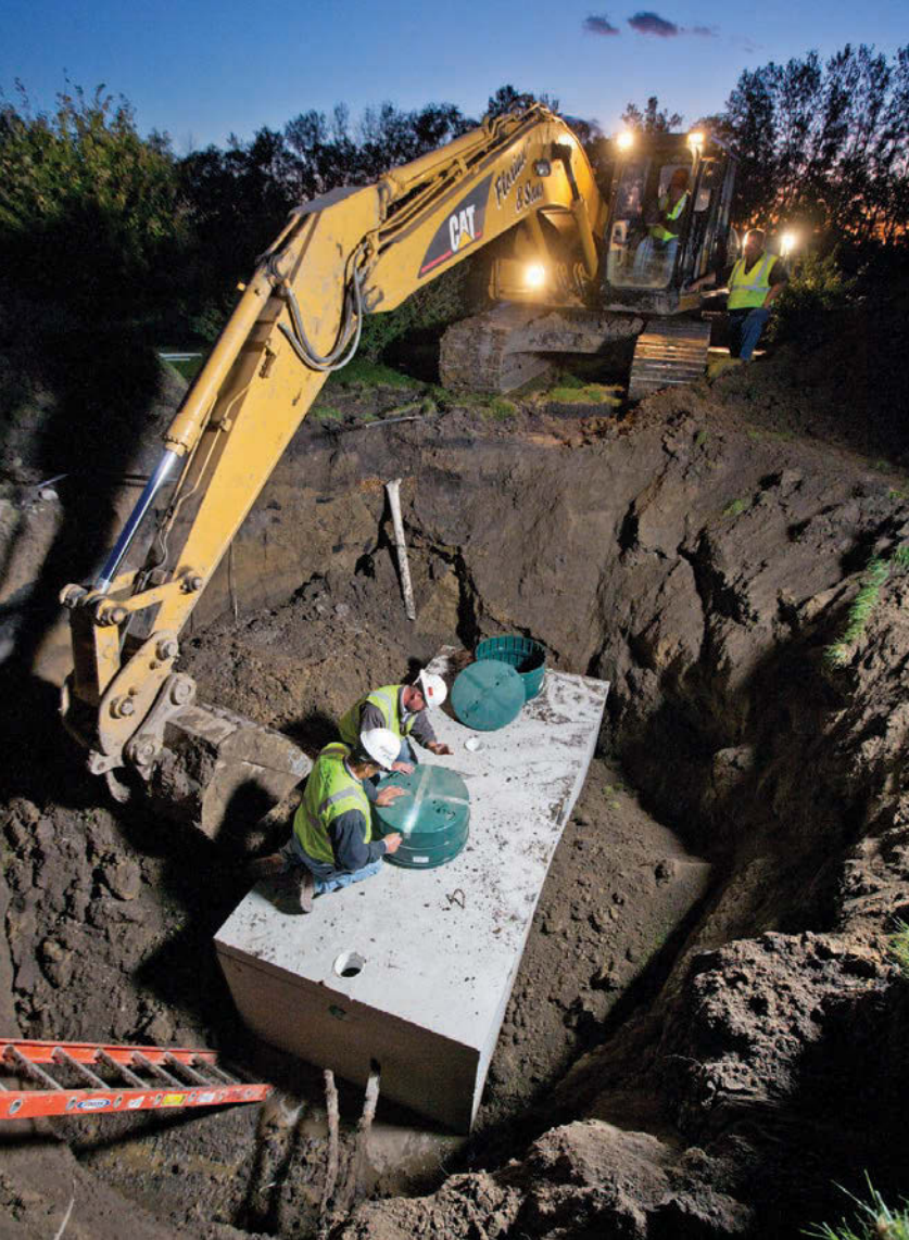
LEFT: Onsite technicians Cameron Deleski and Randy Storey attach the risers from Polylok. RIGHT: Storey and lead onsite technician Deleski rake the rock over the pipes in a mound system.
