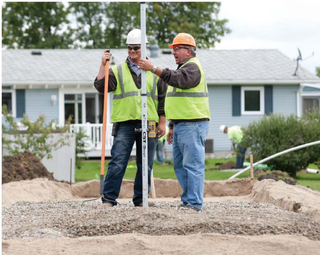
Onsite technician Randy Storey and owner Glen Gonsorowski stand atop a new mound system.
