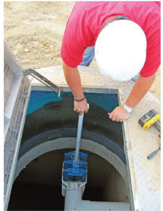
LEFT: Four high-strength FAST treatment units from Bio-Microbics were installed in the 9,000-gallon compartment of the 15,000-gallon tanks. RIGHT: Scott Rexroth of Clear Water Environmental Systems installs one of two Polylok 10,000 gpd PL-525 effluent filters in the outlet riser of the 6,400-gallon septic tank.
