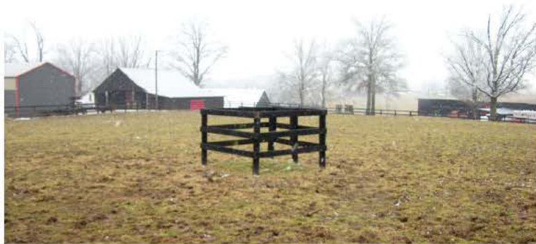
Horses and other livestock should be kept off the drainfield. Here, the distribution box is protected by a fence.
