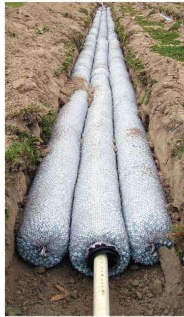
LEFT: An engineered aggregate system greatly simplifies installation. RIGHT: Chamber installations have become extremely common alternatives to conventional aggregate in many regions.
