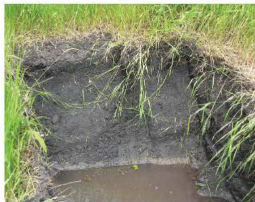
One key to good installations - and generally a code requirement - is to maintain proper separation distance between the system and the water table.
