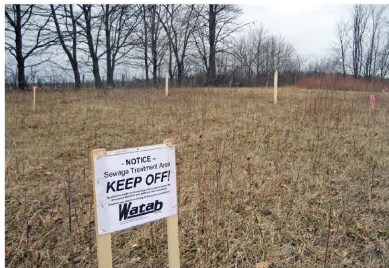
The drainfield site should be protected from traffic that can cause soil compaction.
