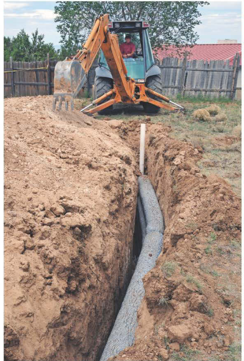
Orlando Sanchez installs EZflow drainfield media from Infiltrator Systems.
