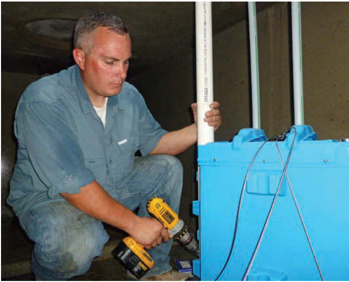
Ryan Spiers of Alternative Wastewater Systems plumbs the 60-pound membrane unit.
