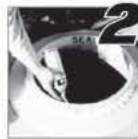
2 Place ring over opening and apply foam.
