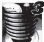
3 Place plastic maintenance pipe on ring.
