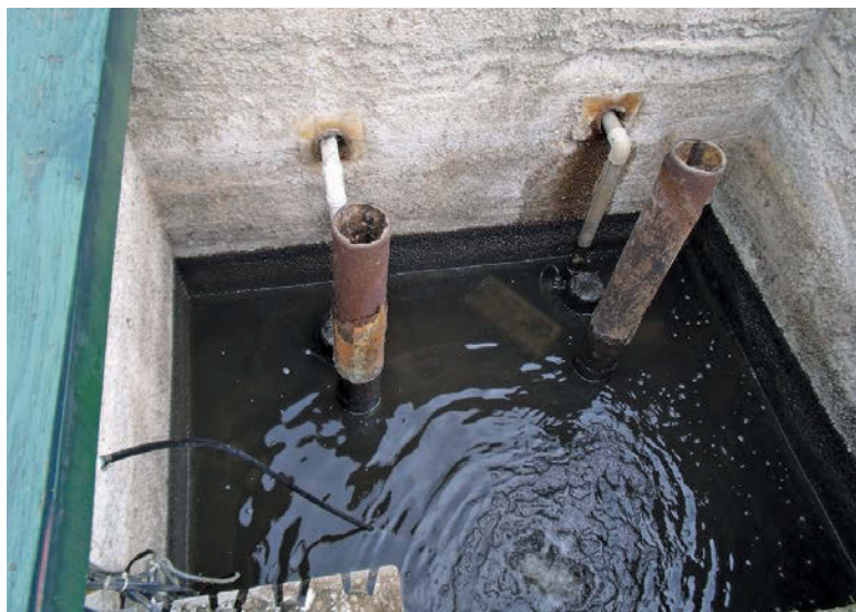
ABOVE: An air hose feeds a diffuser in the dosing station to prevent the water from going semi-anaerobic. RIGHT: A staff member checks one of the four effluent filters. The electrical service panel is on the pole in the background.
