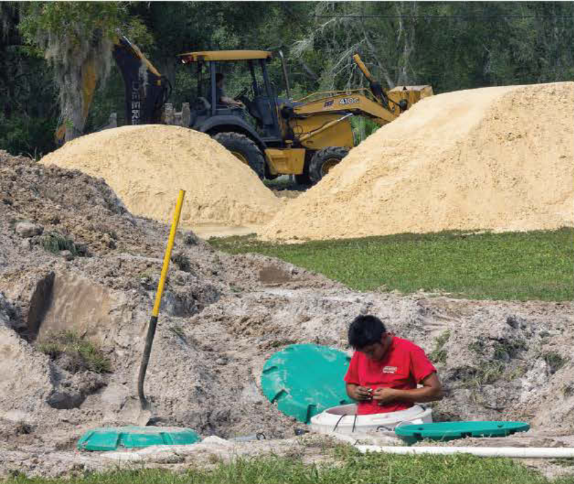
Installer Nahum Sotelo works on a residential installation of a tank from Snyder Industries.
