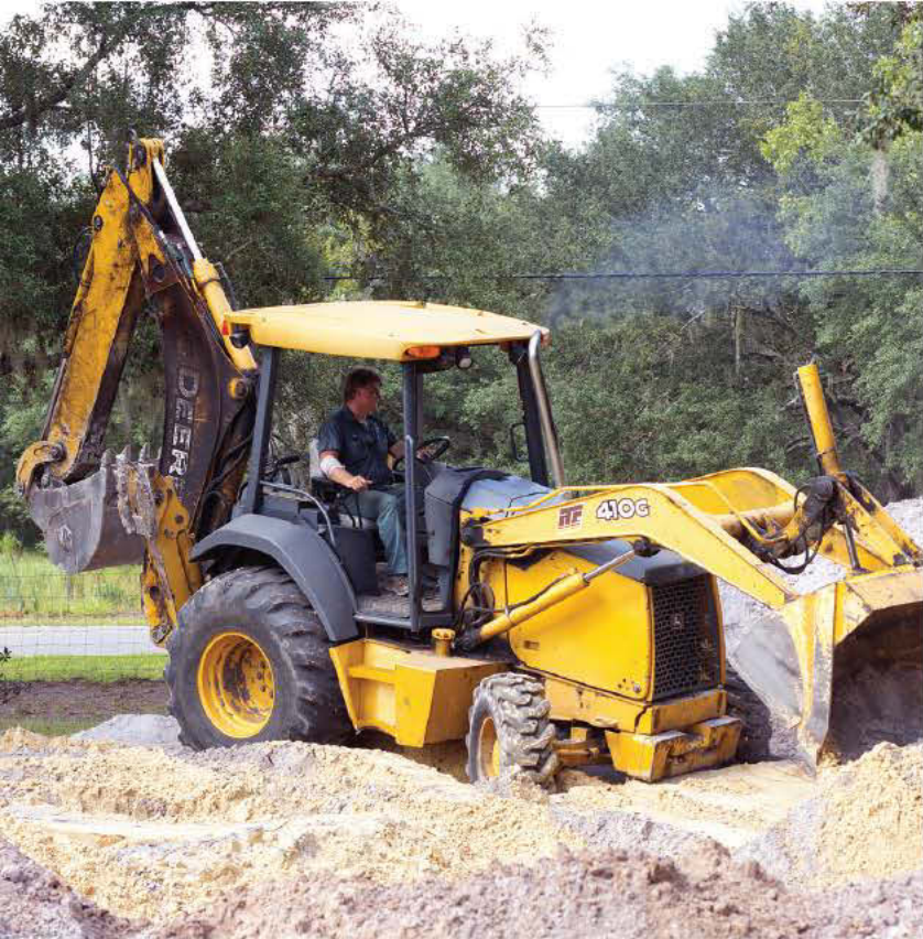
Bryan Turner, vice president of Turner's Septic Service, uses a John Deere backhoe to prepare a drainfield.
