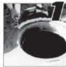
1 Apply foam sealant to tank.
