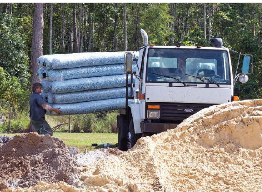
LEFT: Bryan Turner unloads EZflow drainfield media at an installation site in Interlachen, Fla. ABOVE: Installer Brandon Turner at the company’s lime stabilization plant in Bunnell, Fla.
