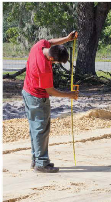
Installer Nahum Sotelo checks elevations on a drainfield.
