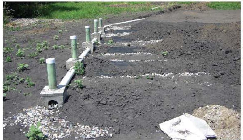
A drop box should be installed level and should include an inspection port.
