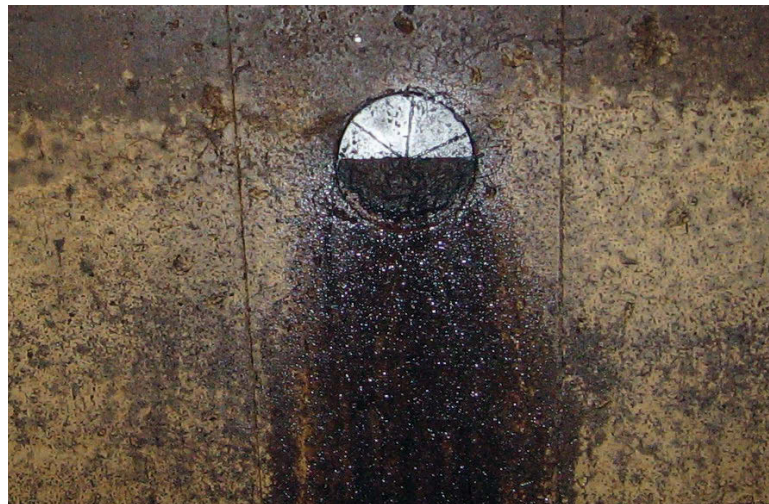
This is the inside of the holding tank for a church. It had been filling up with groundwater even while the church was not being used, requiring expensive pumping. The camera showed where the water was leaking in through a poorly sealed knockout.
