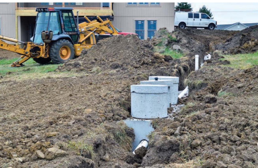
ABOVE: Norweco aerators and 1,000-gallon pump tank are part of a new installation in progress. RIGHT: Dan Owens connects fittings to supply and return lines in the trench.
