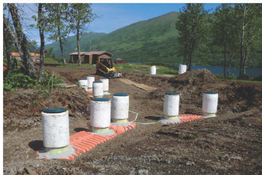
Ed Ward graded a slope, then used a sheet of plywood to drag the septic tanks into position. The middle riser in the front row marks the pump station. (Photos courtesy of Garness Engineering)
