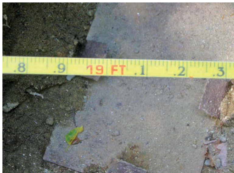
This photo reminded the author of the location of an old distribution box he had uncovered years ago. The tape measure told just how far out from the house to dig. It turned out that the pipe between the box and the septic tank had plugged with roots.
