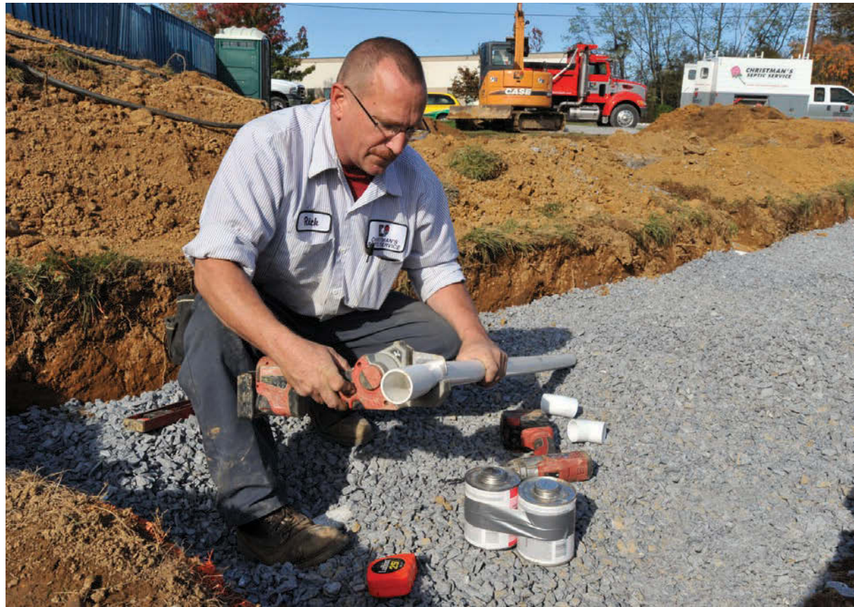
Crew member Rick Smith prepares piping for a drainfield.
