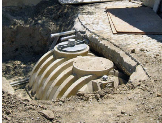
ABOVE: Burying the 750-gallon storage tank beside the footpath made room for a wall to the right. On demand, the delivery pump sends recycled water from the tank to the irrigation network. RIGHT: The expansion tank with the disinfection systems and electrical components on a 4-foot-square panel for easy mounting.
