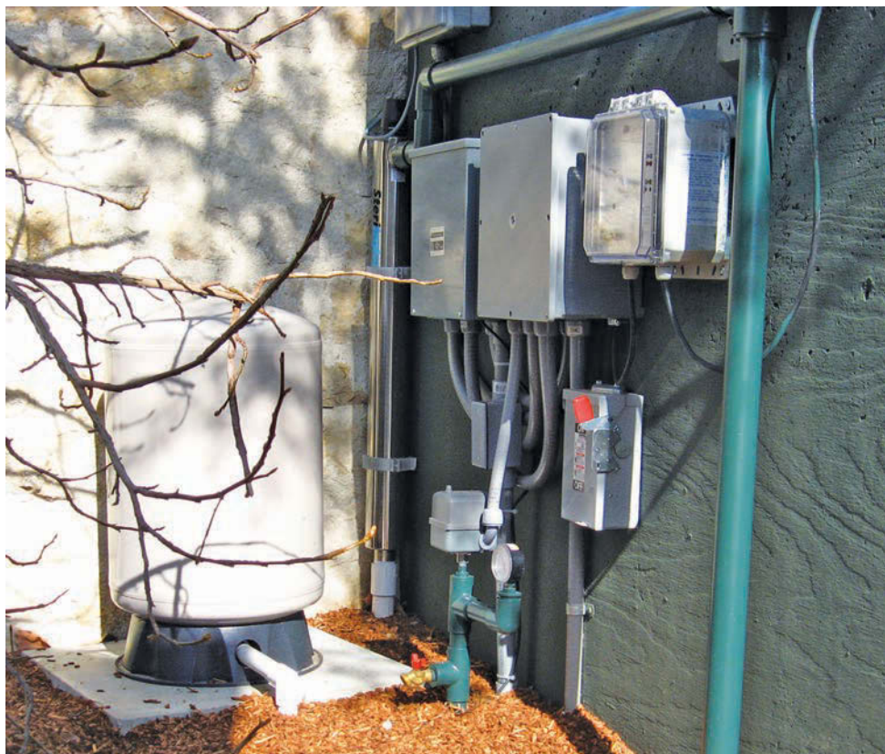
ABOVE: Burying the 750-gallon storage tank beside the footpath made room for a wall to the right. On demand, the delivery pump sends recycled water from the tank to the irrigation network. RIGHT: The expansion tank with the disinfection systems and electrical components on a 4-foot-square panel for easy mounting.
