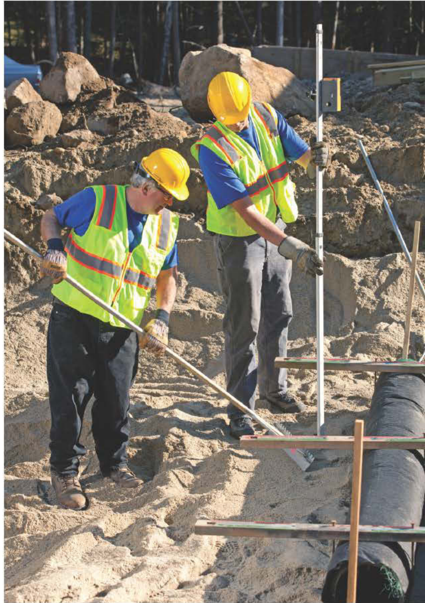
Hanna and Gerald use a transit to level a leach bed.
