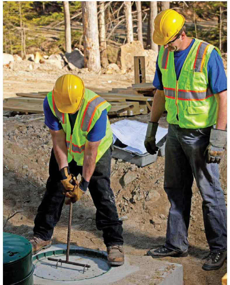
Hanna and Gerald check a Tuf-Tite inlet baffle (risers from Polylok).
