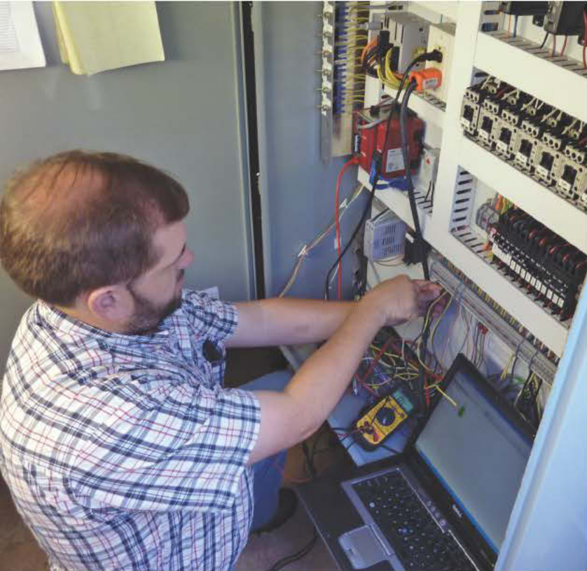
Engineer Adam Smith from Southeast Environmental Engineering wires the drip system's programmable logic controller with remote telemetry from Adenus Technologies.
