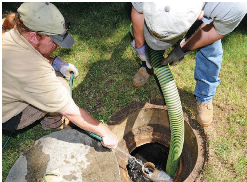
LEFT: The Buttermore's crew installs a plastic septic tank from Infiltrator Systems. ABOVE: Joe Wessell cleans and pumps out the septic system - maintenance is a significant part of the company's business mix.
