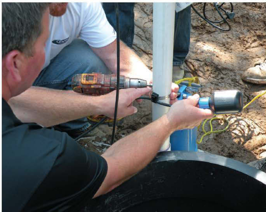
Floats must be installed properly so that the correct amount of effluent is delivered when the pump turns on.
