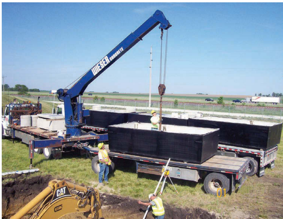
LEFT: Workers from Wieser Concrete prepare to set the bottom half of the dose tank. ABOVE: The 1/2 hp turbine septic tank effluent pump (STEP) vaults from Clarus Environmental.
