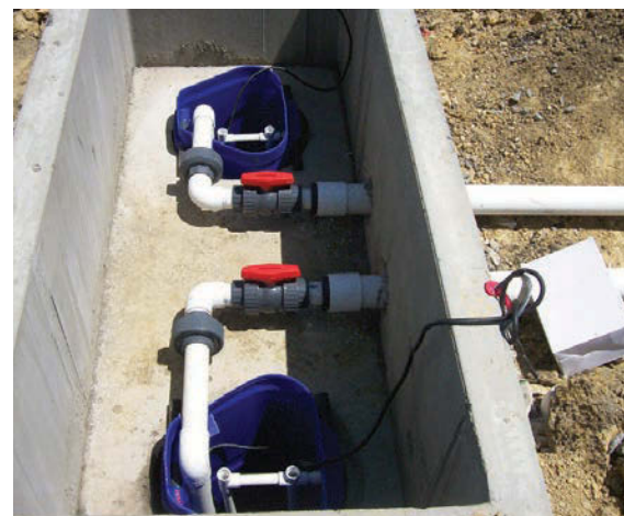
LEFT: Workers from Wieser Concrete prepare to set the bottom half of the dose tank. ABOVE: The 1/2 hp turbine septic tank effluent pump (STEP) vaults from Clarus Environmental.
