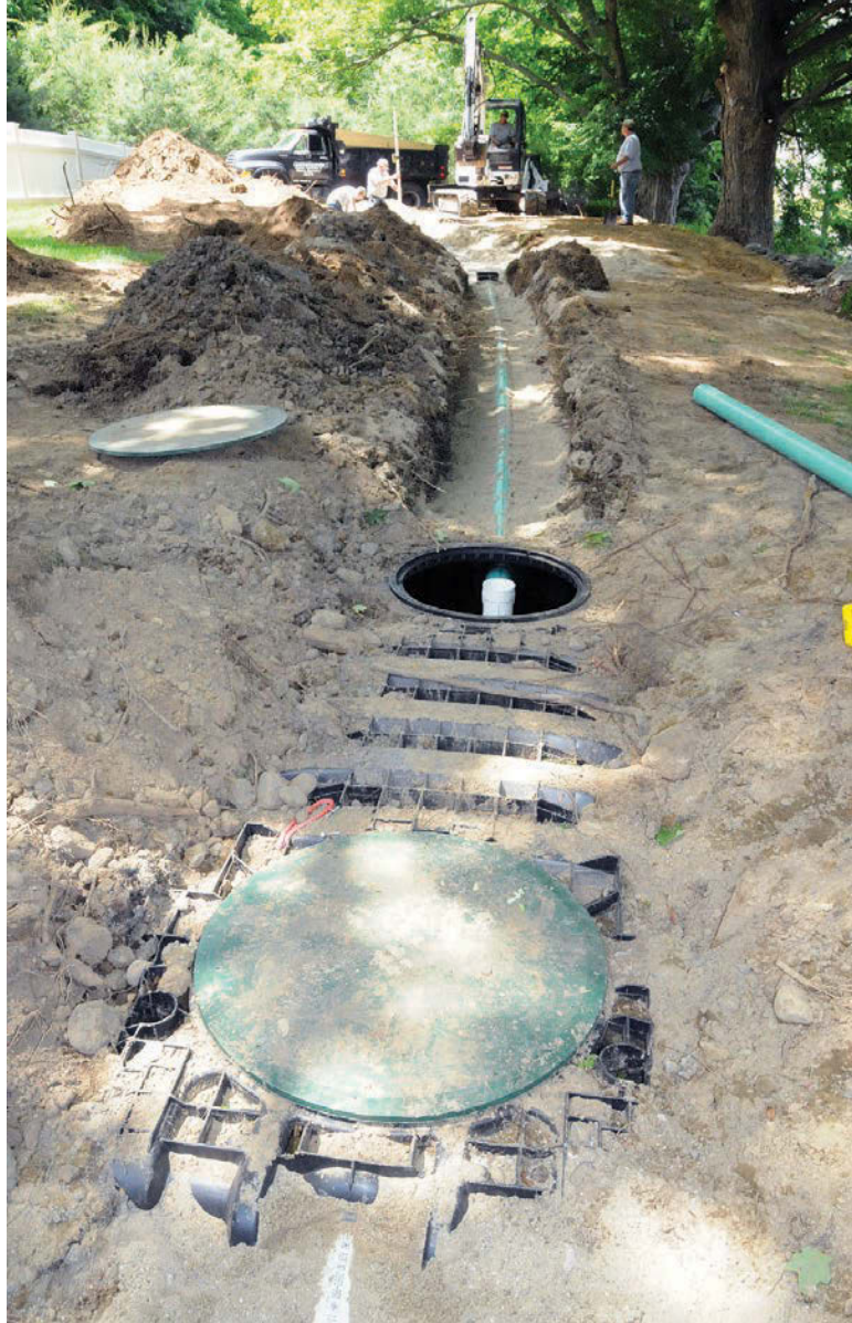
LEFT: The Buttermore's crew installs a plastic septic tank from Infiltrator Systems. ABOVE: Joe Wessell cleans and pumps out the septic system - maintenance is a significant part of the company's business mix.
