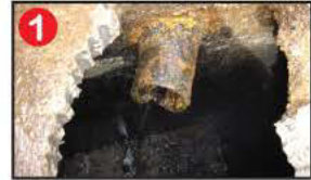
Before (Cast Iron Pipe)
