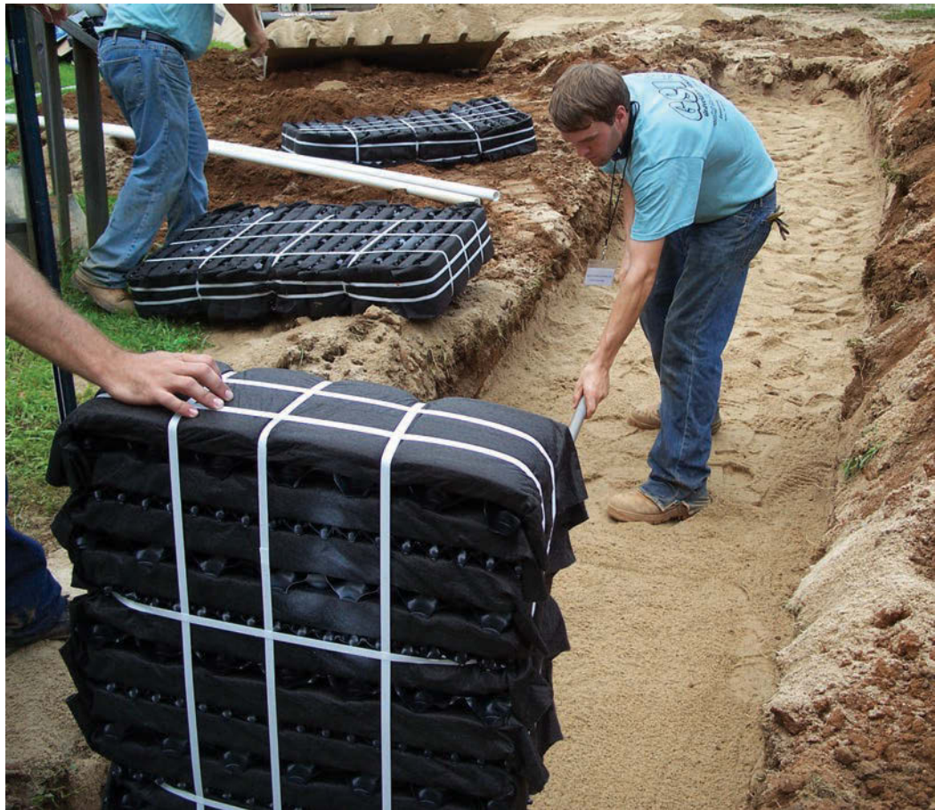
Field technician Justin Kilgore scarifies sand with a rake to ensure that effluent will move freely into it. (Courtesy of Twins Productions)
