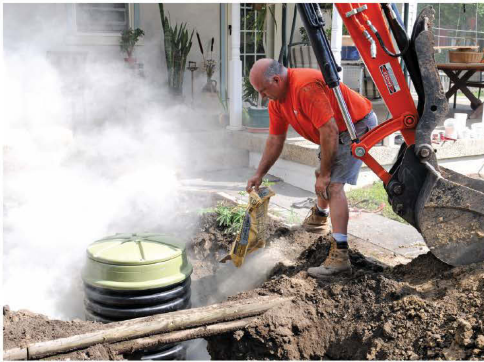
Andy Damiani adds concrete to balance an Environment One grinder pump.
