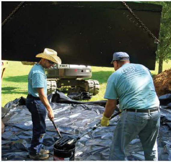
ABOVE: Gravelator Systems owner Harold Kilgore (right) and senior field technician Heath Kilgore apply the second coat of tar and polyethylene film to the dose tank to waterproof it. RIGHT: A crew installs primary treatment modules with orifice sleeves atop them. Eljen representative Jim King explains the procedure to other contractors.
