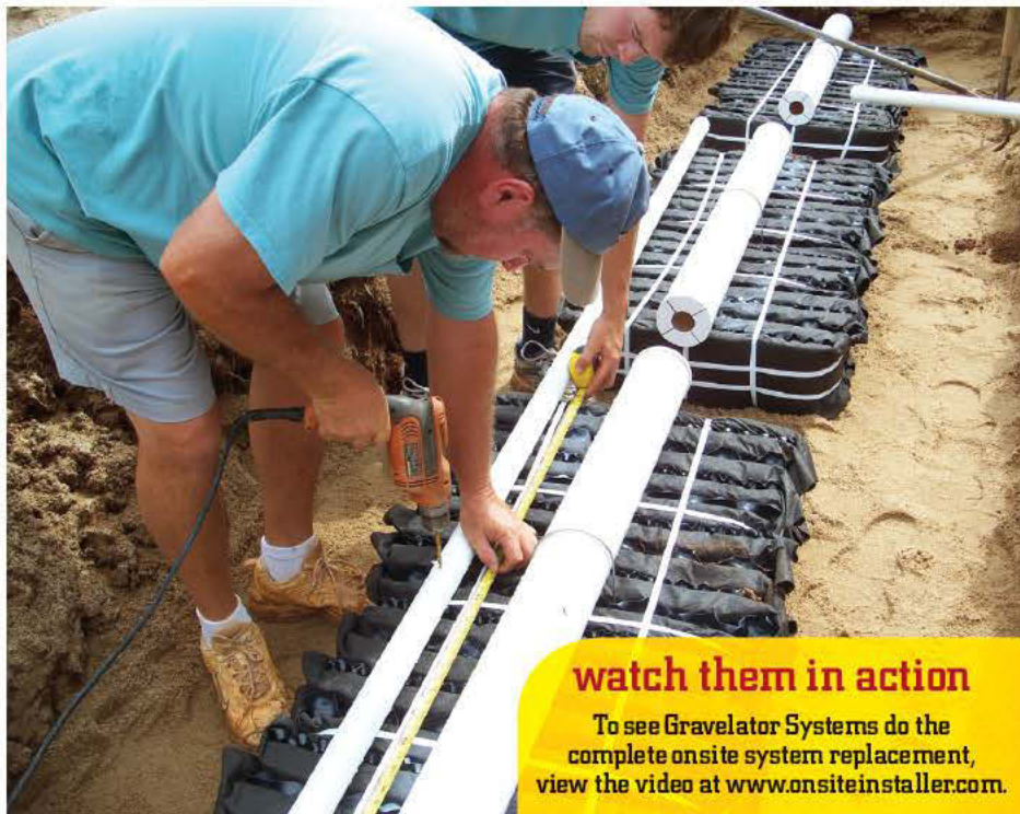
Harold Kilgore (left) and Justin Kilgore drill 0.25-inch orifices in 1.5-inch PVC low-pressure pipe.
