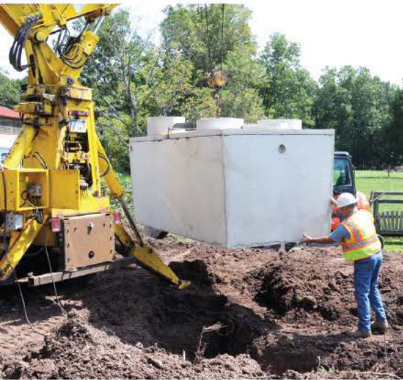
ABOVE: Andy Damiani helps guide a septic tank (Stauffer Concrete Products) into the ground. RIGHT: Damiani lays mastic concrete sealer around the openings in the tank top.
