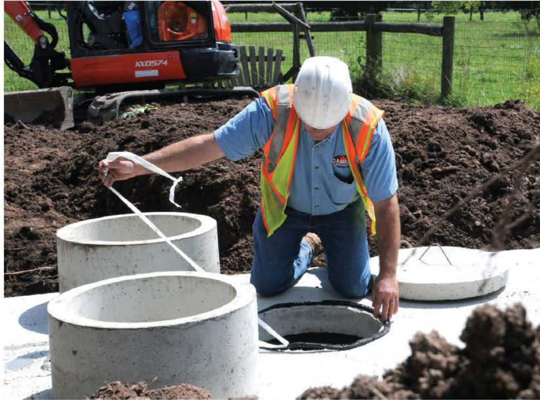
ABOVE: Andy Damiani helps guide a septic tank (Stauffer Concrete Products) into the ground. RIGHT: Damiani lays mastic concrete sealer around the openings in the tank top.
