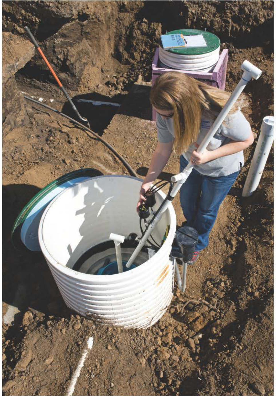
CHURCH Onsite partner Kate Carney examines a float tree from Orenco in a septic system.
