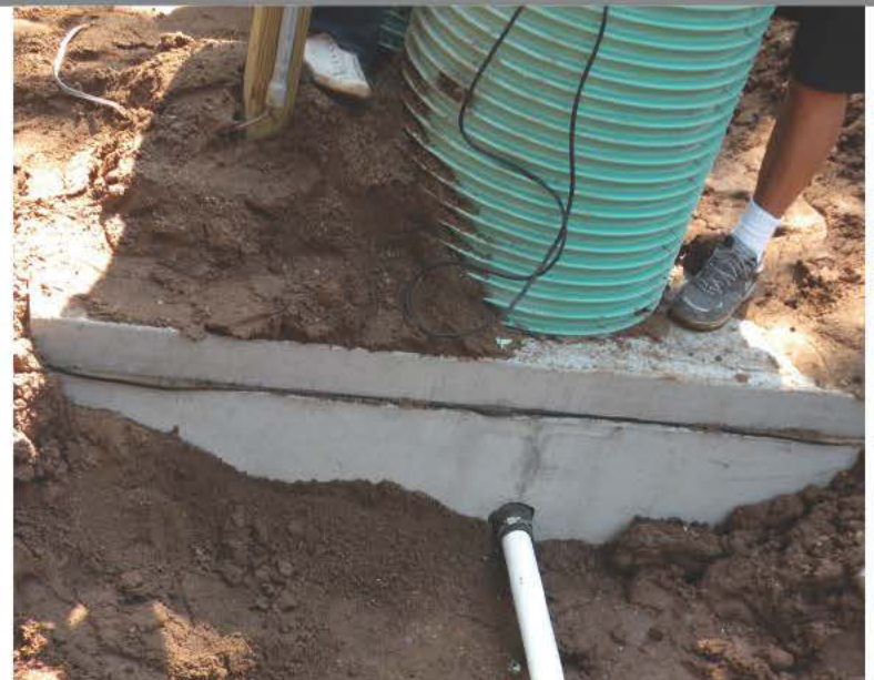
A concrete tank installation shows three critical locations that must be sealed properly to maintain a watertight tank: the inlet and outlets for the piping, the top seam, and the connection between the tank and the riser.
