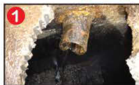
Before (Cast Iron Pipe)
