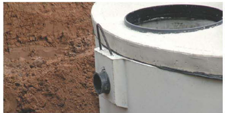
A concrete tank installation shows three critical locations that must be sealed properly to maintain a watertight tank: the inlet and outlets for the piping, the top seam, and the connection between the tank and the riser.
