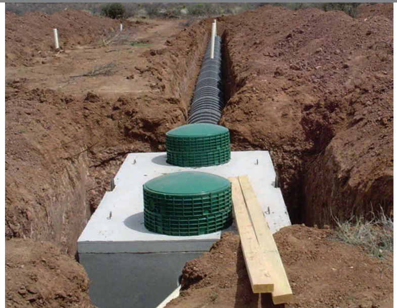
A concrete tank with a top seam and cast-in access risers is a good watertight tank option.
