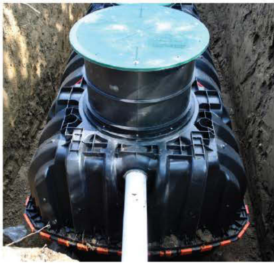
LEFT: The inlet and outlet piping and the access risers should also be watertight. ABOVE: Injection-molded parts on plastic septic tanks allow precise wall thickness. A continuous gasket is physically locked in place to ensure watertight conditions.
