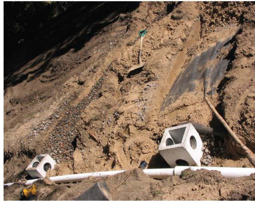
Drop boxes are being installed where rock is the drainfield media.
