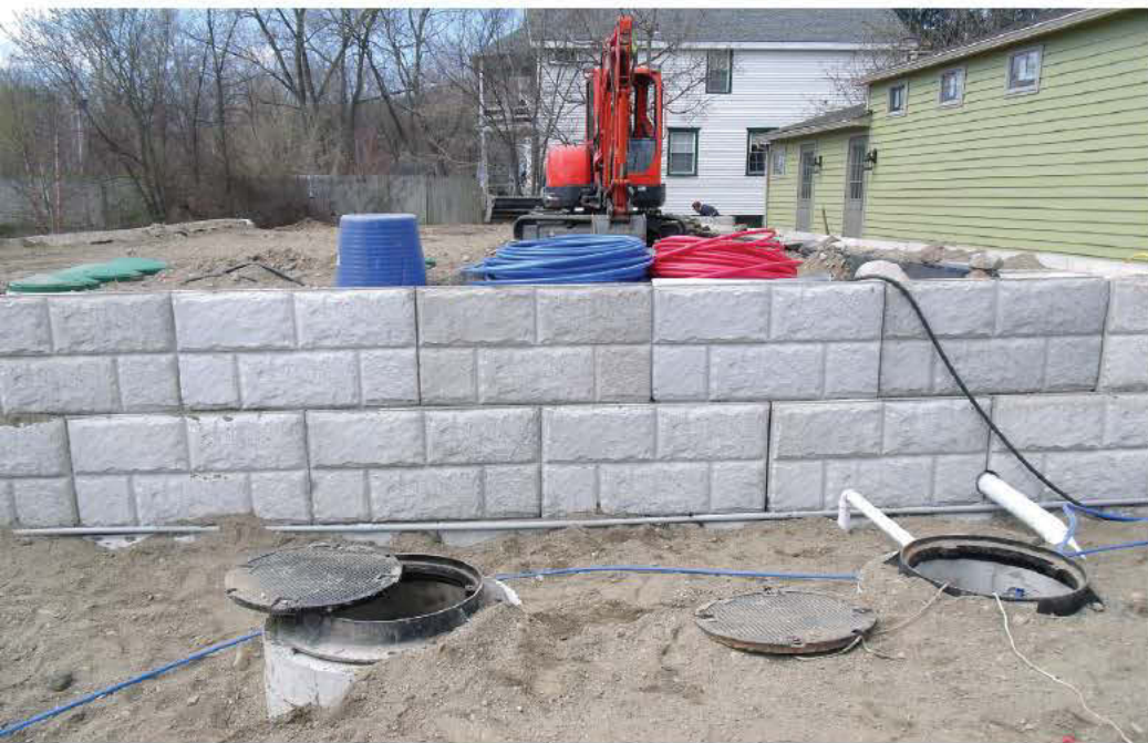
LEFT: A 6-inch pipe sleeve penetrates the head of the retaining wall. It houses the recirculation line from the first distribution box to the septic tank. Beyond the wall are three Fusion purification units and the drainfield. The grease interceptors are between the building and right leg of the enclosure. ABOVE: The clay berm at the foot of the drainfield enclosure is 10 feet from a protected trout stream defining the west boundary of the property.
