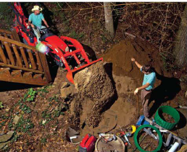
Heath Kilgore (left) and Justin Kilgore fill in with sand around a new Liberty Retro grinding station in Blue Ridge, Ga.
