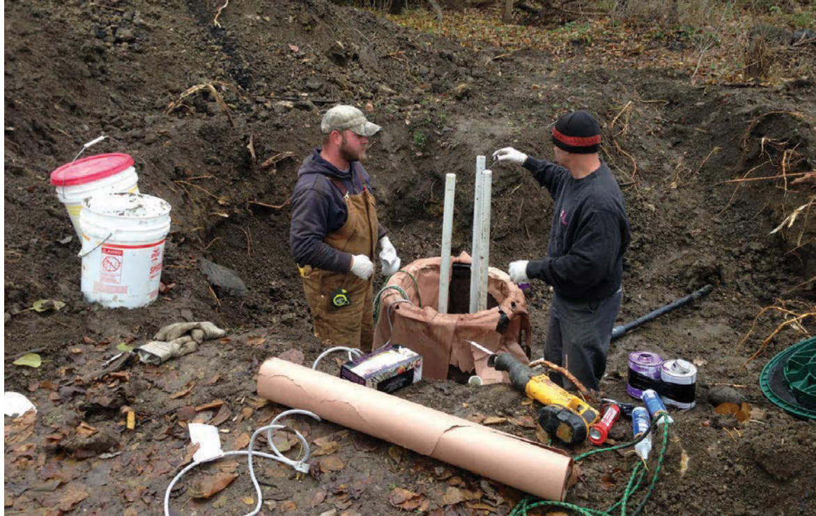
Ben Hoffman (left) and Jim Koltun-chik convert the 3,000-gallon holding tank at one campsite to a dose tank.
