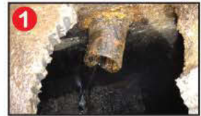
Before (Cast Iron Pipe)
