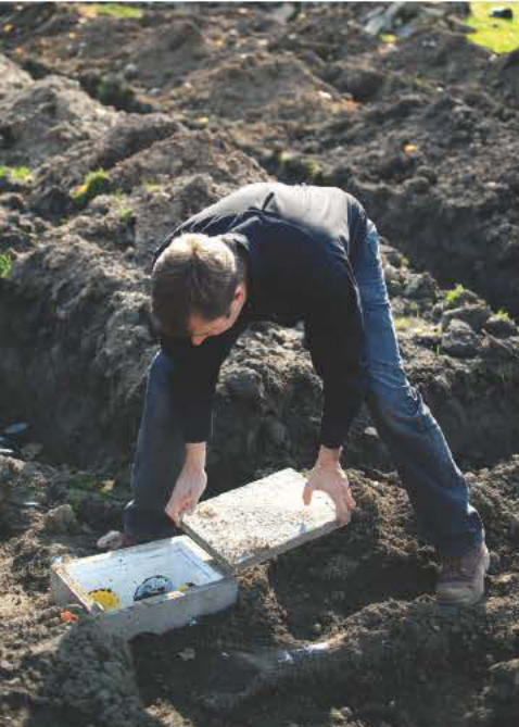
ABOVE: Murdock inspects a distribution box made by Sunnycrest Precast in Auburn, N.Y., at a newly installed onsite system. RIGHT: Craig Hurd from Finger Lakes Recycling (left) and Murdock review a letter from a local health department approving a system design.
