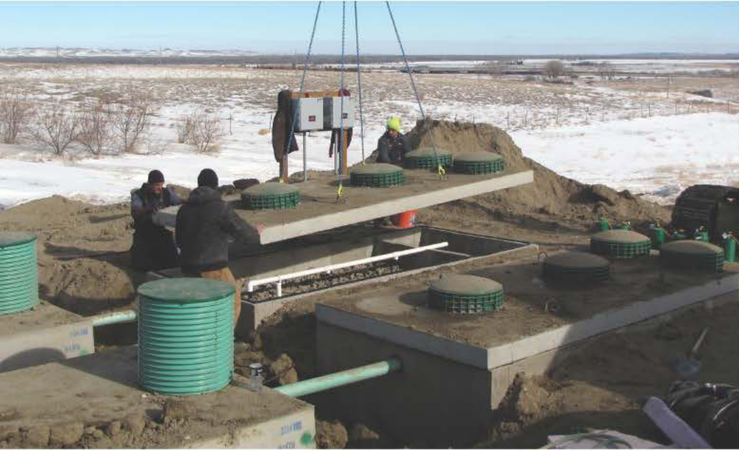
LEFT: Justin Buchanan guides the lid onto an Eliminite fixed-film bioreactor. RIGHT: Buchanan wires a control panel from SJE-Rhombus.
