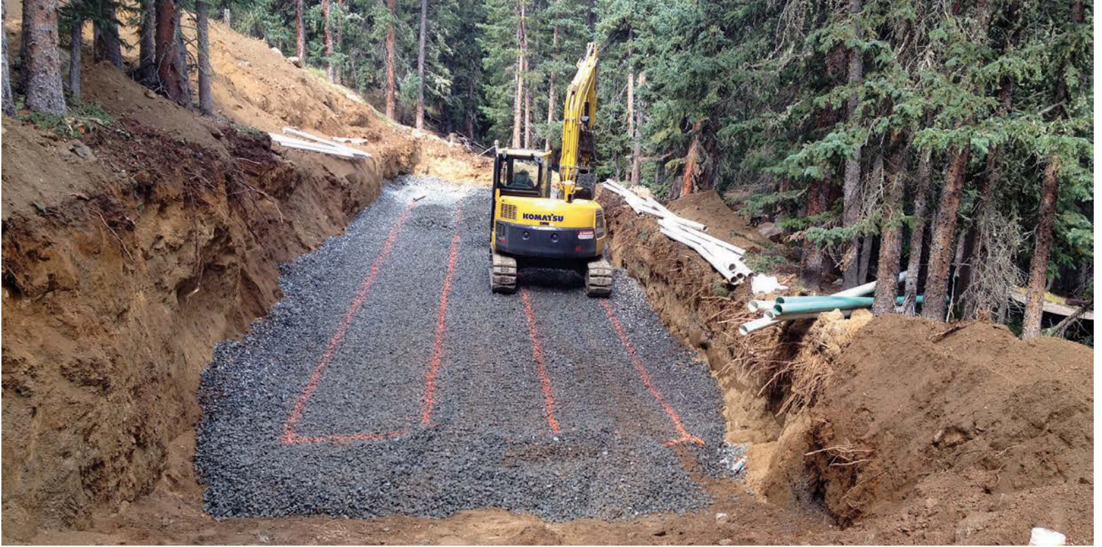
ABOVE: The 21- by 100-foot-long drainfield lies next to, but down gradient, from the old bed. The mountainside has a 20 percent slope. BELOW: Located 30 feet away, the blower introduces air into the treatment tank at 90 to 140 cfm.
