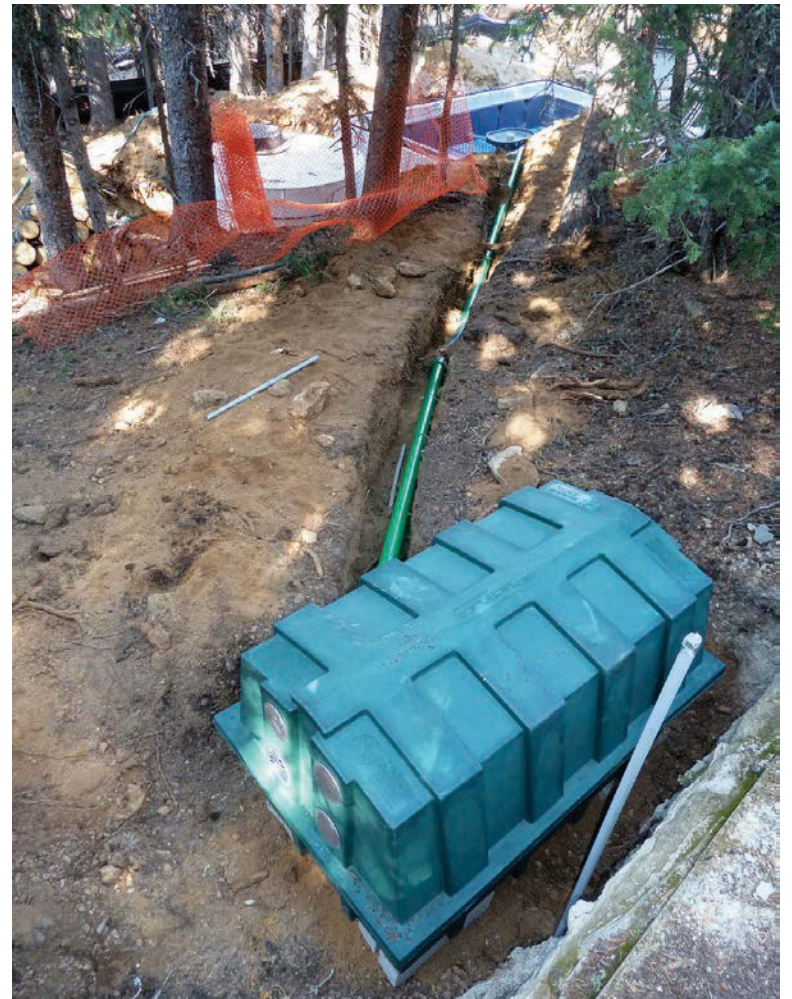
ABOVE: The 21- by 100-foot-long drainfield lies next to, but down gradient, from the old bed. The mountainside has a 20 percent slope. BELOW: Located 30 feet away, the blower introduces air into the treatment tank at 90 to 140 cfm.
