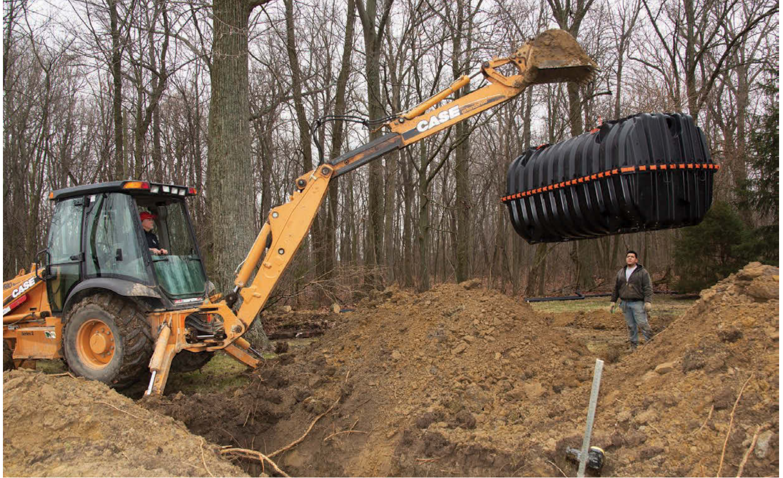
ABOVE: Baker lifts a 1,000-gallon Infiltrator Systems dosing tank during an install as Alberto Mendoza looks on. RIGHT: William Horgus sets up the Leica Rugby Pro 100 laser level to take a reading during a system install.
