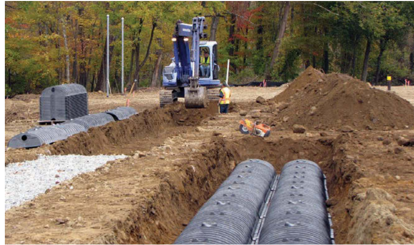
LEFT: The pump tank is wrapped in urethane sheets and inlets and outlets are sealed with waterproofing grout. The dewatering pumps are still active. (Courtesy of Mark Green) BELOW: James Harrison uses a Komatsu excavator to dig a 72-inch-wide trench, while field supervisor Wayne Green checks the elevation with a laser rod. They often had to over-excavate the trench to remove cobble.
