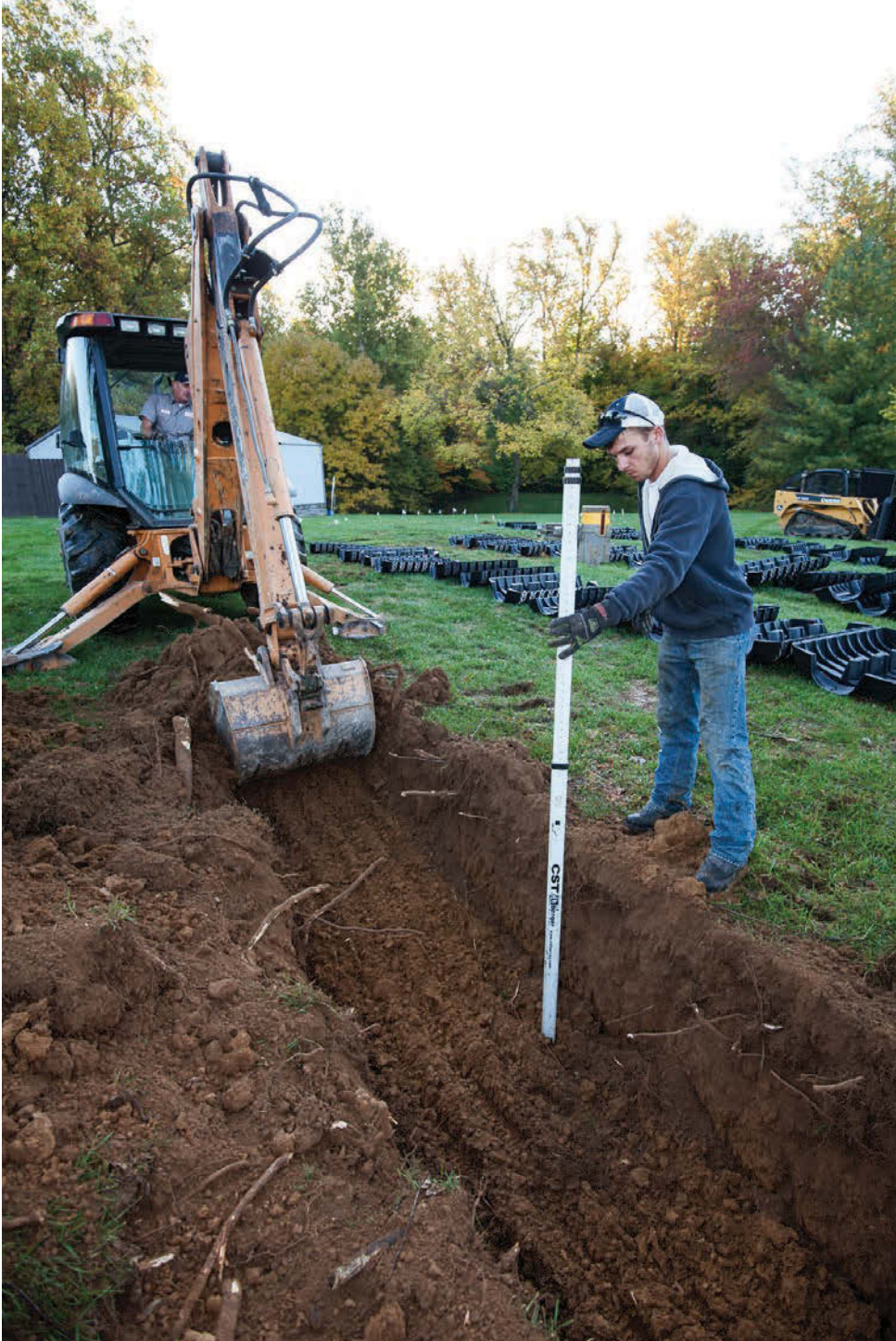
LEFT: Owner Mark Hacker uses a backhoe to dig a field bed, while Joey Ray surveys the height of the bed. ABOVE: Jordan Woning, left, and Joel Ray organize the distribution chamber system from Infiltrator Systems prior to installation.
