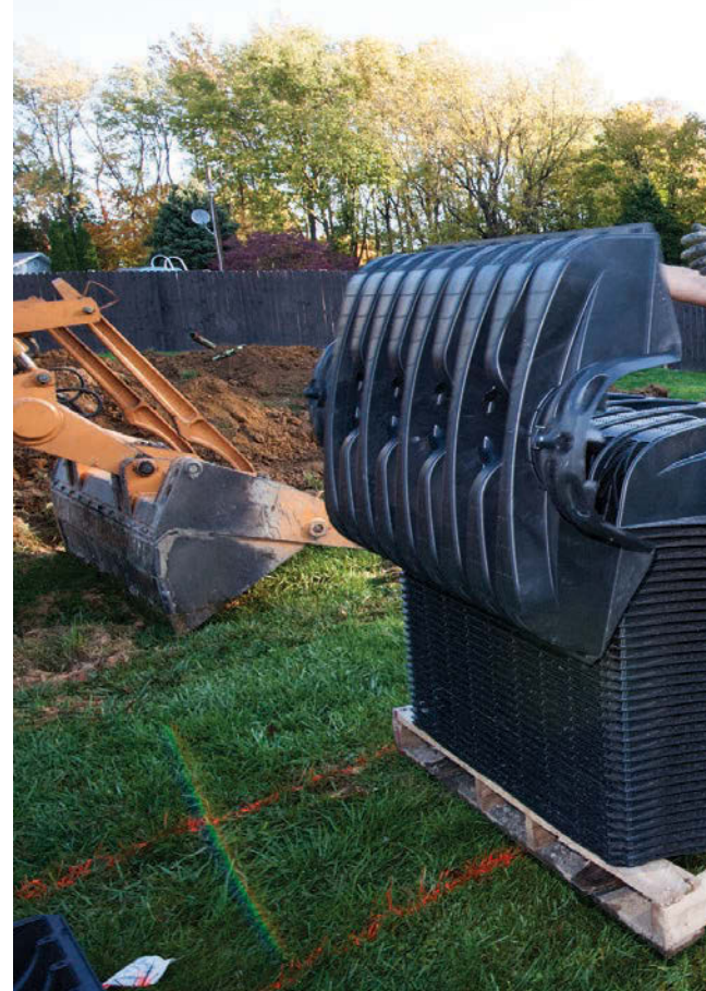
LEFT: Owner Mark Hacker uses a backhoe to dig a field bed, while Joey Ray surveys the height of the bed. ABOVE: Jordan Woning, left, and Joel Ray organize the distribution chamber system from Infiltrator Systems prior to installation.
