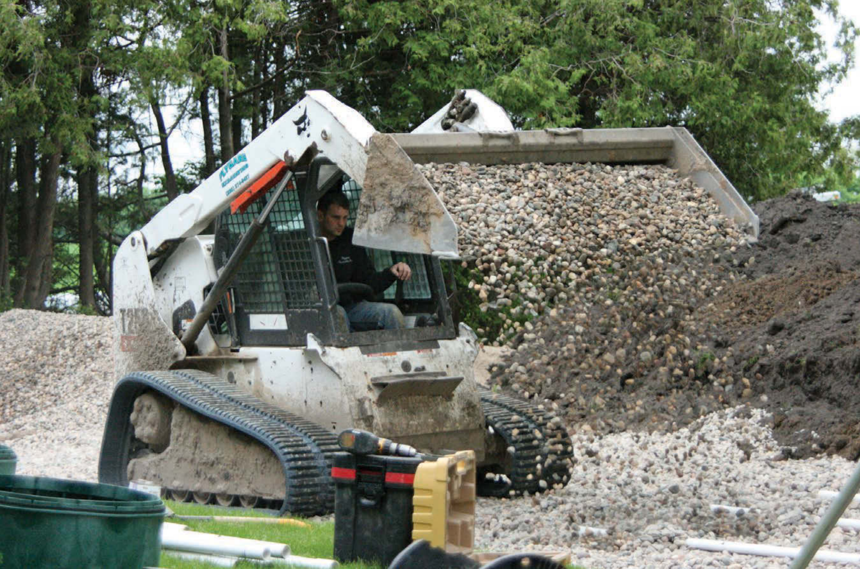
Darren Flygare installs rock in a drainfield using a Bobcat skid-steer loader.
