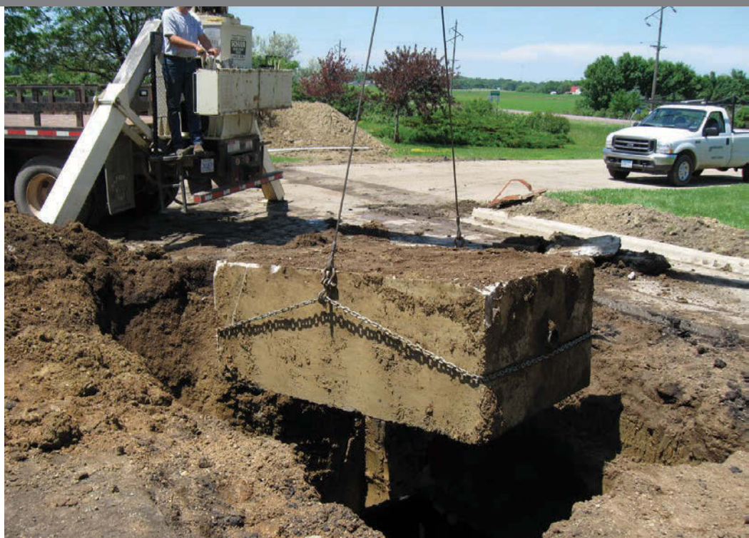
In this case of an abandoned septic system, the contractor chose to remove the old tank. (Photos courtesy of Jim Anderson)
