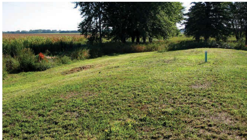
ABOVE: This mound system was just completed and needs proper ground cover. BELOW: A mound with a grass cover established.
