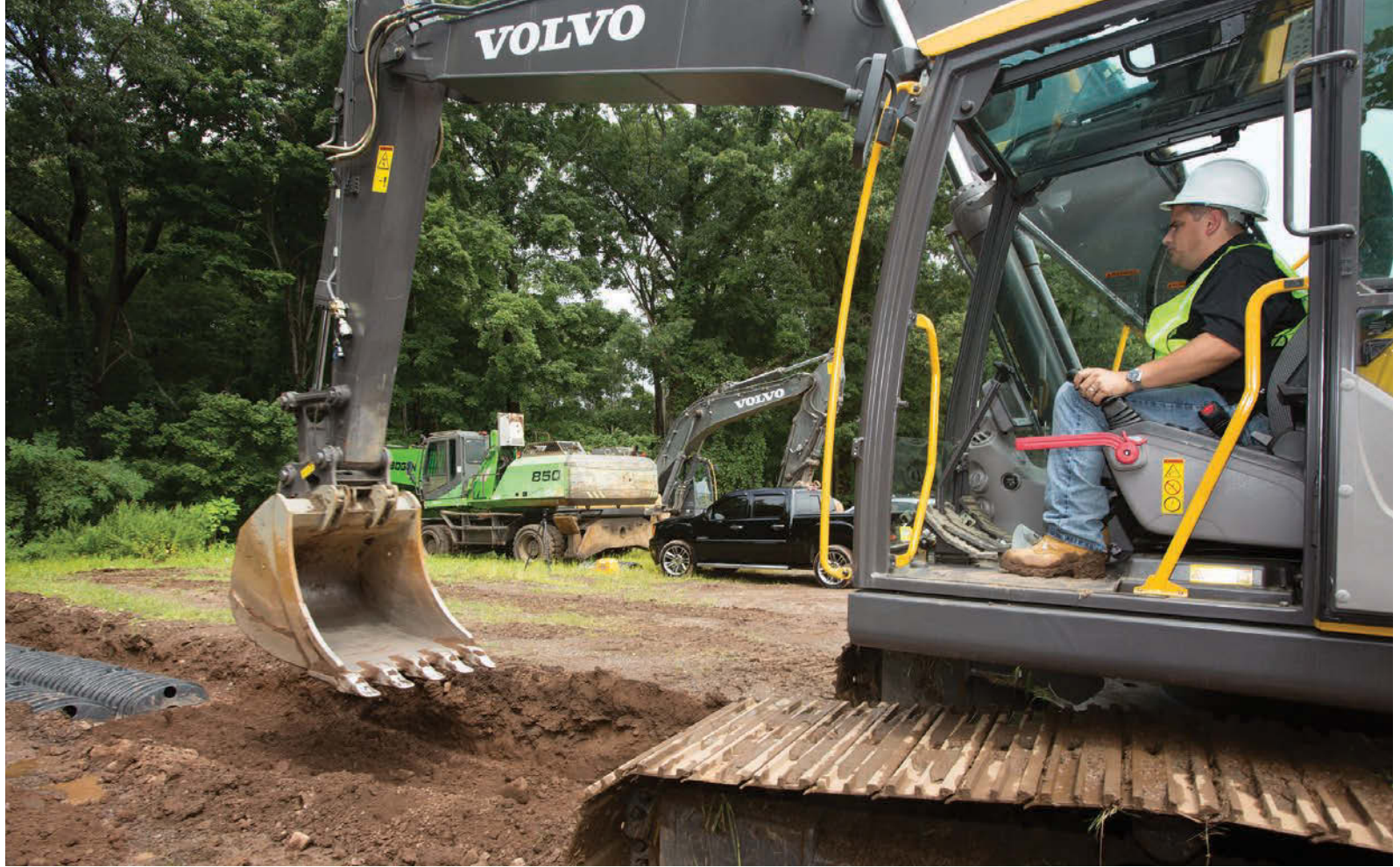
Mark Green is at the controls of his workhorse Volvo excavator installing a new drainfield.
