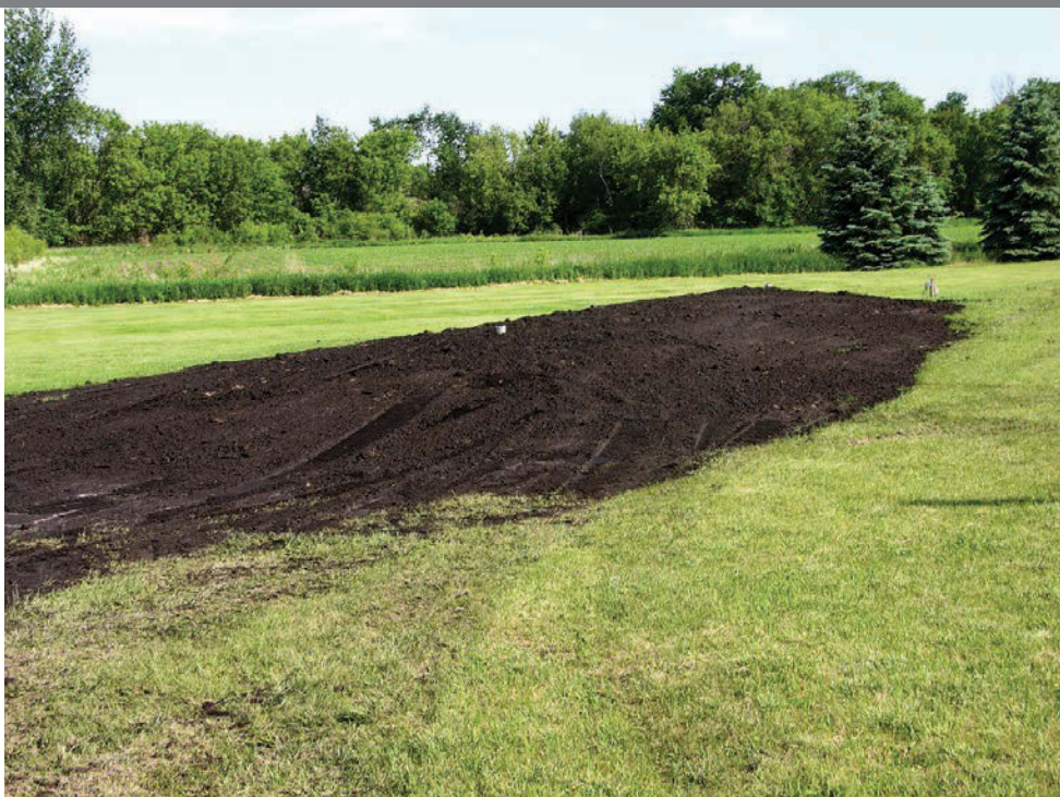
ABOVE: This mound system was just completed and needs proper ground cover. BELOW: A mound with a grass cover established.
