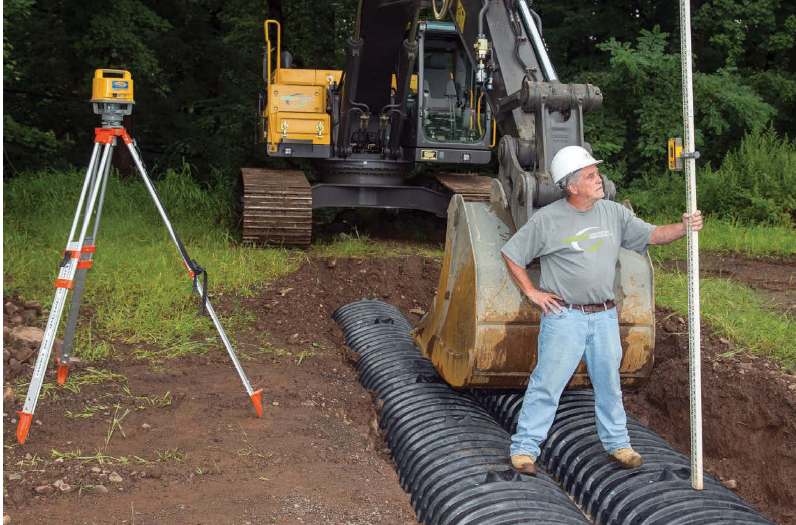
ABOVE: Wayne Green uses a Spectrum LL500 laser/target (Spectra Precision) to confirm the proper height of a double row of CULTEC Contactor 100 chambers at a work site. BELOW: Mark Green's young company serves customers in a 50-mile radius around Waterbury, Conn. Here he poses on a work site with his Volvo 250 excavator in the background.
