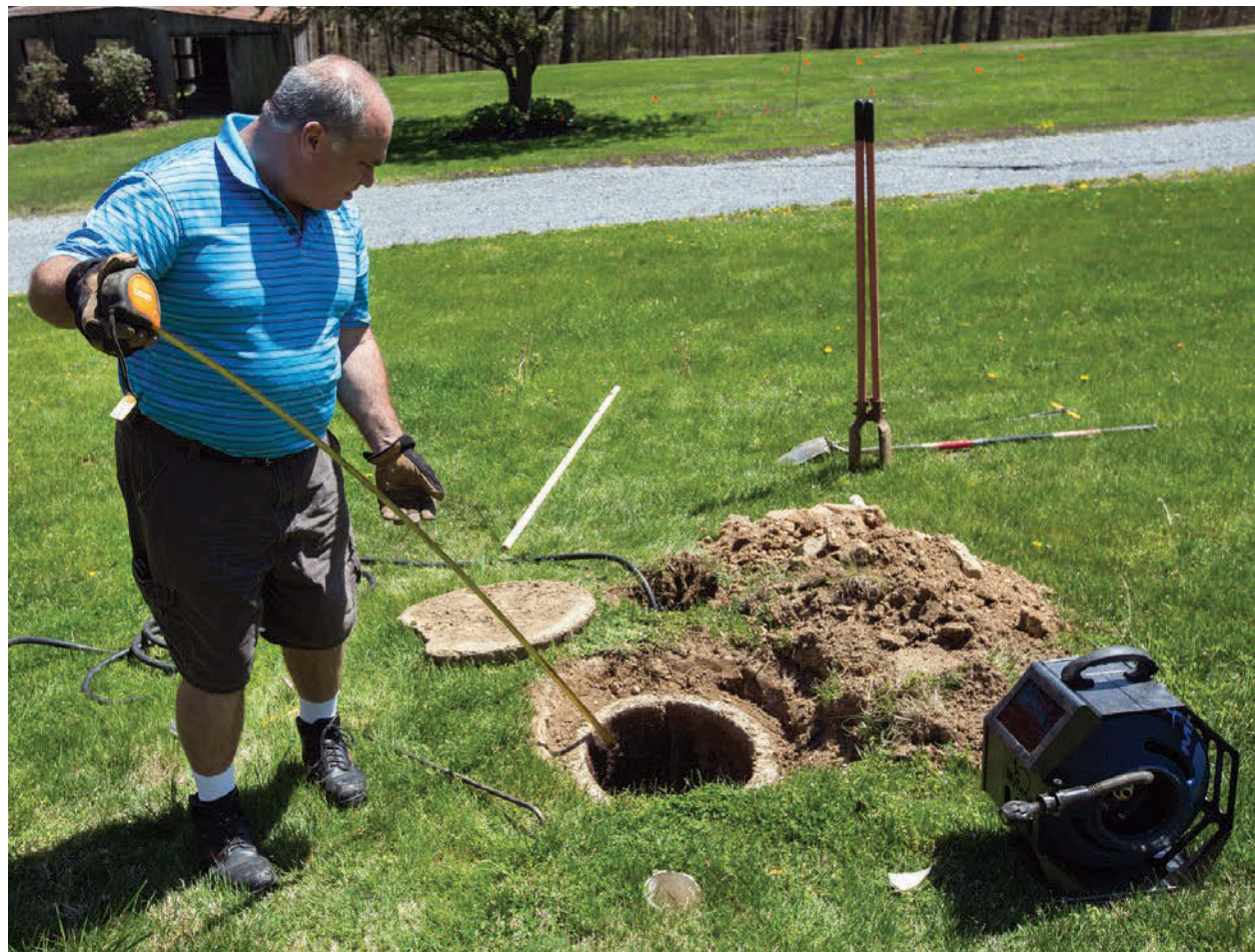
Parker measures the depth of a septic tank during an inspection in Coatesville, Pa.
