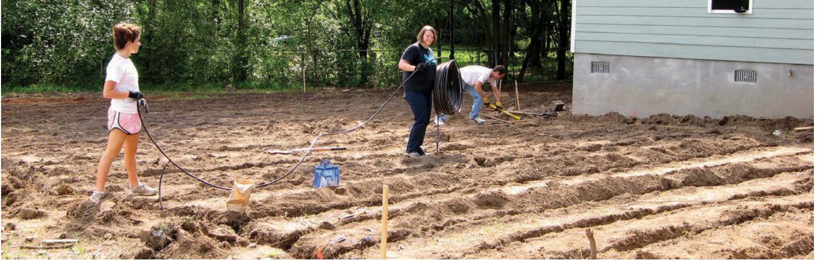
ABOVE: For the first Mercer University project, drip trenches were dug first and not filled until the connections and every other aspect worked. This system was the senior design project for Kristina Deer, center. Sarah Dorminy, left, helps lay tubing, while Micah Esmond works in the background.
